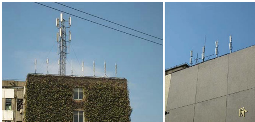
Fig. 1.11 Group cell trial systems (multi-antenna units)
