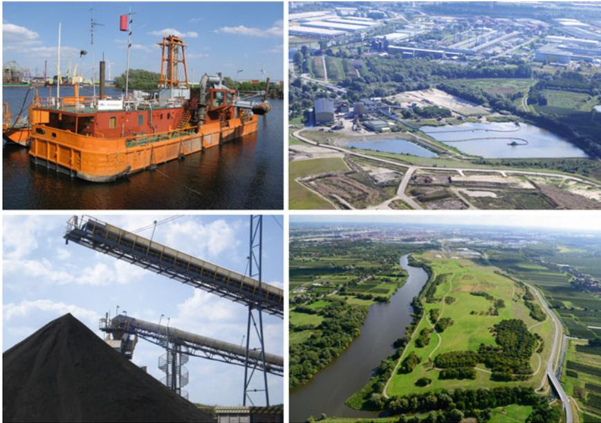
**Fig. 4** Sediment treatment in the City of Hamburg. *Upper section left* reclamation dredger, *right* the 'METHA' plant (MEchanical Treatment of HARbour sediments). *Lower section left* stockpiling of dewatered separated contaminated sediment, *right* silt disposal site Francop/Hamburg. *Sources* Hamburg Ministry of Urban Development and Environment and Hamburg Port Authority
