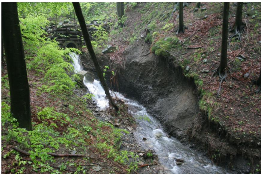
**Fig. 4** Accelerated incision downstream the sluice during 5/2010 flood event (Lubina watershed)
