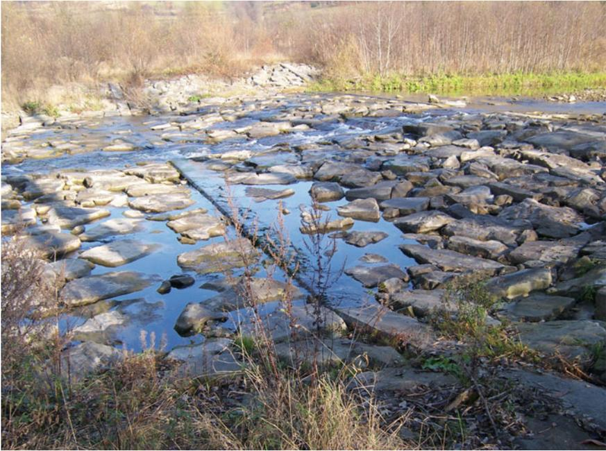
**Fig. 1** Rapid hydraulic structure (RHS) in Porębianka stream under low water level conditions in summer 2011 (*photo* by K. Plesiński)
