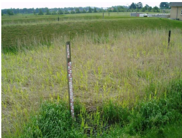
Figure 19.5 Basin containing Nickel polluted sludge. Note the yellow color and poor reed coverage (06-06-2011) (Photo: Orbicon).
