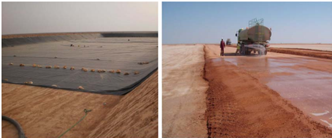
Figure 1.3 Installation of the HDPE liner in the buffer pond (left) and of the mineral sealing layer in the wetland cells (right).
