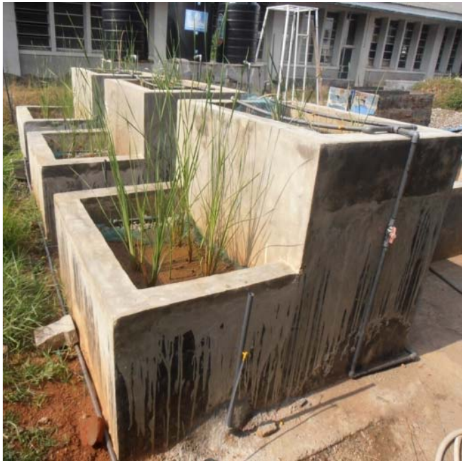
Figure 13.3 Plate 1: Pilot scale hybrid constructed wetland units planted with Typha angustifolia .
