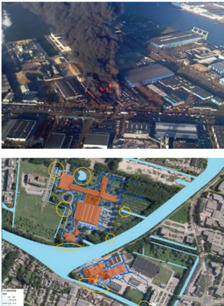
Figure 23.12 Top: fire at Moerdijk (the Netherlands) leading to environmental disaster. Bottom: surface model at industrial site to calculate the outflow of water during intensive rainfall or emission during calamities to locate the best locations for constructed wetlands.
