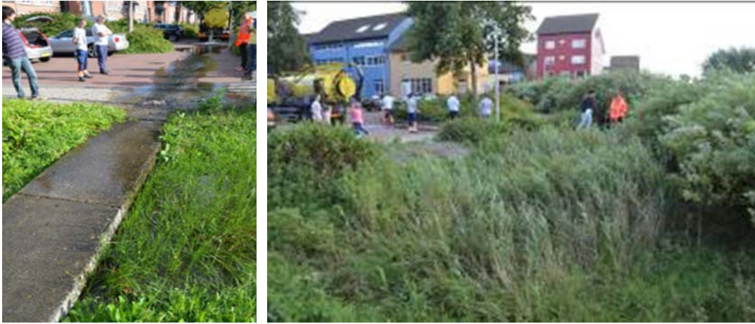
Figure 23.13 Full-scale testing of horizontal constructed wetland in Purmerend [2]. Reproduced with permission.
