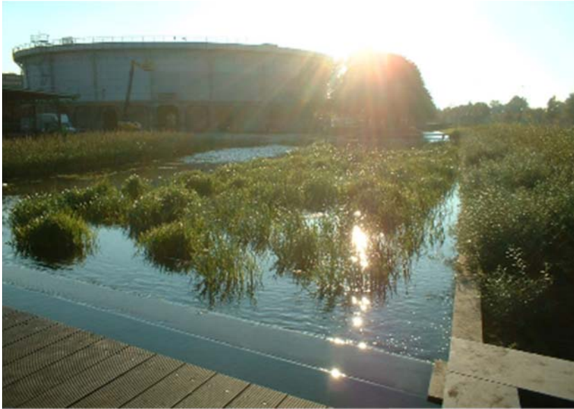
Figure 23.7 Example of horizontal wetland in Amsterdam in Westergasfabriekpark for closed system [11].
