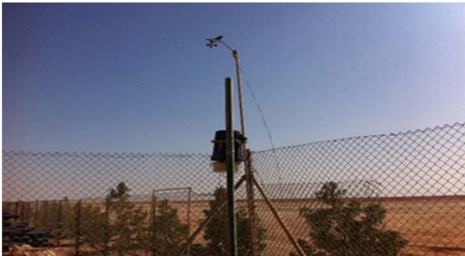
Figure 1.5 Weather station close to the SFCW cells. [5]
