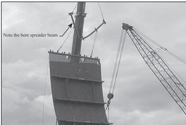
Fig. 9–3 Bent spreader beam.
