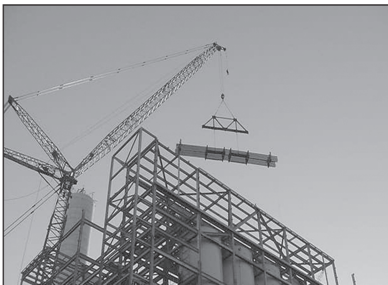
Fig. 6–1 A safely planned lift—there are no personnel below the load.
