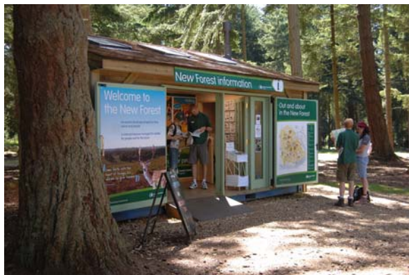
Plate 48 Mobile steel visitor centre, New Forest, UK (Worthington) see box 81
