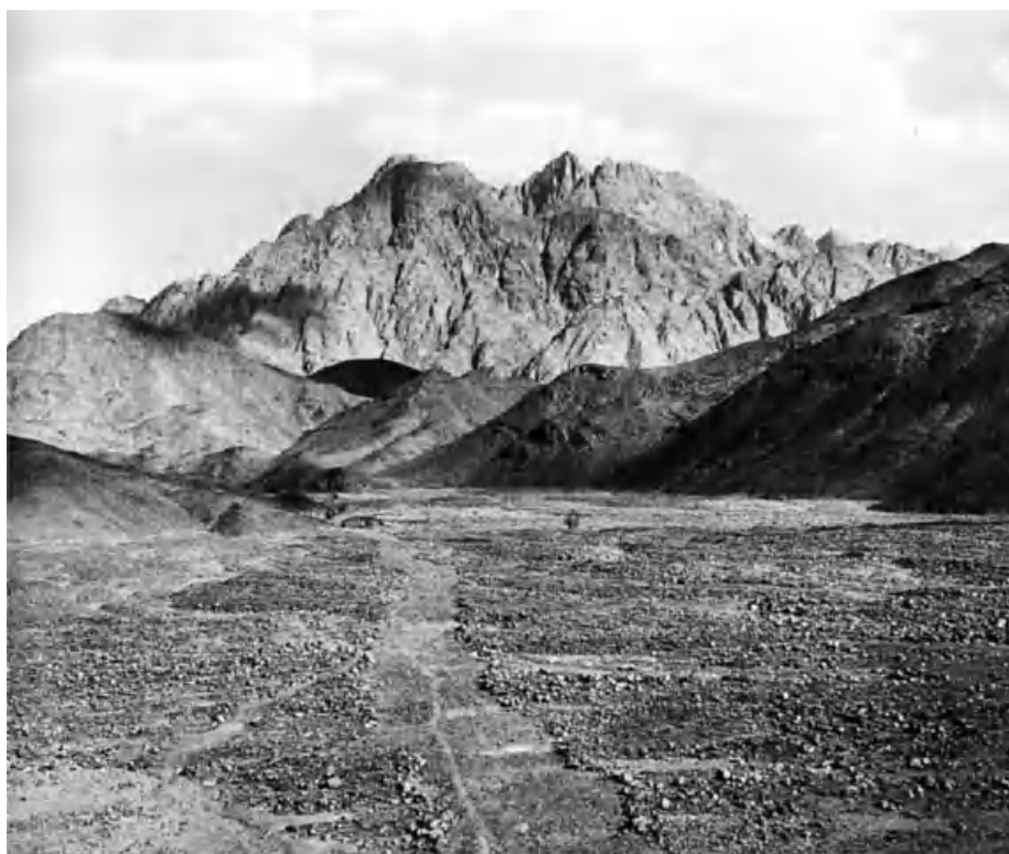
Figure 12.1b Unpaved road in Egypt's eastern desert: a gravel surface cleared of boulders for a width of approximately 8 m.
