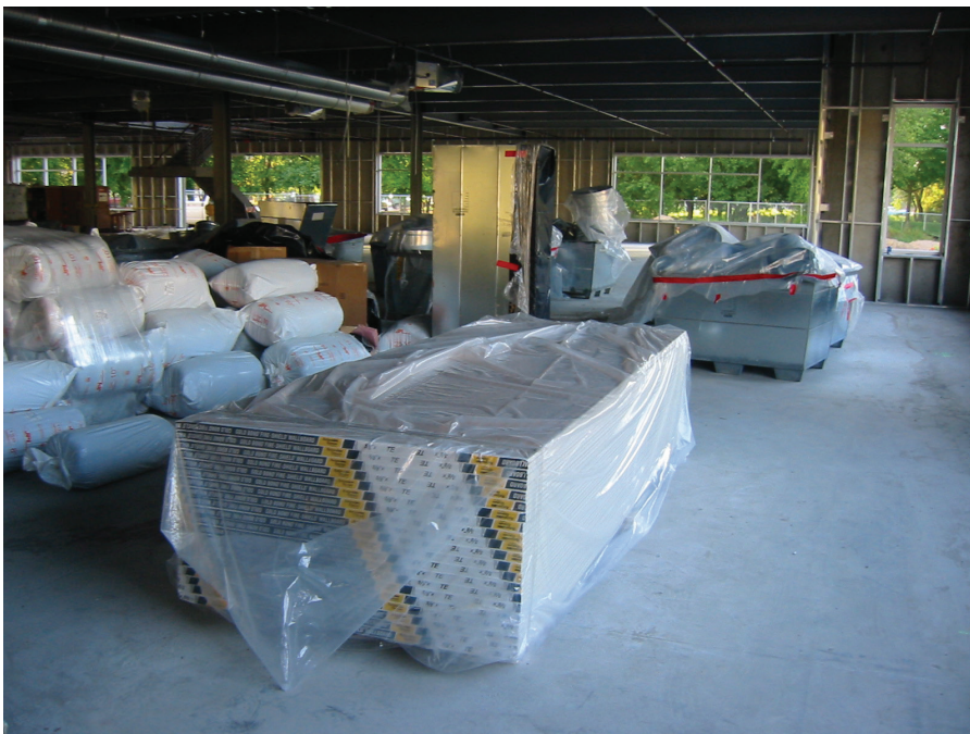
Figure 14.6 Construction products and materials such as the gypsum board shown here should be kept dry, covered, and off the ground to prevent future mold and IAQ problems. (Photograph courtesy of DPR Construction, Inc.)
