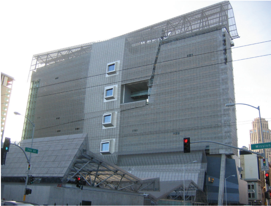
Figure 16.2 The folded, perforated metal skin covering portions of the San Francisco Federal Building assists in the flow of air through the structure and provides an interesting and appealing appearance for the structure, both at the ground level and at the upper façade. (Photograph courtesy of Jenna Hildebrand)
