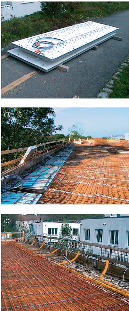
Figure 2.29 (A) The edge strip heating elements placed in the formwork. (B) Technical installation in the reinforced concrete floor prior to pouring. (C) Heating, cooling, and ventilation pipes are integrated into the reinforcement. (Source: © Dietmar Straub, Besigheim, Germany, and © Martin Duckek, Ulm, Germany)
