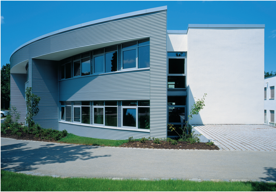
Figure 2.26 The signature exterior of OWP 11 in Stuttgart, Germany, is its metal façade, which is the outer layer of a well-insulated wall system that reduces internal heating and cooling loads to very low levels. (Source: © Dietmar Straub, Besigheim, Germany, and © Martin Duckek, Ulm, Germany)
