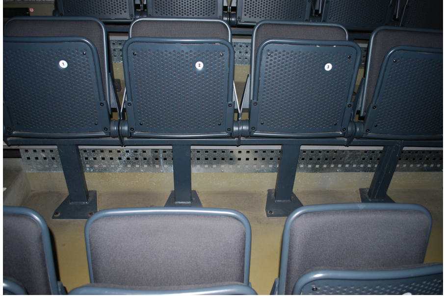
Figure 7.11 Grilles located under the seats in the performance halls are the locations where air flows into the spaces for heating, ventilating, and cooling. The main mode of operation is natural ventilation, with airflow being induced by the buoyancy or rising warm air in the exhaust air chimney.
