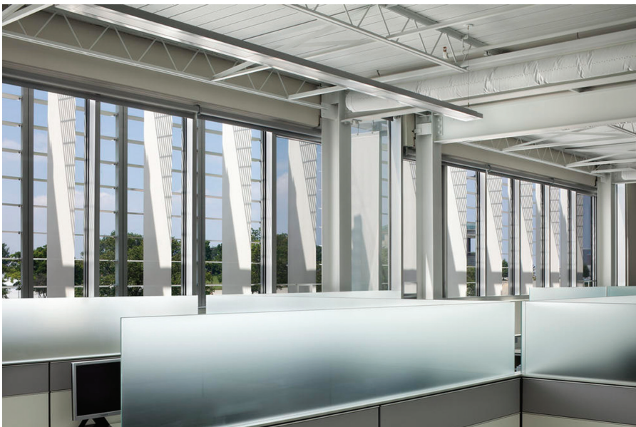
Figure 8.14 The daylight harvesting system functions at such a high level that it allows lights to be shut off during 98 percent of daytime hours. The operable windows provide local thermal comfort control and are also part of a cross-ventilation scheme activated by the building automation system, which emails occupants when conditions are suitable for opening windows. (Copyright Assassi, Courtesy of BNIM)
