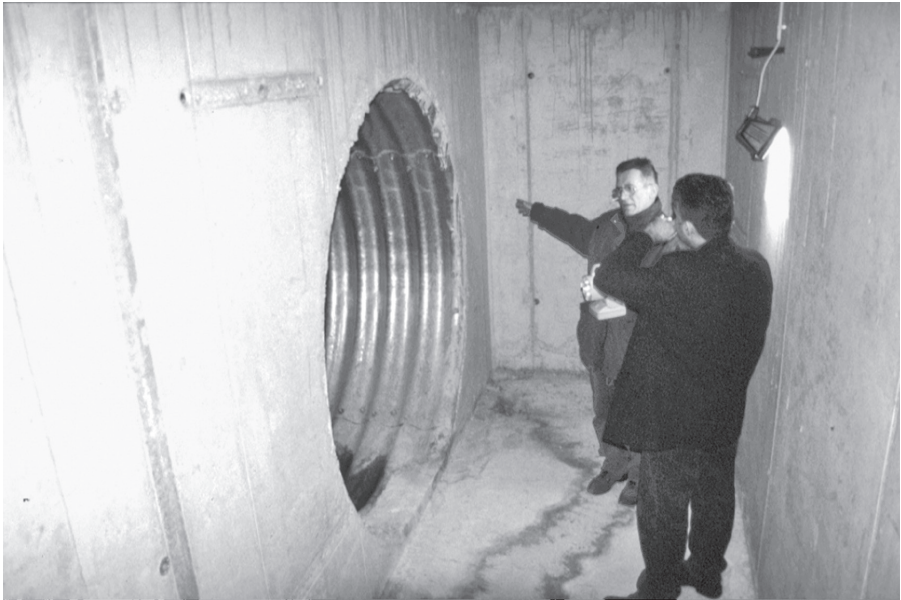
Figure 9.24 Ground-coupled system showing an air intake tube, 1.8 meters (6 ft) in diameter, under a Mercedes showroom in Stuttgart, Germany. The galvanized steel tube, which is 100 meters (325 ft) long, heats cold air via ground contact in winter and cools hot air in summer. The tube is located in a zone under the building where the temperature is a constant 16°C (60°F).
