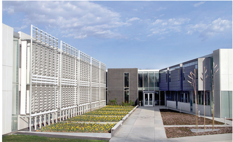
Figure 8.15 The louvers on the south façade of the IUB/OCA Building contribute to the passive design of the facility by controlling solar glare and heat gain while admitting daylight. (Photo courtesy of iub.iowa.gov)
