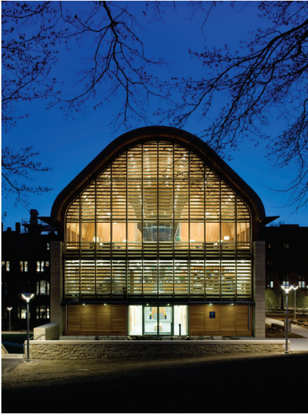
Figure 3.31 (D) The south side of the building is recessed, and window overhangs are integrated into the building façade to control glare and thermal loads while maximizing daylighting. (Photograph by Morley Von Sternberg)
