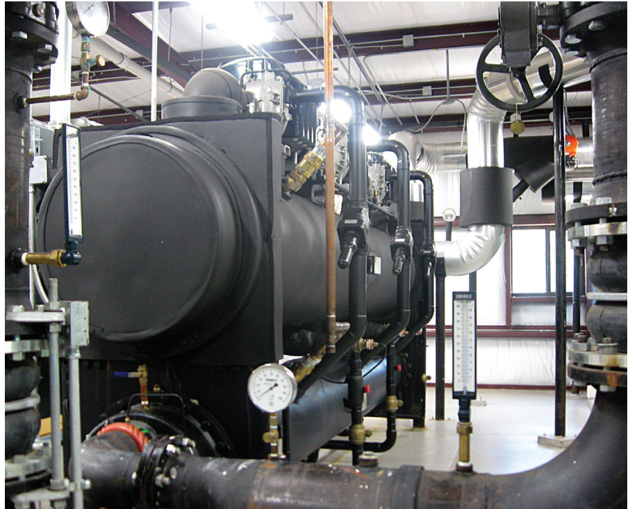
Figure 6.8 A high-efficiency Smardt centrifugal chiller was installed to replace the outdated unit, providing cooling for the entire St. Johns River State College. The chiller is designed to meet future needs as the campus continues to expand. (Photograph courtesy of Glen Roberts, St. Johns River State College)
