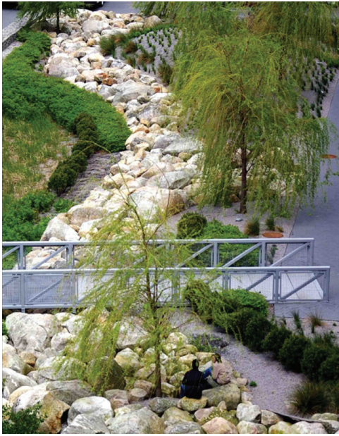
Figure 8.8 The stormwater bioretention system for the Stata Center, a Frank Gehry–designed building on the Massachusetts Institute of Technology campus in Cambridge, Massachusetts, is a multifunctional constructed wetland that detains runoff to reduce peak downstream flow. The plants and planting medium of the wetland clean the runoff and allow some groundwater infiltration. (Photo by Stuart Patton Echols)
