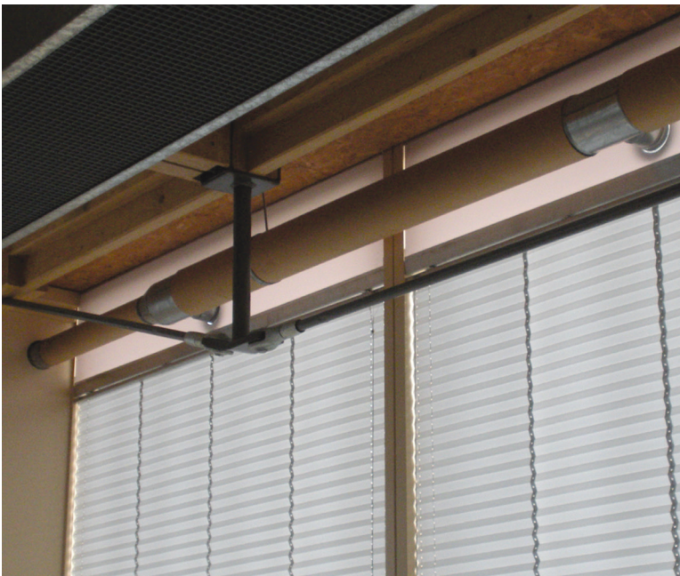
Figure 11.11 (E) Cardboard ductwork is inexpensive, resourceful, and recyclable and will be close to the end of its life expectancy by the time the XX Office Building is ready for deconstruction. (D. Stephany)
