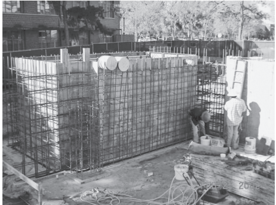
Figure 10.9 The rainwater harvesting system for Rinker Hall at the University of Florida in Gainesville has a cast-in-place cistern (shown here under construction) located under the south stairwell of the building. The rainwater is used for flushing the building's toilets. (Photograph courtesy of Centex-Rooney, Inc.)
