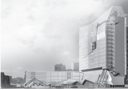
Figure 3.1 The Federal Building in San Francisco, California, exemplifies ecological design by employing local natural forces, such as the prevailing winds and sunlight, to provide cooling and daylighting. Detailed analysis of natural airflows induced by wind and thermal processes was accomplished using sophisticated computational fluid dynamics modeling. (Illustration courtesy of Morphosis Architects)
