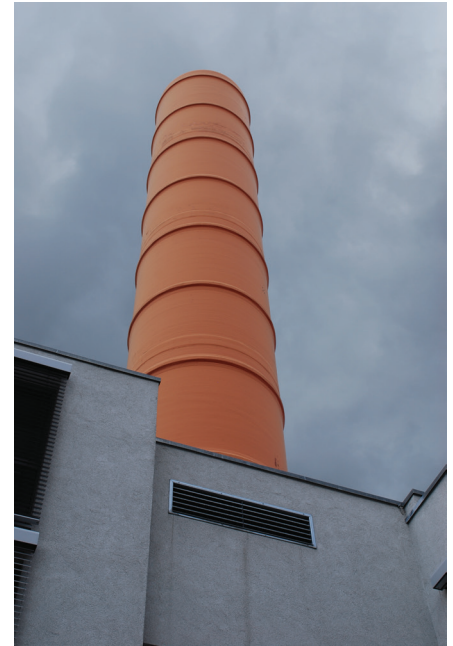
Figure 7.8 The key element of the Theaterhaus natural ventilation system is a 93-foot (30-m) chimney, which induces airflow from outside the building, through the building interior space, to be exhausted by the stack, or chimney, effect. The chimney was a feature that was added to the building and that adds to the industrial appeal and appearance of the former steelworks.
