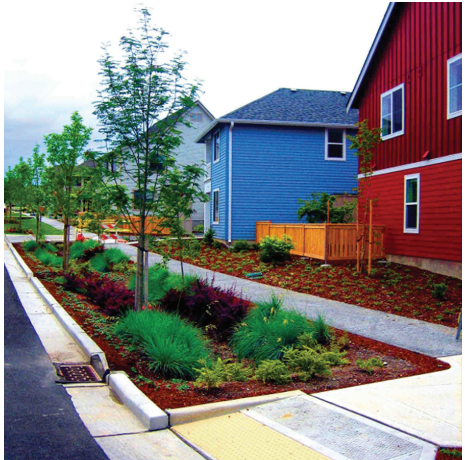
Figure 8.7 Designed in partnership with the Housing Authority of Seattle, Washington, this natural drainage system for the High Point neighborhood of West Seattle treats about 10 percent of the watershed feeding Longfellow Creek—one of Seattle’s priority watersheds. The natural drainage system mimics nature in many ways by using features such as swales to capture and naturally filter stormwater and open, landscaped ponds or small wetland ponds to hold an overflow of stormwater. (Photo by Stuart Patton Echols)
