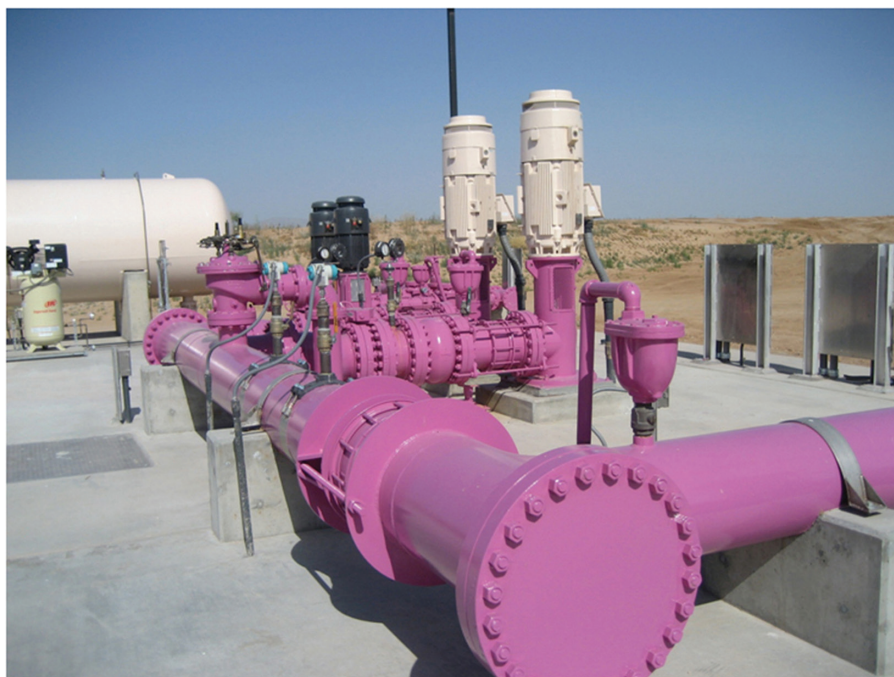
Figure 10.13 (A) Reclaimed water is former wastewater that is cleaned and redistributed through a clearly coded system of bright purple pipes. Reclaimed water is used when the application does not require potable water. (B) Posting is mandated where the water comes in contact with the public so as to prevent human consumption. (Source: City of Clermont, Florida)
