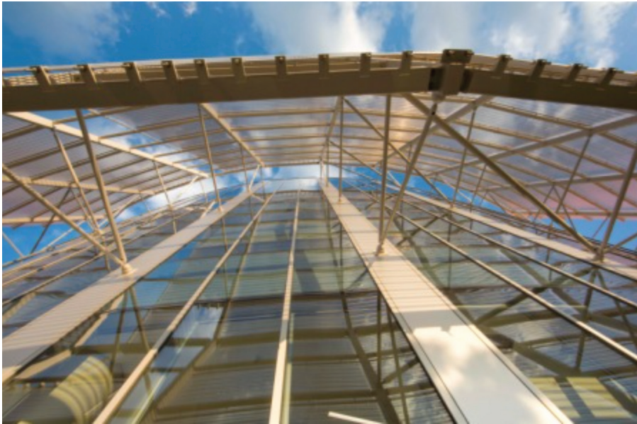
Figure 5.11 The metal mesh sunscreen is the signature architectural element of the University of Florida Research and Academic Center laboratory building. It reduces heat and glare while allowing daylighting and views through the often very challenging west façade of the building. (Photo courtesy of HOK Architects)
