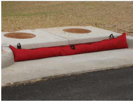
Figure 14.1 Storm drain inlet protection implementation on a newly constructed site. This type of device must be monitored continuously during construction operations to ensure it is functioning properly. (Don Thieman, CPESC, ASP Enterprises)
