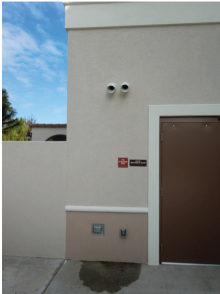
Figure 14.10 The CxA identified boiler exhaust condensation and dripping onto an exterior outlet and proposed the relocation of the electrical outlet to prevent future corrosion as well as increase safety. (Photograph courtesy of John Chyz, Cross Creek Initiative, Inc.)
