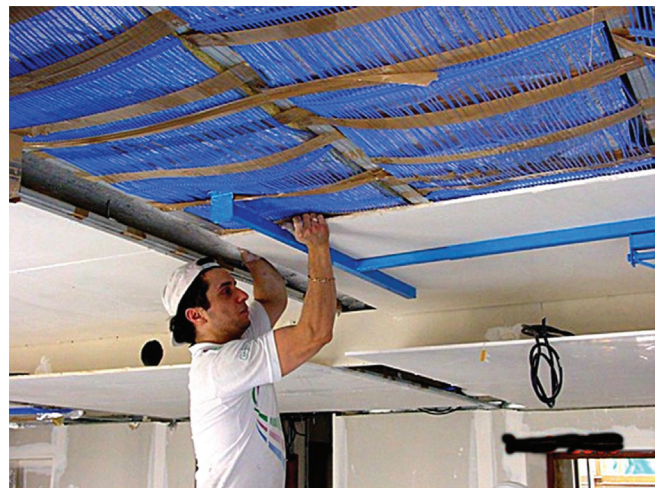
Figure 9.23 Radiant cooling panels provide a low-energy solution for cooling, requiring only a fraction of the energy of a conventional system based on air handling and ductwork. (A) A dropped-panel installation showing a radiant cooling panel installation and ease of maintenance. (B) Installing a cooling mat: grids of plastic tubing carrying chilled water are placed under the ceiling drywall. (Photographs courtesy of Juan Rudek, Karo Systems)
