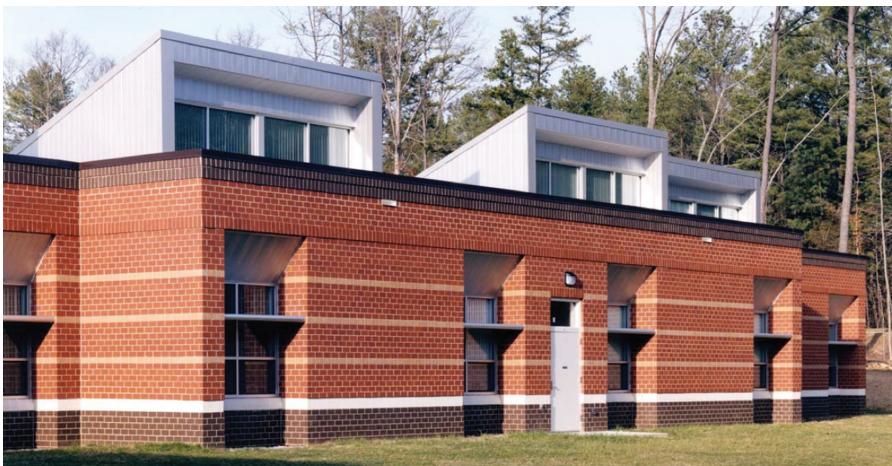
Figure 9.6 The daylighting strategy for Smith Middle School in Chapel Hill, North Carolina, employs (A) south-facing roof monitors with high-visible light transmission glazing and interior vertical baffles to provide for optimum controlled daylighting without glare throughout the entire classroom depth, (B) integrated lighting controls, and (C) exterior lighting shelves with high-visible light transmission glazing above to enhance daylighting and low-E glass for view windows below. (Sources: (A) Image courtesy of Lighting Research Center/Rensselaer Polytechnic Institute; (B–C) Innovative Design)
