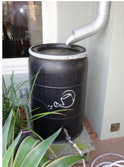
Figure 10.16 (B) Rain barrels collect roof runoff and store it for later nonpotable use. (Maxine Thomas, Florida Master Gardener/ University of Florida—IFAS Extension Realtors)
