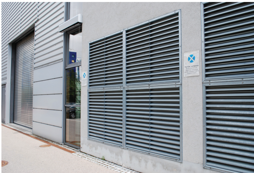
Figure 7.9 The grilles for the outside air intake for Theaterhaus are located on the side of the building. Air is induced to flow through the building by the rising warm air in the exhaust air chimney located on the top of the building.
