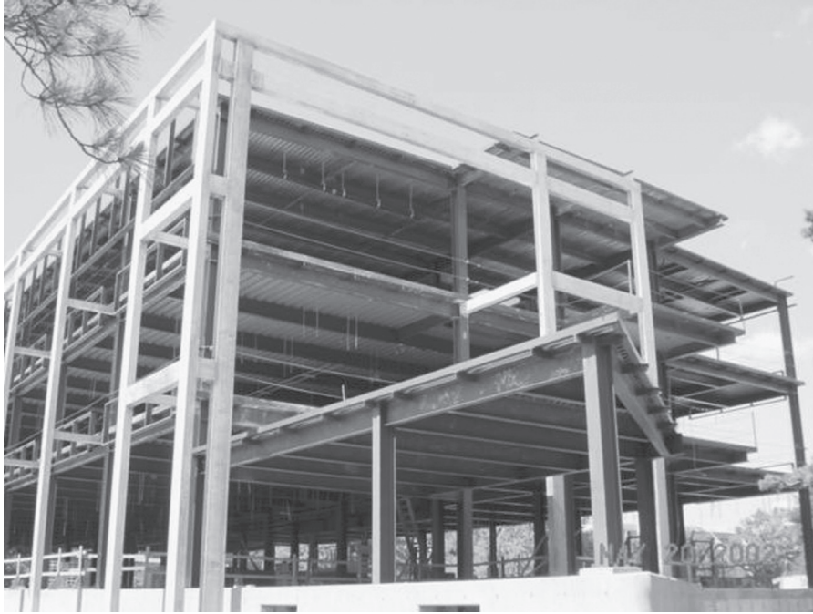
Figure 2.7 The structural system for Rinker Hall, a Leadership in Energy and Environmental Design (LEED)–certified building at the University of Florida in Gainesville, is steel. Steel is an excellent material due to its high recycled content—almost 100 percent for some building components—and is readily deconstructable and recyclable. Rinker Hall is the only building out of the thousands certified by the US Green Building Council to have been awarded an innovation credit for its deconstructability. Although some would consider metals such as steel to be “green” building materials, their embodied energy—that is, the energy required for resource extraction, manufacturing, and transport—is fairly high and results in the consumption of nonrenewable fossil fuels and the generation of global warming gases and air pollution. Consequently, whether steel can truly be considered a green building material is controversial and depends on the criteria used in the evaluation. Of all the challenges in creating high-performance green buildings, finding or creating truly environmentally friendly building materials and products is the most difficult task facing construction industry professionals.
