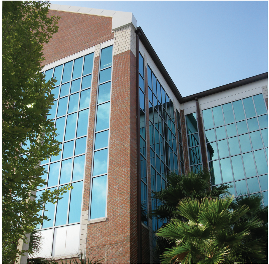
Figure 9.14 Low-E glazing on the Orthopaedics and Sports Medicine Institute at the University of Florida in Gainesville. High-technology glazing allows the design of buildings that admit visible light for daylighting but reflect infrared radiation. DOE-2.1 and daylighting simulations confirmed that daylighting and low-E glass produced greater savings than focusing solely on the thermal resistance of the building envelope. (Source: T. Wyman)
