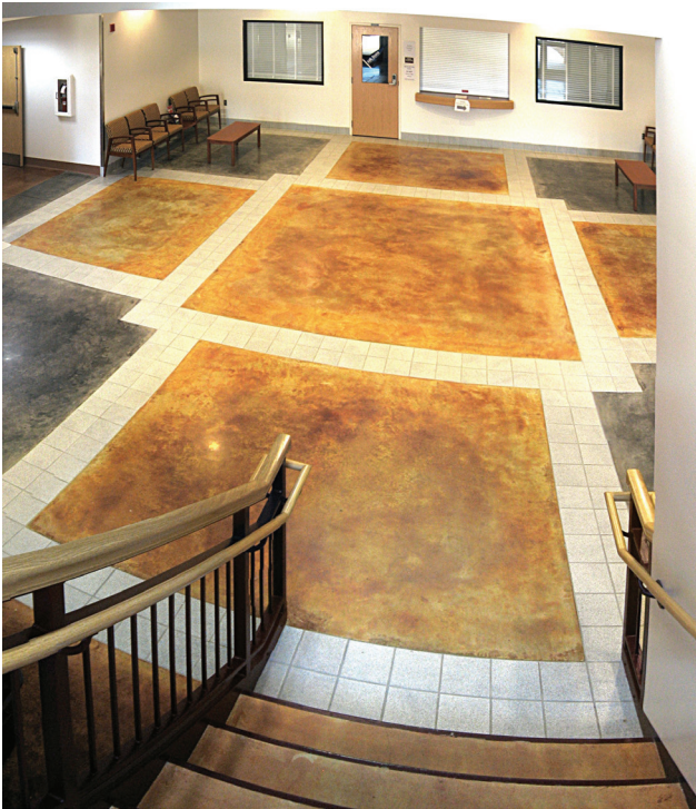
Figure 6.10 Polished, stained concrete floors were specified instead of far less durable floor coverings. These provide a long-lasting, very attractive option and reduce the quantity of materials needed for construction. (Photograph courtesy of Glen Roberts, St. Johns River State College)
