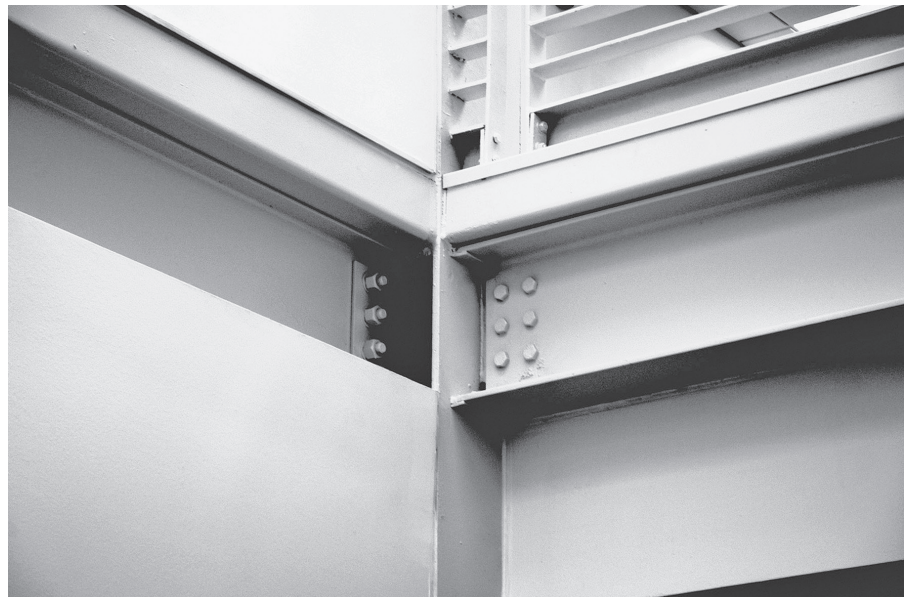
Figure 11.10 One of the innovations in the design of Rinker Hall at the University of Florida in Gainesville was to include DfD as a design criterion. One of the design features is the use of bolted, exposed steel connections to permit their ready removal. (Photograph courtesy of M. R. Moretti)
