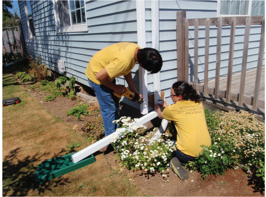
Figure 10.16 (A) Disconnecting downspouts from storm sewer systems prevents roof runoff from overloading these systems by dispersing it to vegetated areas. (Source: City of Gresham, Oregon)
