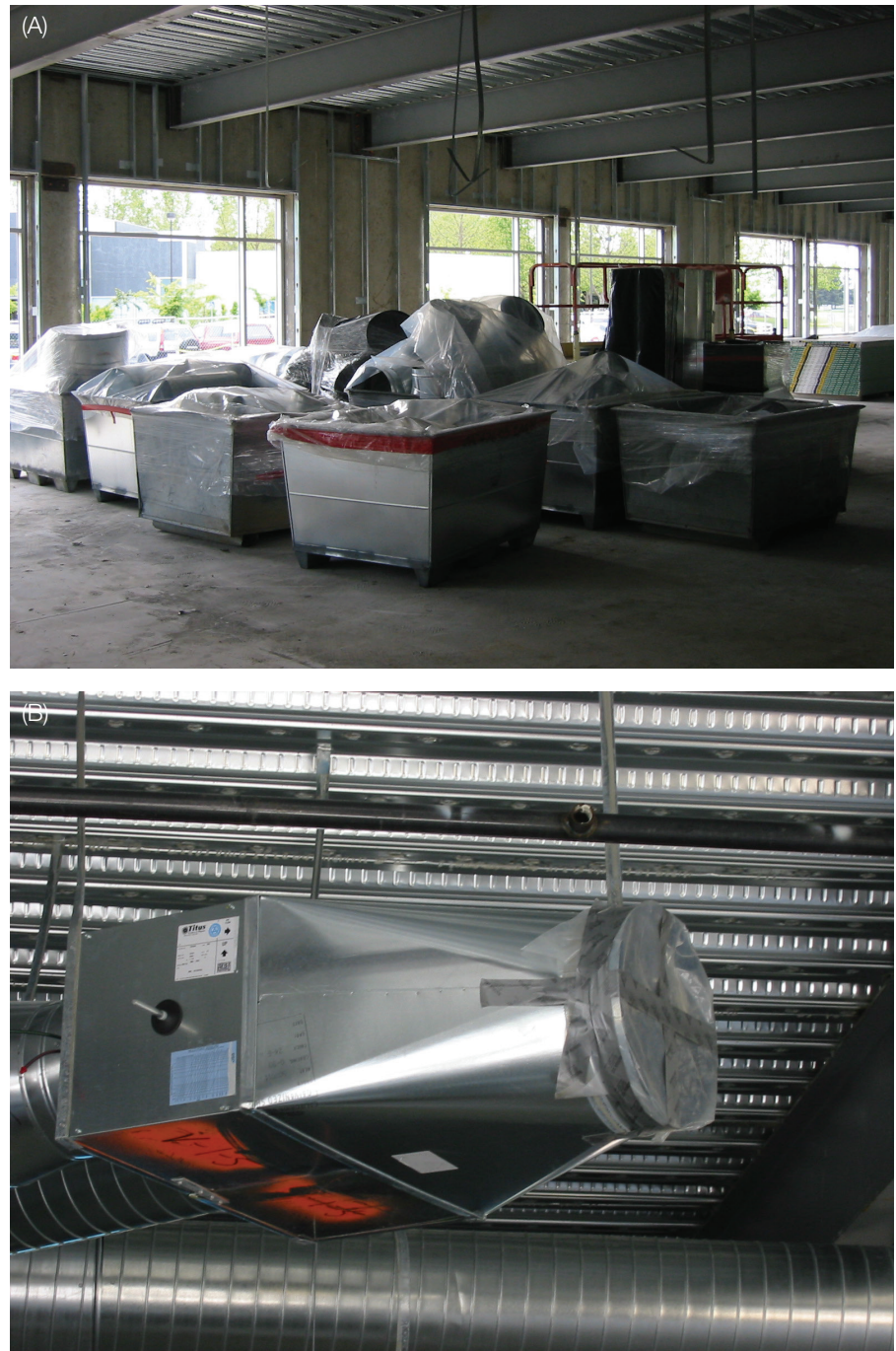
Figure 14.3 (A) Ductwork should be protected during storage and prior to installation. (B) Openings should be sealed during the installation process to prevent contamination. (Photographs courtesy of DPR Construction, Inc.)
