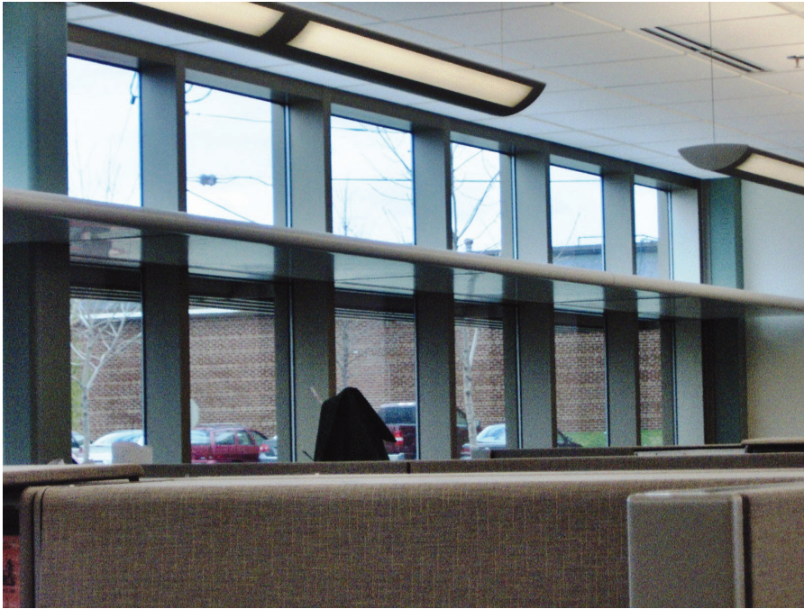
Figure 13.2 (C) A light shelf allows sunlight in while protecting users from glare that is often associated with tall windows. (Decorating with Fabric)
