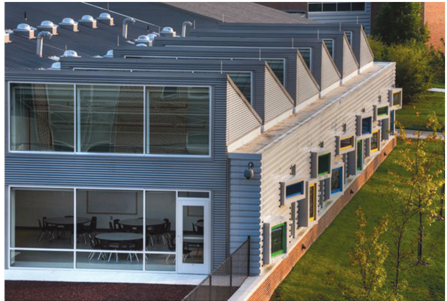
Figure 13.2 (B) A sawtooth roof design at Manassas Park Elementary School in Manassas Park, Virginia, a suburb of Washington, DC, is oriented to allow diffuse light to enter the building. This building also uses solar tubes that illuminate separate interior spaces on sunny days. (© Prakash Patel for VMDO Architects)
