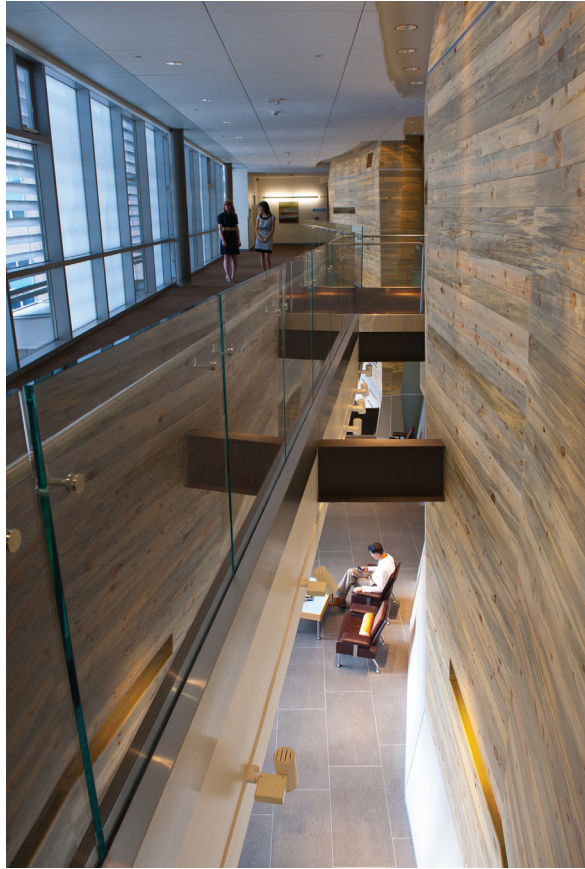
Figure 1.7 (C) The daylighting system for the NREL RSF was designed using extensive simulation. Shading devices were carefully placed on the exterior and interior to manage both direct and indirect sunlight, distributing it evenly to create a bright, pleasant working environment. (Source: National Renewable Energy Laboratory)
