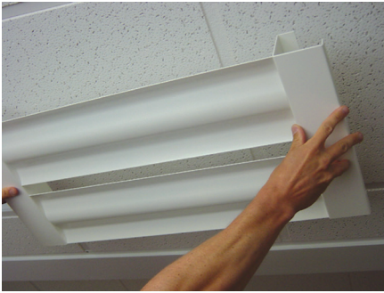
Figure 9.32 Chilled-beam systems are aluminum-finned copper assemblies through which water circulates, providing radiative cooling or heating and inducing airflow by convective effects. (Courtesy of Interface Engineering)
