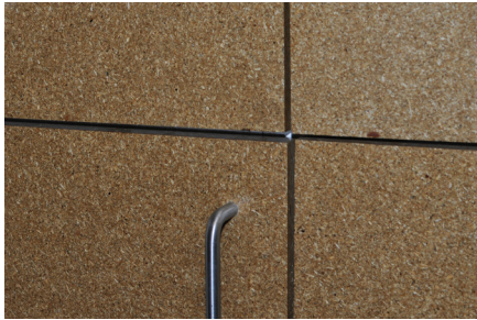
Figure 11.2 Typical of new materials emerging to serve the green building market is compressed wheatboard, made from wheat straw, which can be used in millwork or for cabinetry, as shown here in a laboratory at Rinker Hall at the University of Florida at Gainesville. (T. Wyman)
