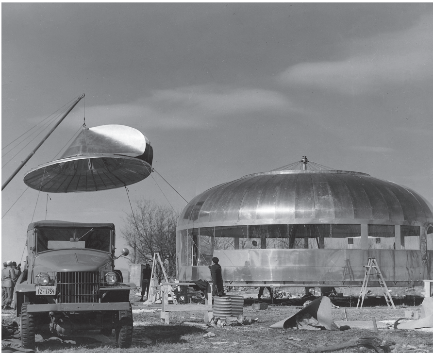
Figure 3.3 R. Buckminster Fuller's Dynamic Maximum Tension, or Dymaxion House, in Wichita, Kansas, was the first serious attempt to create an autonomous house. It was designed for mass production, weighed just 3,000 pounds (1364 kilograms) compared with the 150 tons (137 metric tons) of a typical house, featured a built-in wind turbine for generating power, and had a graywater system. (Courtesy of The Estate of R. Buckminster Fuller)
