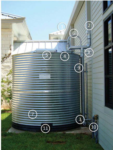
Figure 10.10 Rainwater is harvested in a cistern system consisting of these 12 components: (1) nontoxic, noncorrosive roofing material; (2) nontoxic, noncorrosive gutters and downspouts; (3) first-flush diverter with a cleanout trap and bleed valve; (4) debris traps and sediment filter; (5) easily accessible but locked passageway; (6) engineered cistern that avoids direct-sunlight exposure to the collected rainwater; (7) automatic water refill with air gap supplied from the building; (8) cistern; (9) pump electrical supply; (10) pump start/stop relay; and (11) backflow prevention valve. The submersible pump is located inside the cistern while the overflow system is located behind the cistern. (H 2 Options, Inc.)
