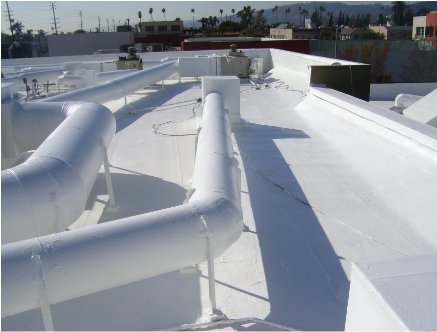
Figure 9.16 In a renovation project, the roof of this art studio in Hollywood, California, was coated for waterproofing with SureCoat, a white finish, which could be applied to the mechanical system as well, giving it a very high reflectivity, or albedo. Research by the Lawrence Berkeley National Laboratory and the Florida Solar Energy Center has demonstrated that light-colored roofs with a high SRI use 40 percent less energy than dark roofs. (All rights reserved. SureCoat Systems)
