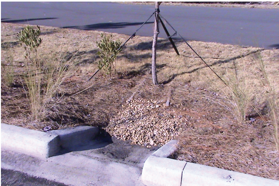
Figure 6.7 Bioswales surrounding the parking lot reduce stormwater runoff into nearby wetland areas. (Source: D. Stephany)
