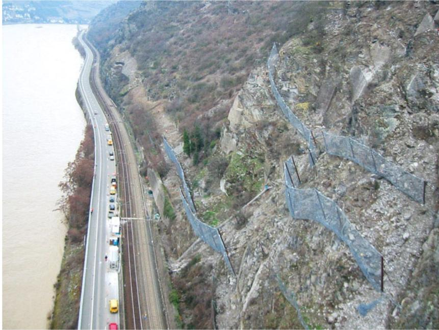
**Photo 2.4** Mitigation measures against rockfalls are usually costly. The most exposed sites are typically protected by special flexible anti-rockfall barriers. Elements of a particular protective system are chosen based upon the presumable power of a
