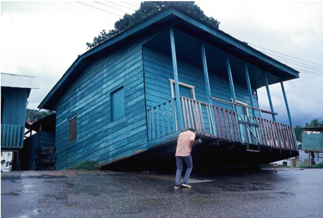
**Photo 3.33** In many cases, small houses are damaged by strong winds directly. The photo shows a house in Honduras that was blown off its foundation by Hurricane 'Fifi'. (Photo credit: UNESCO, M. Ginies, 1974)
