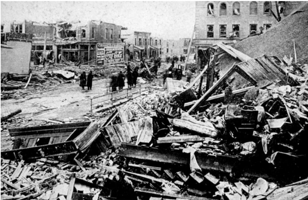
**Photo 3.7** The devastation shown in Omaha, Nebraska (United States), triggered by a tornado on 23 March 1913, is typical of combined devastation. Though whirl-type destruction prevailed, several buildings were subjected to by-blow and blast-type
