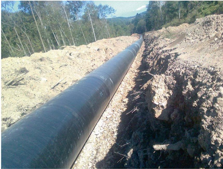
**Photo 12.10** The next stages in building a pipeline over land are: (3) making ditches; (4) laying the pipes along the route of the pipeline; (5) pipe bending; (6) welding; (7) wrapping the pipes with polymeric bands; (8) applying an insulating coating; (9) installing cathodic corrosion protection systems; (10) laying
