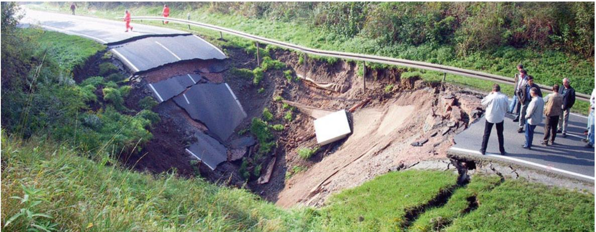
**Photo 1.29** The effects of karst on auto roads and railroads are also widespread. The photo shows damage to Road 180 due to a sinkhole in the south of Lutherstadt Eisleben, Germany, in 2001 (Photo credit: State Office for Geology and Mining, Saxony-Anhalt, Germany)
