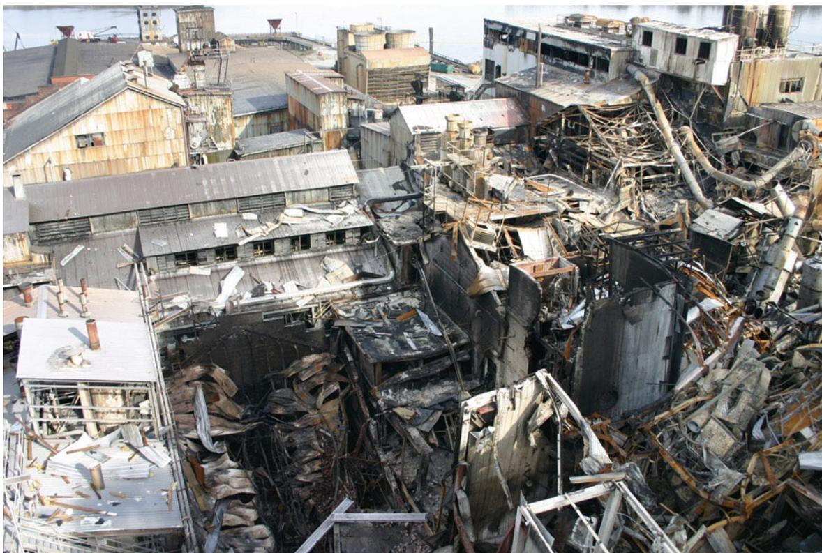
**Photo 9.37** Dust that forms in flour milling plants, sugar mills, and plants producing cocoa powder, dried milk, and other products is able to spontaneously explode. A view of the damage
