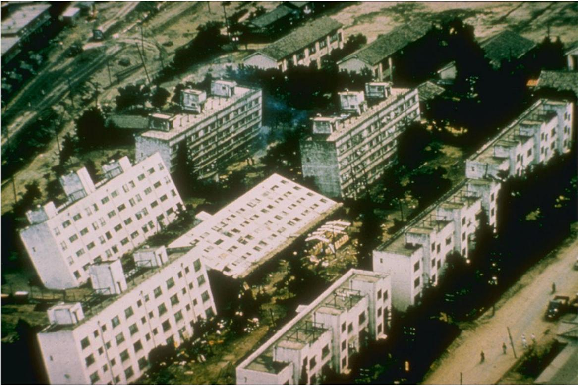
**Photo 1.3** Ground liquefaction during earthquakes is not widespread, since it requires coincidence of a number of conditions. This photo illustrates the negative impact of ground liquefaction. In the course of the magnitude 7.4 earthquake of 16 June 1964, Niigata prefecture, Japan, several big buildings slowly subsided and leant in liquefied ground. Thanks to the durability
