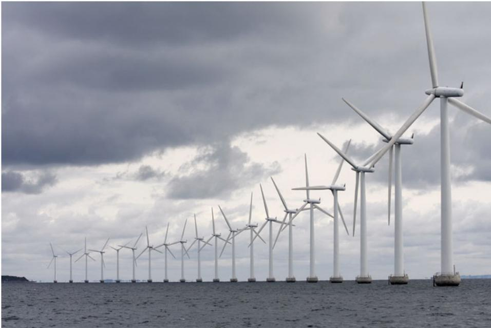
**Photo 8.15** According to where they are placed, the following types of wind power plants can be identified: (1) ground (wind turbines are usually installed in the hills); (2) coastal, or onshore (a small distance from the sea coast); (3) offshore (constructed at
