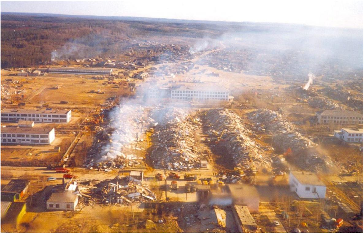
**Photo 1.2** The destructive character of the magnitude 7.5 Neftegorsk earthquake in Sakhalin on 28 May 1995 was caused mainly by the earth tremor. As a result, 17 of 22 panel five-storey buildings were completely ruined; two other buildings
