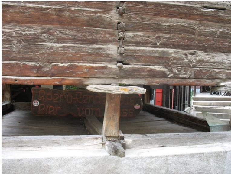
**Photo 5.117** One rodent control technique is prevention of their access to structures. The photo shows a storehouse built on piles with upper parts that end with stone plates, precluding the
