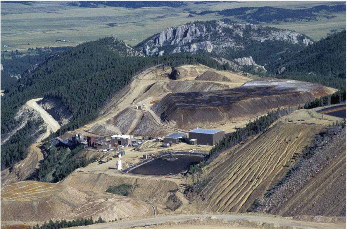
**Photo 10.14** In the case of heap leaching, the major factor causing adverse environmental influences is leakages that arise when the watertight diaphragms under the ore stacks and in the
