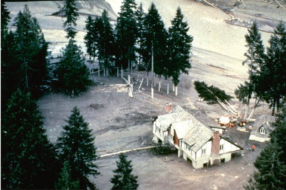
**Photo 1.9** Volcanic mudflows (lahars) appear when water-sodden ash glides down volcanic slopes. The photo shows a lahar-damaged house after the eruption of Mount St. Helens (United States) which occurred on 18 May 1980 at a distance of 40 km from the house. The mud coatings on trunks indicate the
