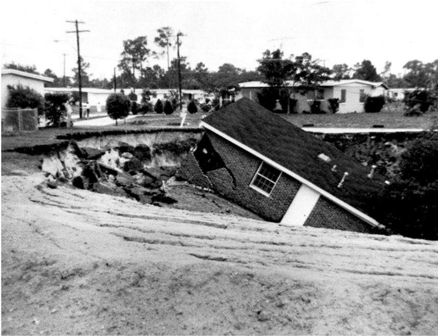
**Photo 1.28** Destruction of buildings is a typical consequence of sinkhole formation. This karst collapse took place on 22 May 1967 in the state of Florida (United States). The sinkhole had
