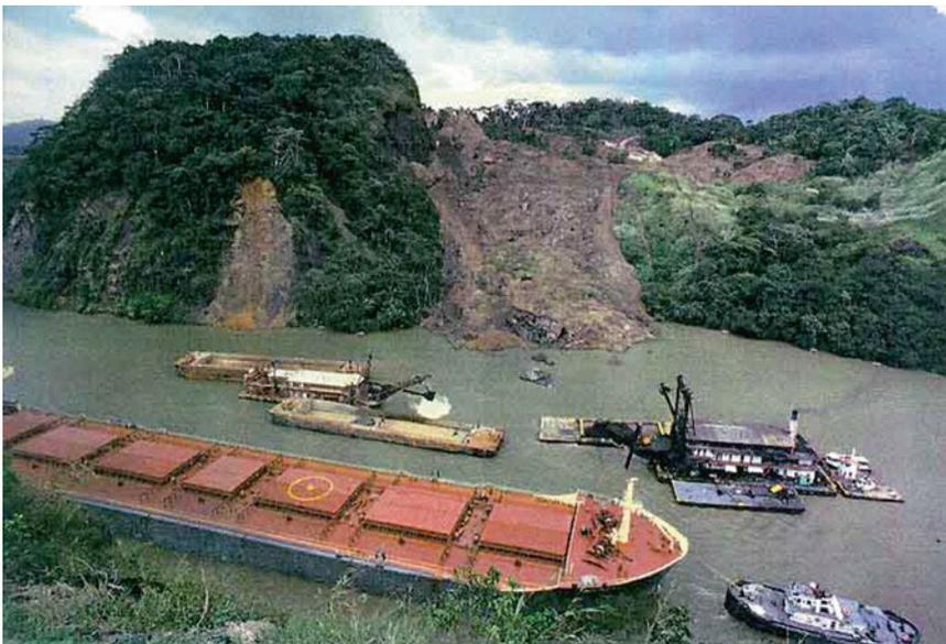
**Photo 2.18** Landslides frequently aggravate the construction and operation of channels since they cut down slopes and raise the level of groundwater. In particular, they seriously complicated the digging of the Panama Canal and prolonged construction. Landslides increased the excavation volume by 55.5 million
