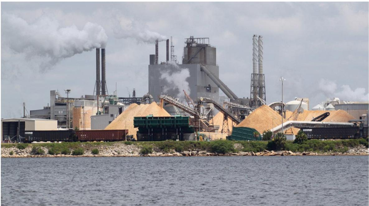
**Photo 9.28** Atmospheric pollution associated with wood pulp and paper plants occurs as a result of emissions of dust and gaseous substances. The solid particles include sodium and calcium compounds, and particles of starch, talc, lime, clay, and pigments. The gaseous pollutants include hydrogen sulphide,
