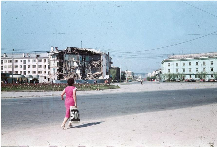
**Photo 1.18** The photo shows a wall collapse in a dwelling in Yakutsk, Russia, caused by thermokarst. Nobody was injured. To prevent such collapses, houses must be built on piles. Thereby, the air space under the house should prevent the heat impact on the frozen ground. This house was erected ‘low-sitting’, and for
