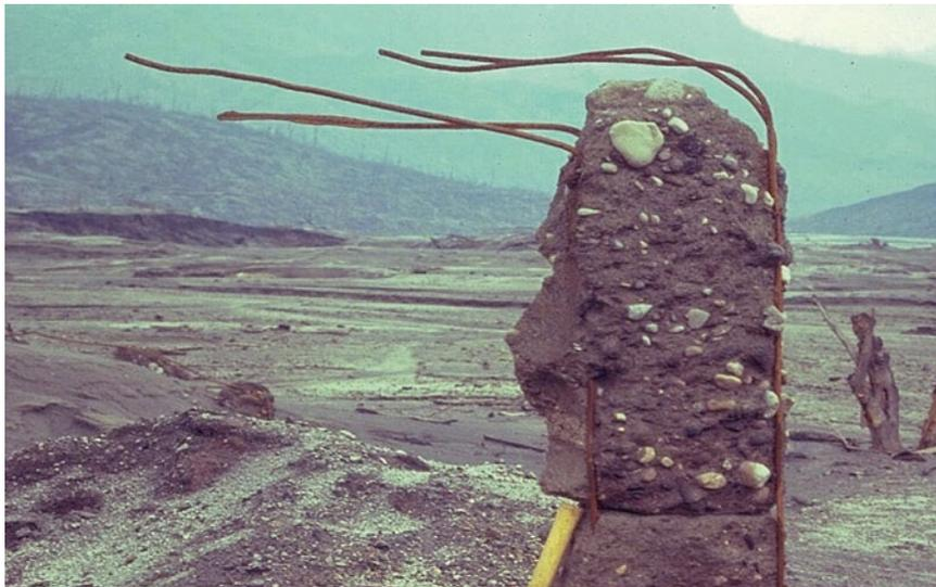
**Photo 1.8** Burning volcanic clouds are a mixture of volcanic gases and tephra. Their destructive effects are caused by high temperatures that lead to fires and by high pressure due to considerable density of clouds and high speeds of their displacement. This photo shows the ruins of a house in the village of Francisco Leon, south-eastern Mexico, destroyed by the burning volcanic cloud during the El Chichón volcano eruption from
