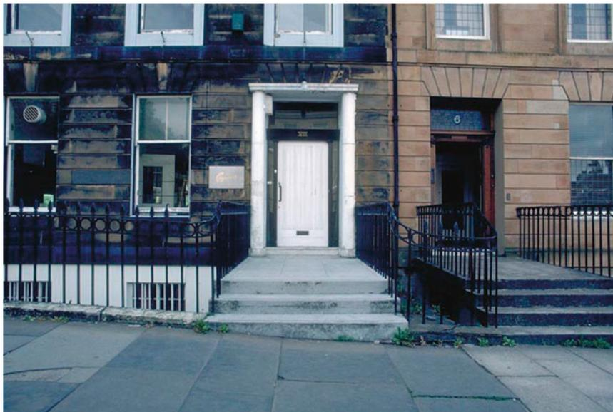
**Photo 8.7** This picture shows long-term effects of coal burning in Glasgow, Scotland. The building on the right was recently cleaned (Photo credit: Marli Bryant Miller, Department of Geological Sciences, University of Oregon, United States)
