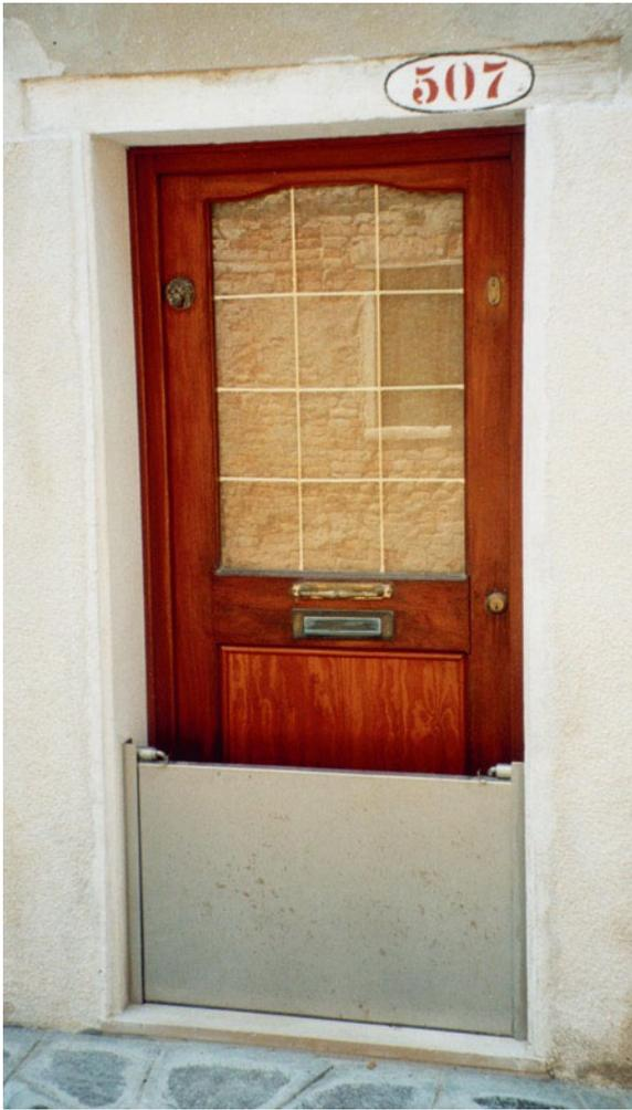
**Photo 4.8** Wind-induced surges are typical of Venice, Italy. The photo shows a house door with an additional hermetic barrier, which protects the house from seawater (Photo credit: Lee Boshier, Loughborough University, United Kingdom, August 2003)
