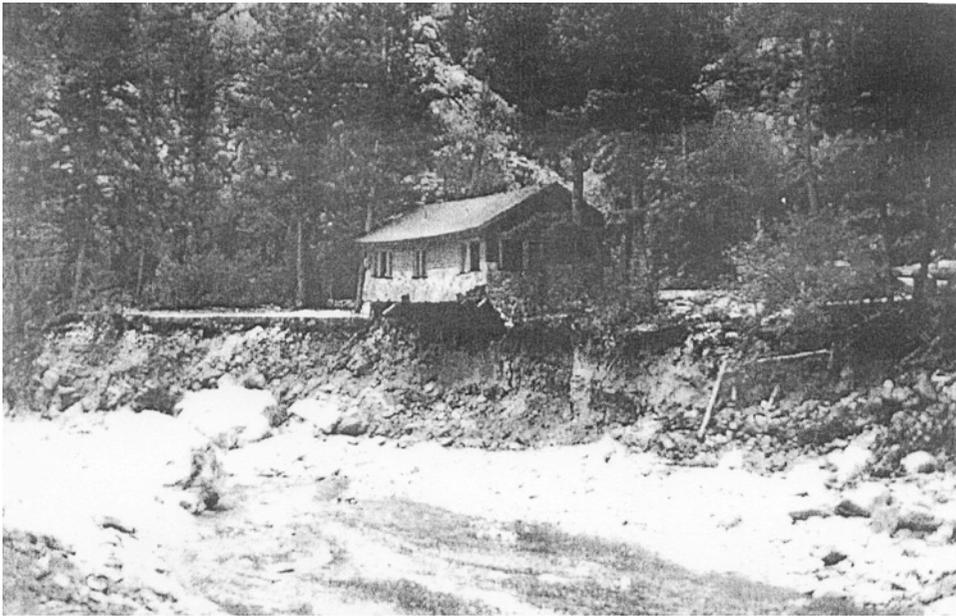
**Photo 2.38** Riverbed erosion has various impacts on dwellings. One of the major factors is damage and destruction of houses owing to riverbank cut-offs. The photo shows a house in
