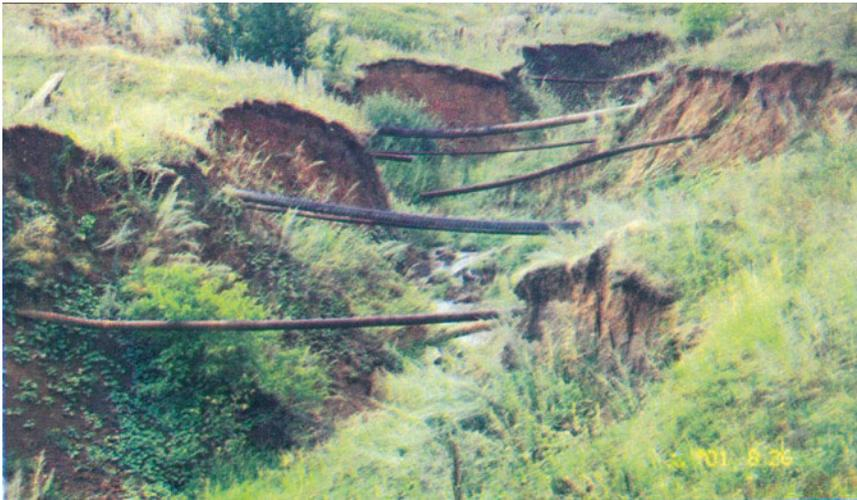
**Photo 2.34** Formation and growth of ravines influence pipeline transport. The photo shows the exposition and deformation of oil pipelines in the Yelabuga district of the Republic of Tatarstan
