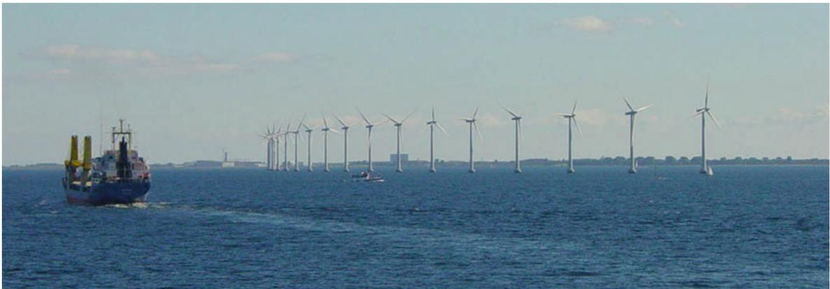
**Photo 8.16** Middelgrunden is an example of an offshore wind farm. It is in the Øresund, 3.5 km outside Copenhagen, Denmark. When it was built in 2000, it was the world's largest offshore wind farm, with 20 turbines and a capacity of 40 MW. The farm
