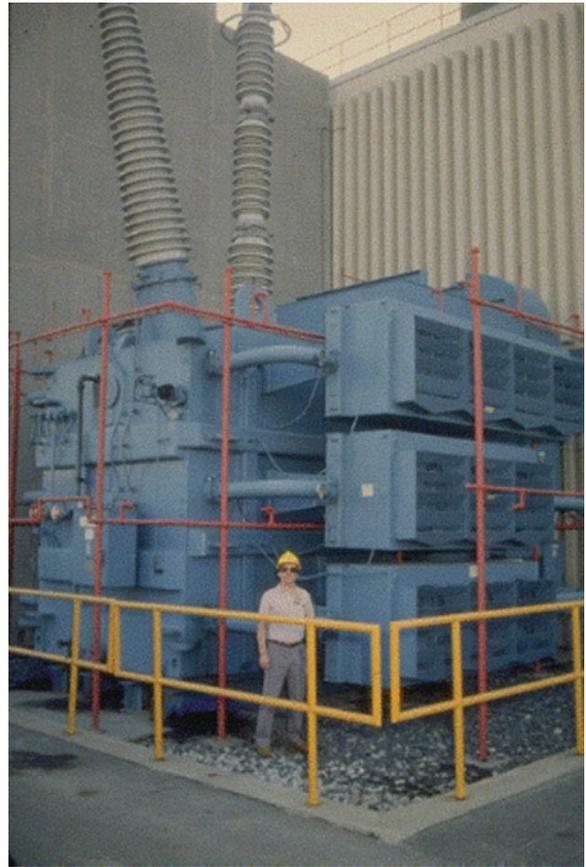
**Photo 7.5** The magnetic storm on 13 March 1989 disabled the transformer in the Salem Nuclear Power Plant (New Jersey, United States) due to overheating; the transformer had to be replaced. Economic losses amounted to several million dollars. The photo shows the damaged transformer (Photo credit: John Kappenman, Public Service Electric and Gas of New Jersey)
