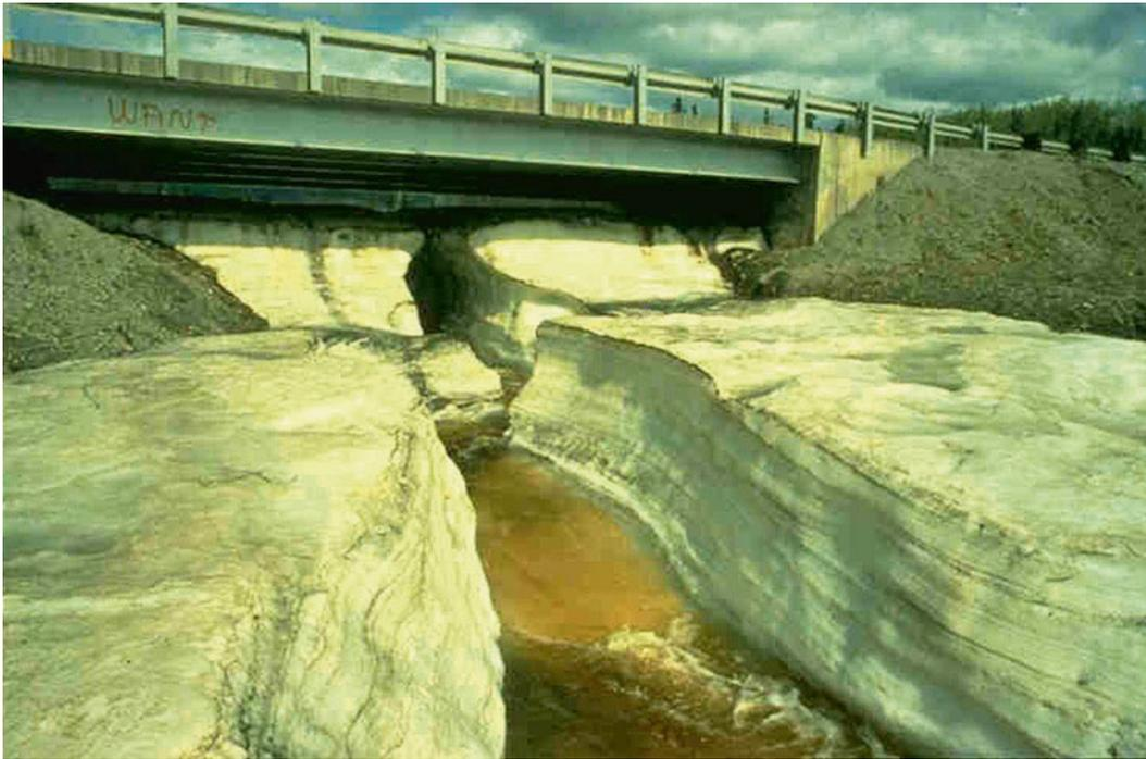
**Photo 2.26** Aufeises also block up water pipes and sewage outlets. Hence, in the springtime, water washes away roadbeds and destroys bridges. The photo shows melting aufeises in the
