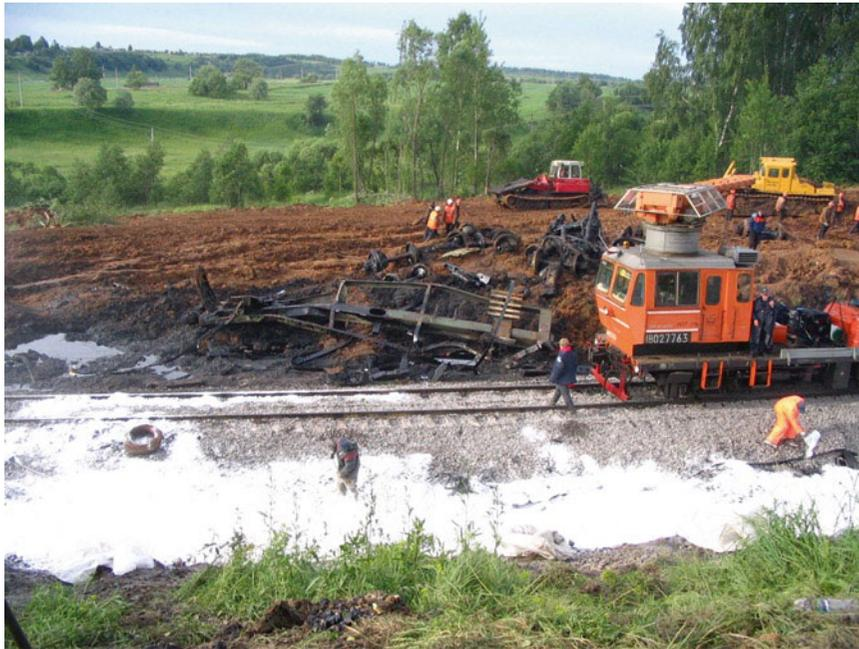
**Photo 12.8** The scales of contamination in rail transport increase many times in case of emergency. As a result of a derailment of a freight train on 15 June 2005, near Rzev (Tver oblast, Russia), 21 tanks with fuel oil overturned. Altogether, about 300 ton of oil products were released. Removing the
