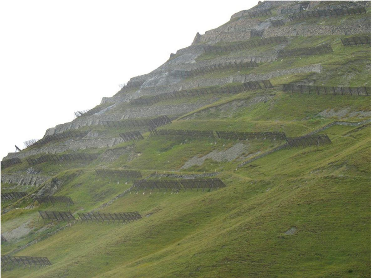
**Photo 2.11** There are many ways to protect objects and people from avalanches. One of them is erecting snow-stabilizing barriers. The increase in roughness of the slope surface helps stabilize the snow blanket and prevents avalanches from passing. The
