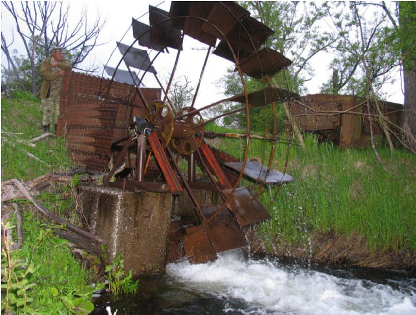
**Photo 8.4** In small water courses, hydroelectric stations designed to supply electricity to small power users in remote areas are not infrequently constructed. The photo shows one such
