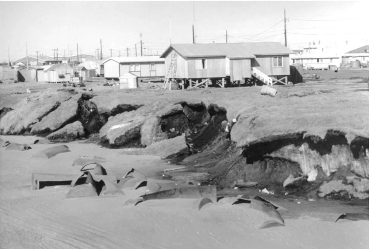
**Photo. 1.20** The average rate of thermoabrasion does not exceed 0.5–1.0 m/year; however, it may become as high as 10 m/year. Coastal retreat occurs mostly during 2–3 summer months; the process dramatically intensifies at times of heavy storms. The
