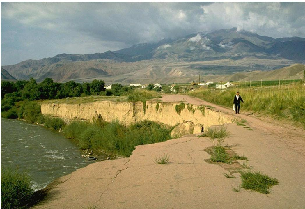
**Photo 2.39** Impacts of riverbed erosion on auto roads and railroads are, in most cases, exerted through lateral erosion too. The photo shows the destruction of a roadbed as a result of riverbank
