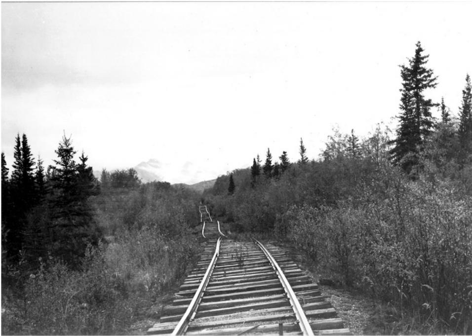
**Photo 1.19** Thermokarst poses a formidable threat to railroad maintenance. The photo illustrates the numerous deformations of the Northwestern Railway near Strelna, 75 miles northeast of Valdez, Alaska (United States). The thermal equilibrium of the fine-grained sediments underlying the roadbed was disrupted
