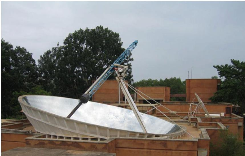
**Photo 8.14** This photo shows the Solar Bowl in Auroville, India. It used solar energy for cooking. The ferrocement base of this stationary bowl faces south. It is 15 m in diameter and 7 m above ground level. The sun's rays, trapped by a huge hemispherical mirror, focus on a cylindrical boiler that fol-
