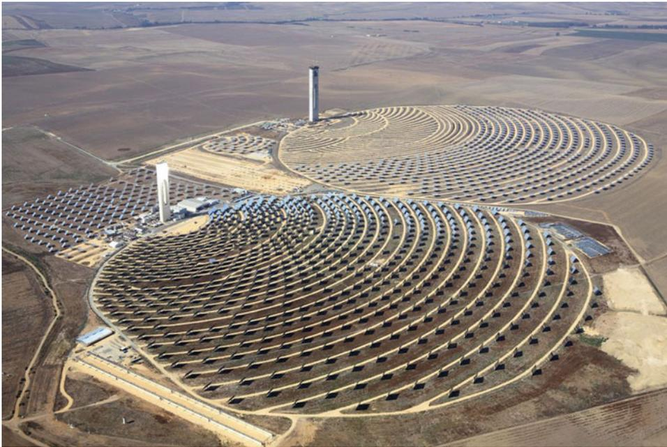
**Photo 8.13** The construction of solar power stations needs large areas of land. A power plant producing 1,000 MW in a hot, dry locality (such as west or central Australia) will need a total collector area of 13–25 km<sup>2</sup>. This area is more than that occupied
