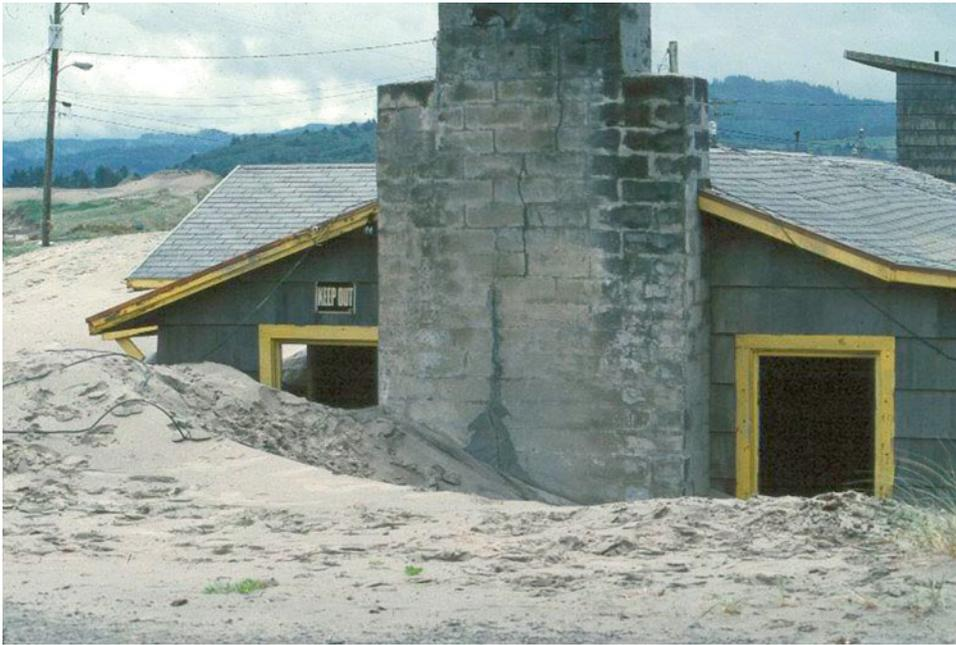
**Photo 2.28** Burial of objects with sand is typical not only of deserts but also of seaside areas. The photo shows a house being buried with sand along the coast of Oregon (United States)
