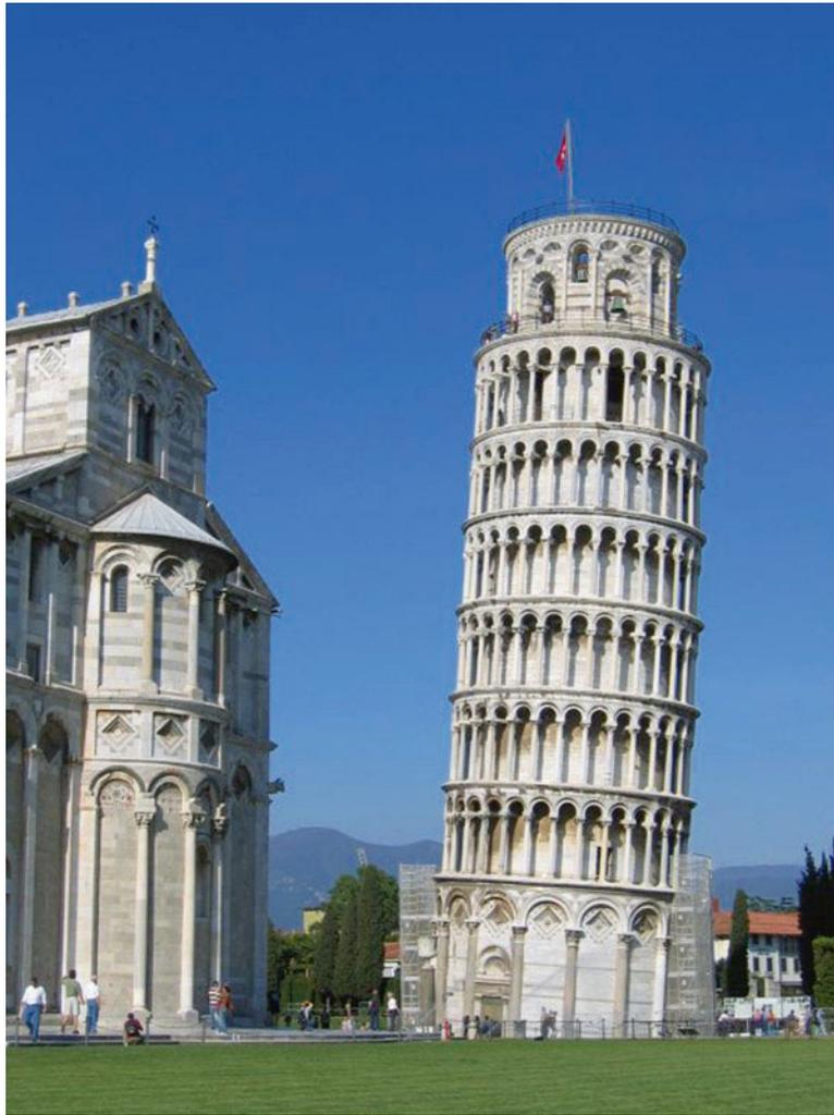
**Photo 1.33** The Tower of Pisa stands on limous and clayey ground. Its ‘fall’ is caused by nonuniformity of subsidence of underlying ground. Its south side subsided 3 m deep, and the north, 1 m deep. Non-uniform subsidence has been occurring for
