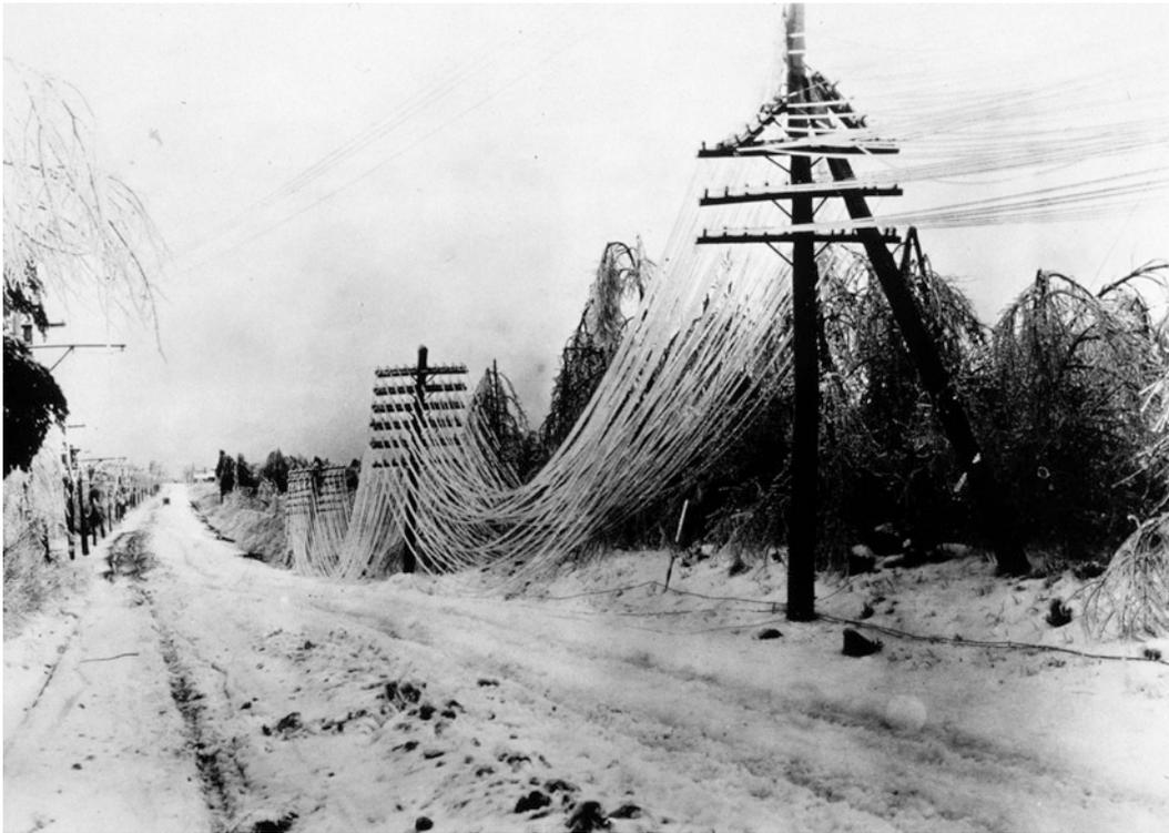
**Photo 3.44** Ice-up destroys communication and power lines. The weight of ice crusts can reach 86 kg/m. The photo shows a telephone line covered with ice in the United States (Photo credit: U.S. National Oceanic and Atmospheric Administration)
