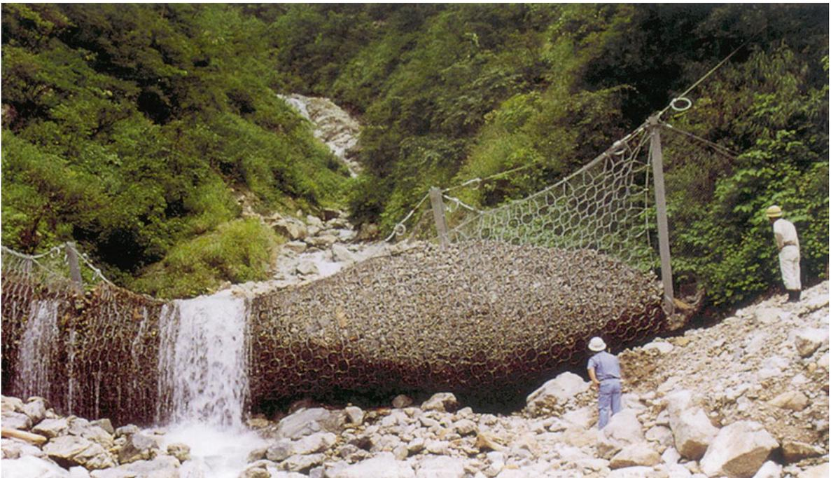
**Photo 2.23** Protective measures against mudflows are varied. One of them is installation of flexible mesh barriers. The photo shows a flexible mesh barrier in the area of Aobandani, Japan, to protect against debris flow. It is 20 m long and 4 m high and is
