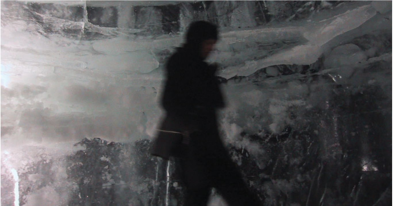
The temperatures of the different days were registered as ledges on the wall. The colour of the surface changed as the colour of the water pumped from the sea had varied. The thickness alternated according to the outside temperature and directions of the wind on the site. Some ice was white, almost like snow, and some was so clear that one could see outside.
