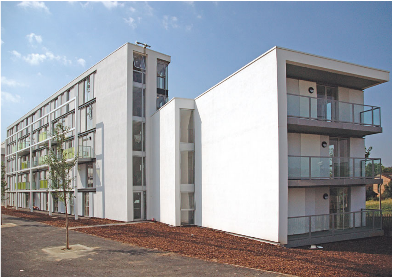
Block J, the most northern of the buildings on the site, contains the units available for shared ownership. While all the apartments are single aspect, the ample glazing and use of balconies ensure that each unit has plenty of natural light and interesting views out over the site to the city beyond.
