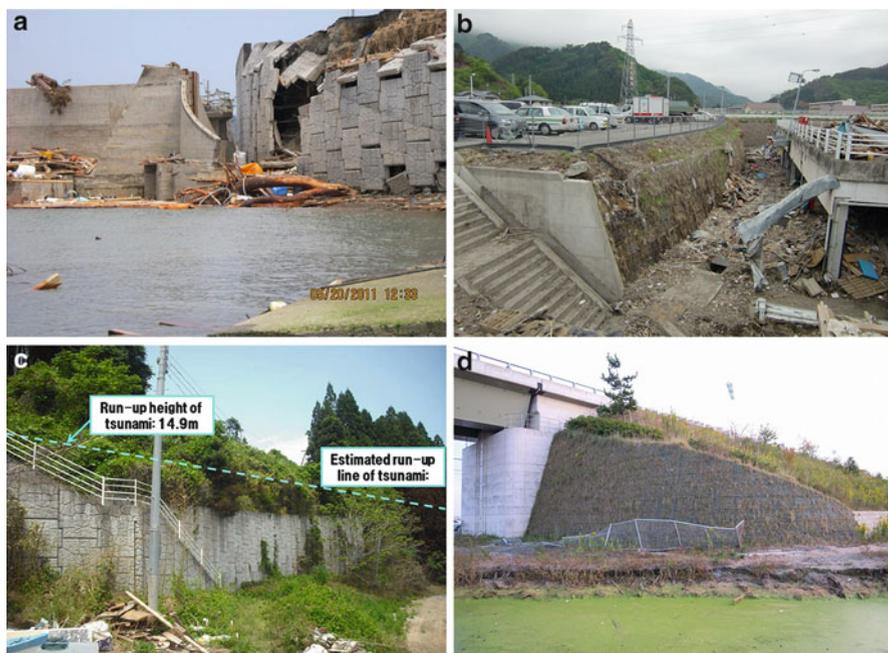
**Fig. 12.11** Performance of reinforced soil wall against seismic motion and tsunami action. (a) Case 8: ultimate limit state. (b) Case 9: serviceability limit state. (c) Case 10: no damage. (d) Case 11: no damage (a and c: by courtesy of Dr. Otani: Hirose Co.; b and d: JC-IGS Technical Committee (Dr. Hironaka))
