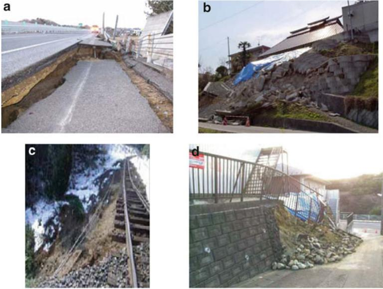
**Fig. 12.7** Damage to non-reinforced soil structure during great East Japan earthquake. (a) Subsidence of highway embankment (East Nippon Expressway Company, 2011). (b) Collapse of retaining wall on local road (JC-IGS Technical Committee, 2011). (c) Collapse of retaining wall on railway track (East Japan Railway Company, 2011). (d) Collapse of retaining wall at housing site (Koseki et al. 2011)
