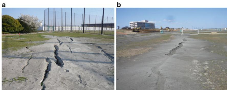
**Fig. 4.35** Linear fissures in wide flat ground. (a) Cracks at Sports Park at Urayasu. (b) Cracks on the elevated bed of the Tone River
