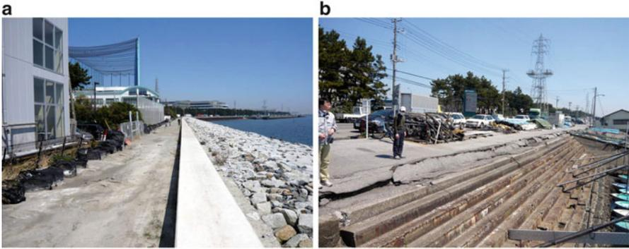
**Fig. 4.26** Ground damage at Shiohama, Ichikawa, Chiba-city. (a) Damaged steps in the fishery port with the lateral displacement of about 50 cm – a view to the east. (b) A view of the undamaged seawall (center) with extensive liquefaction at inland walkway – a view to the east
