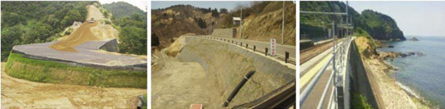
**Fig. 12.4** Earthquake disaster rehabilitation by reinforced soil wall
