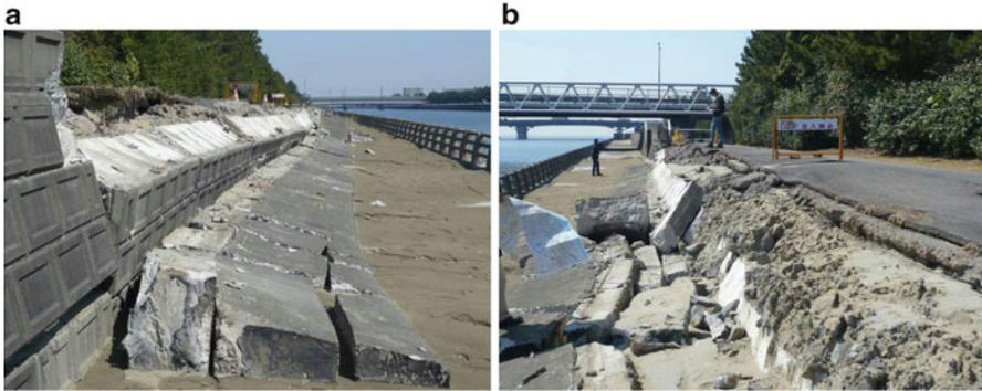
**Fig. 4.32** Failure of the walkway wall on the north of the Hanami River. (a) Collapse of the wall north of The Hanami River – viewed from the west. (b) Collapse of the wall north of the Hanami River – viewed from the east to the sea
