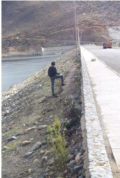
The estimate accelerogram at the site of Paloma dam has  $PGA = 0.661 \text{ g}$  and  $P_D = 43.59 \cdot 10^{-4} \text{ s}^3$ , for this accelerogram the dam suffered a vertical settlement of the core of 68 cm shown in Fig. 7.2.
