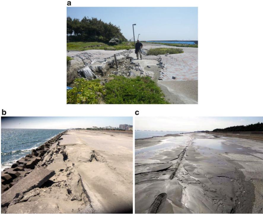
**Fig. 4.24** Lateral spreading towards the sea behind the cemetery park at Hinode-8, Urayasu. (a) A depression of the ground inland of the seawall – a view to the east. (b) Damage at the edge of the apron – a view to the west. (c) Sand gushing from a seam of pavement over the apron in front of the seawall – a view to the west
