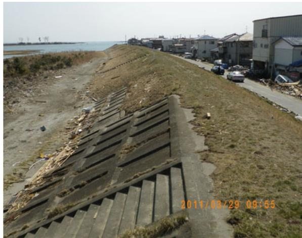
Figure 6.10 shows a levee of Kitakami River (Fig. 6.2) that was destroyed by run-up of tsunami. Figure 6.11 in contrast illustrates a Natori River levee (Fig. 6.2) that survived the overtopping of tsunami water. The different performance of the two levees may be interpreted as what follows and facilitates future tsunami mitigation;
