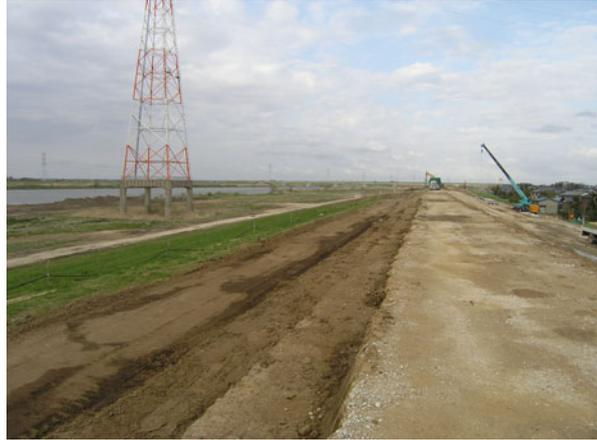
**Fig. 6.20** Reconstruction of land side of Tone River levee at Sakae by installing sheet pile walls with holes
