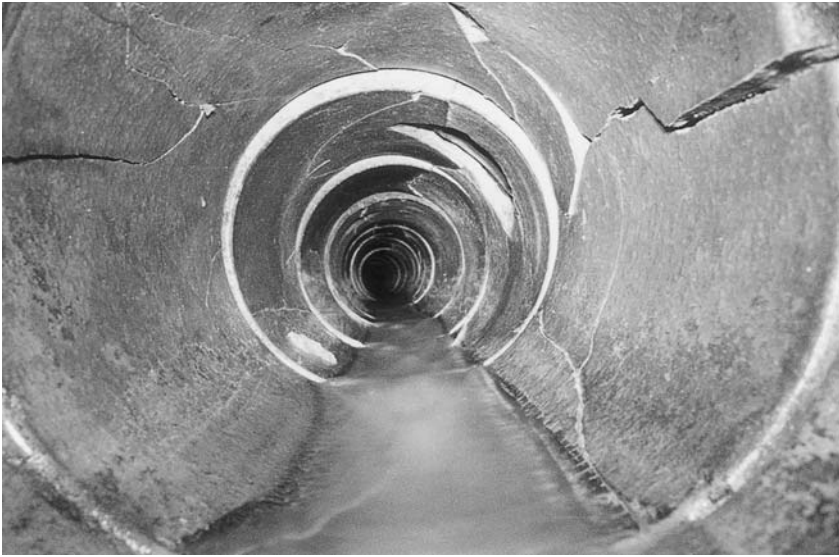
Fig. 17.2 CCTV image of a sewer in poor condition (courtesy of Telespec Ltd, Guildford)
