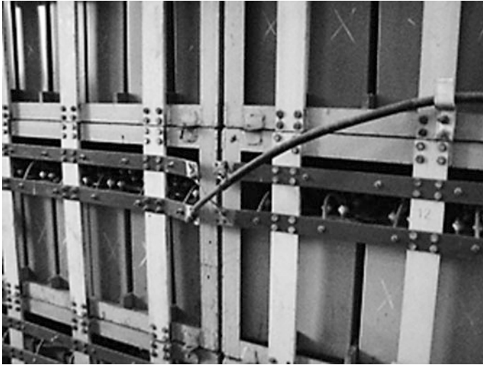
Fig. 2.10 Connection of the capacitor banks' cells [26]
