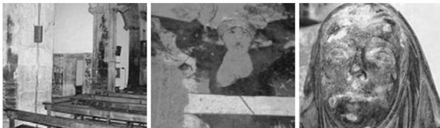
Fig. 2.1 Some examples of heritage degradation by hygrothermal behaviour (Guimarães et al. 2011)
