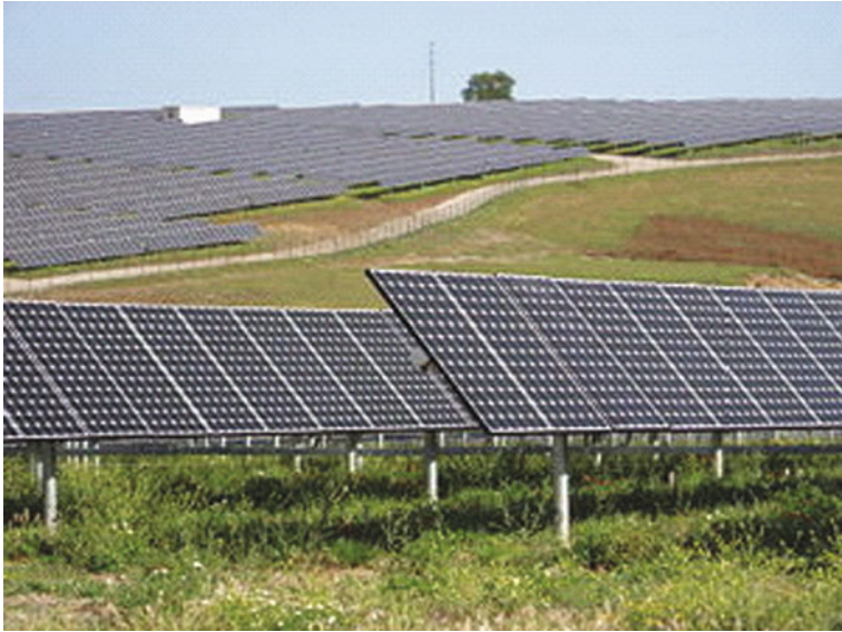
Fig. 13.2 Solar power plant near Serpa, Portugal ( 38^{\circ}1'51''\text{N} , 7^{\circ}37'22''\text{W} )
