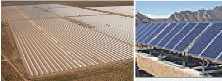
Fig. 13.1 Solar photovoltaic cells using for generating electricity
