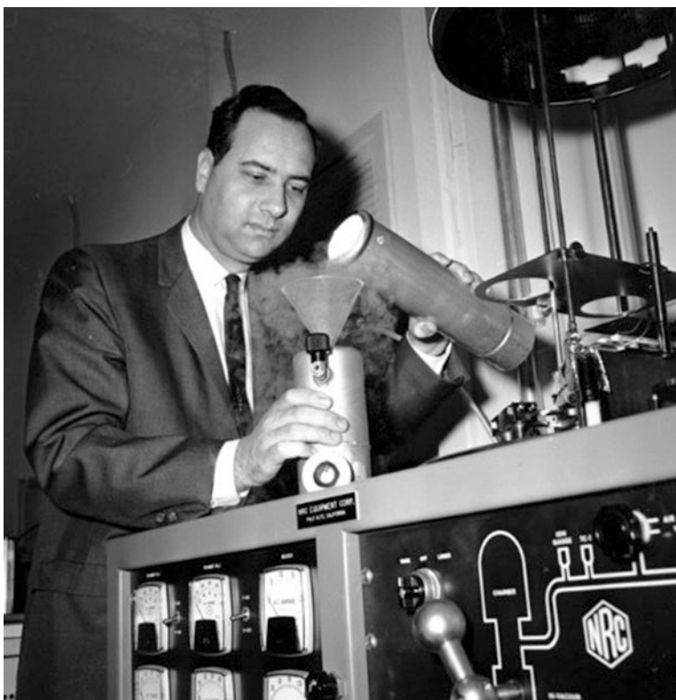
Ted pouring liquid nitrogen into a cooling unit around an experimental laser in his laboratory at Korad Corporation, 1960s. Courtesy of the Union Carbide Corporation
