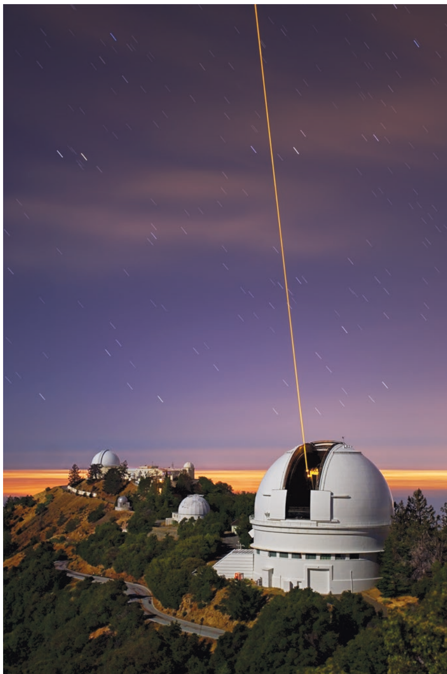
Laser guide star technology which has greatly sharpened the ability of land-based telescopes to see deep into the universe; shown at Lick Observatory, University of California. ©Laurie Hatch
