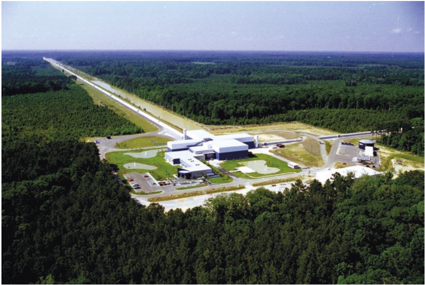
Laser Interferometer Gravitational-Wave Observatory (LIGO), which in 2015 provided first detection of gravity waves, confirming Einstein’s 1915 prediction; installation at Livingston, Louisiana, with two 2.5 mile (4 kilometer) arms. Courtesy of Caltech/MIT/LIGO Lab
