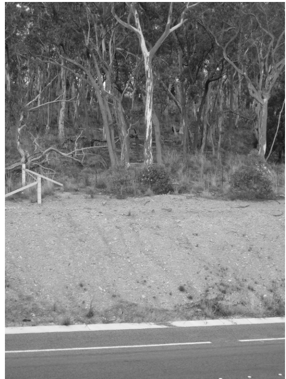
FIGURE 12.2. A road verge slope showing signs of sheet and rill erosion caused by excessive overland flows from above the roadway. Flows have also washed away the mulch that was originally applied to this slope.
