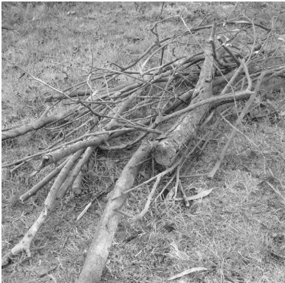
FIGURE 11.12. Brush packs constructed on the slopes of former farmland pastures to obstruct sheet flows.
