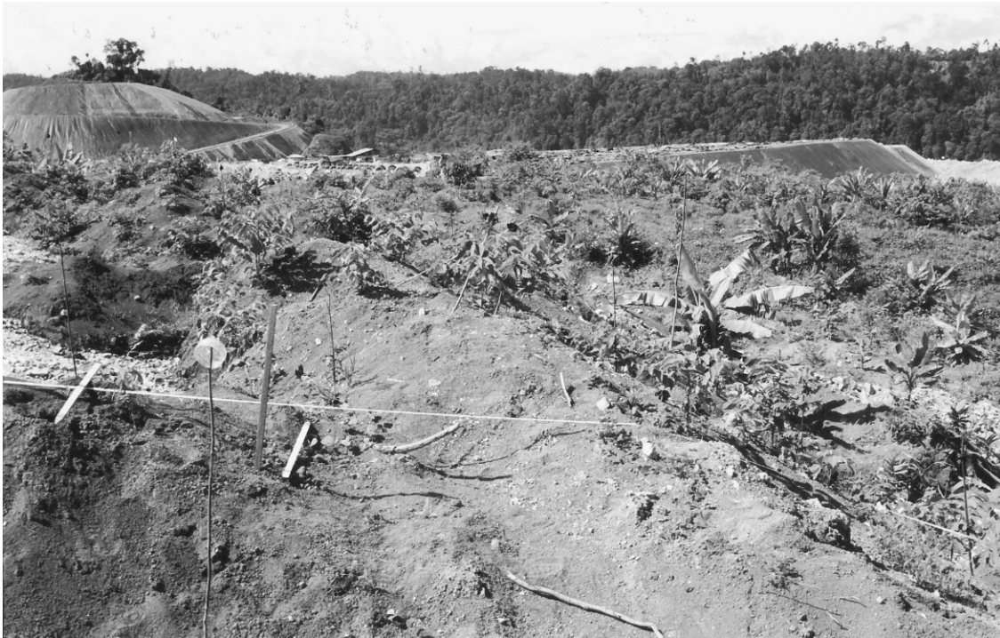
FIGURE 4.16. Topsoil has been dumped in discrete heaps to form a patchwork of microcatchments across a slope on a mine site in East Kalimantan.
