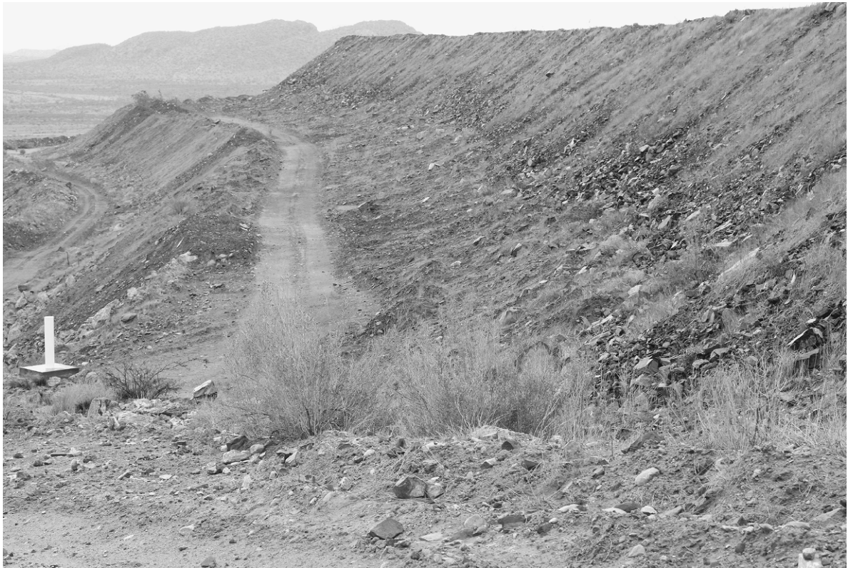
FIGURE 7.2. Stepped walls of a tailings storage facility built from dry tailings and covered with nonreactive waste rock.
