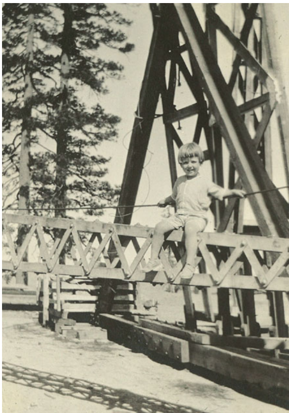
Fig. 4.9 Billy sits on a steel girder during the construction of the 100" dome in 1915
