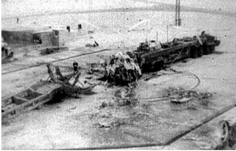
Figure 2.9: Wreckage of the rocket and the launch site structures in the aftermath of the R-16 explosion. (Courtesy Russianspaceweb.com)
