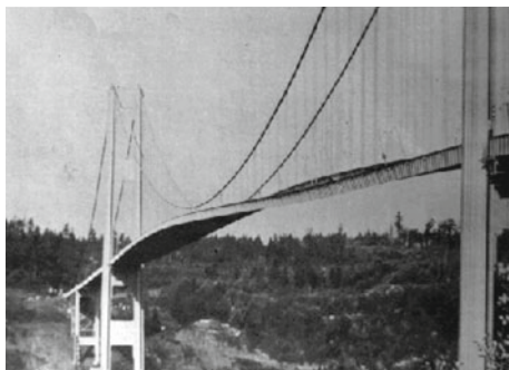
Fig. 2.7 Vibration of the Tacoma Narrows Bridge prior to the 1940 collapse
