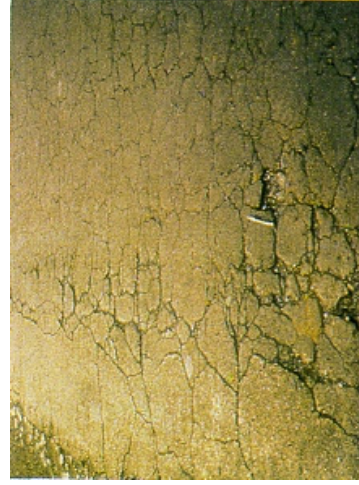
Photo 15 Generalized crazing with fish net cracking; losses of materials with
