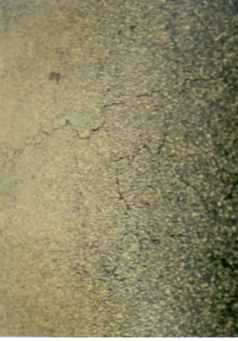
Photo 13 Fine crazing with large map cracking
