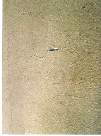
Photo 8 Branching longitudinal crack
