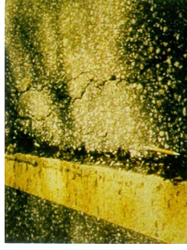
Photo 18 Wide branching centreline crack stripping
