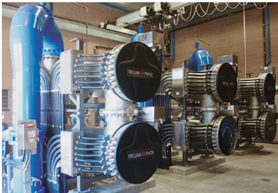
Fig. 5.2 An AOP plant for groundwater treatment for photolysis of volatile organic compounds (VOCs) by UV radiation. Courtesy of TrojanUV
