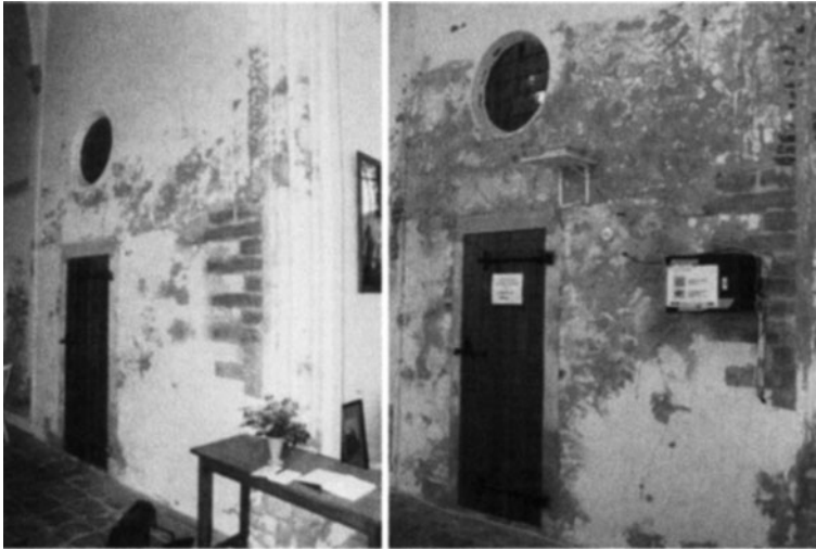
Fig. 9.8 Deterioration of a new render between 1991 and 1995 in an ancient building in The Netherlands
