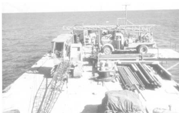
Figure 16.24 Example of coring from an anchored barge (ca. 1955)
