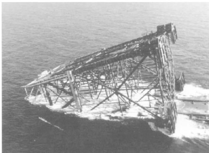
Figure 14.27 Launching of a 4-Leg Jacket
