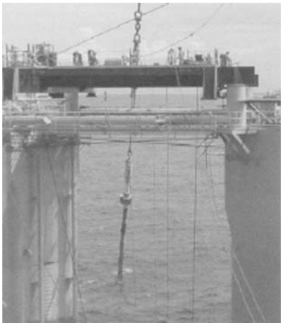
Figure 9.64 The Prince SCR during hang-off installation showing the pre-installed VIV stakes [Gore and Mekha, 2002]
