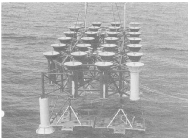
Figure 14.20 Subsea template lifting
