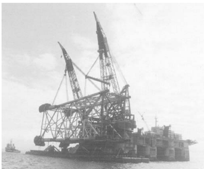
Figure 14.1 Two block upending (Marathon East Brae jacket)
