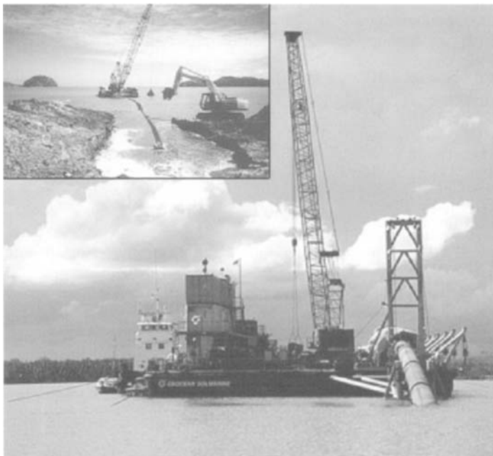
Figure 14.30 Shore pull operation
