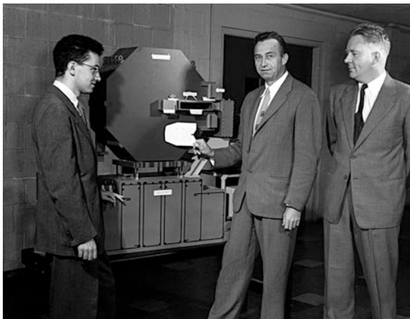
Fig. 2.8 Snyder, Livingston and Courant (from right to left) are pictured in front of the mock-up of a strong focusing bending magnet (From Panofsky) (Courtesy of Brookhaven National Laboratory)
