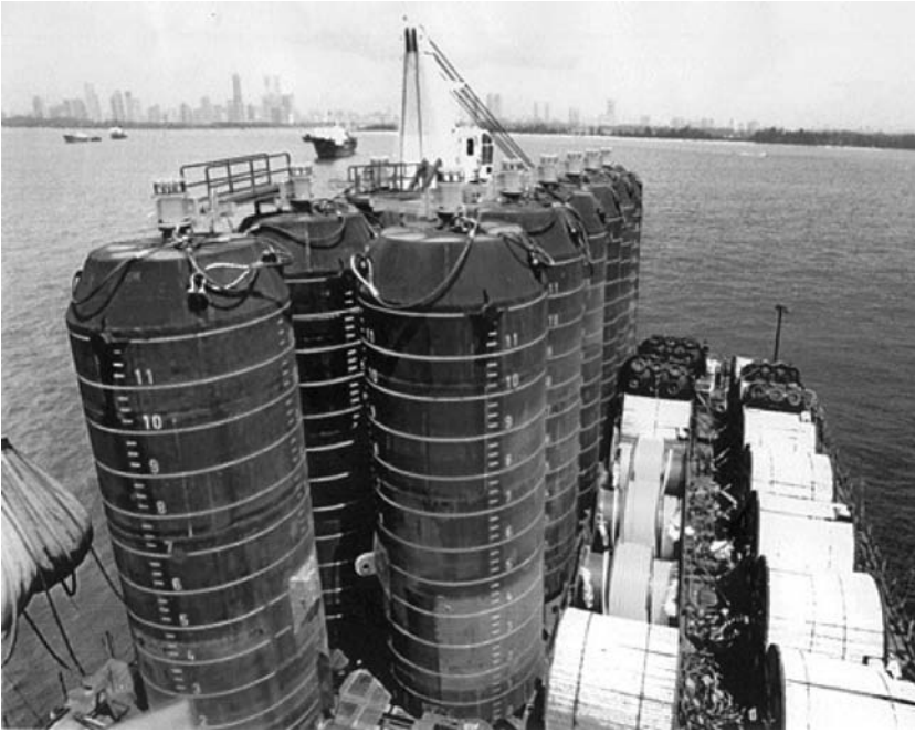
Figure 1.9 Suction anchors assembled on load out vessel
