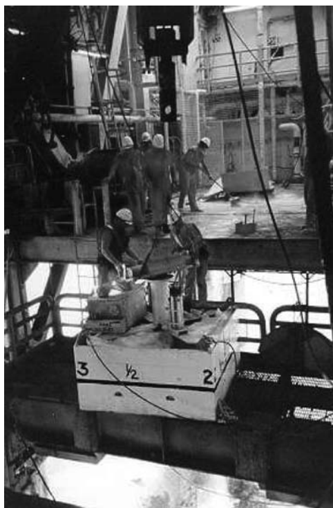
Figure 3.26 Seabed frame (SBF) being prepared
