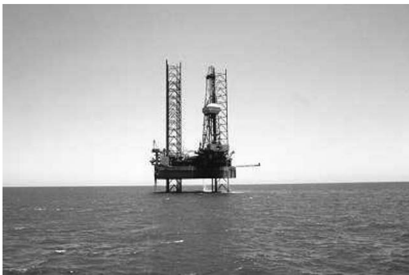
Figure 3.21 Jack-up drilling rig
