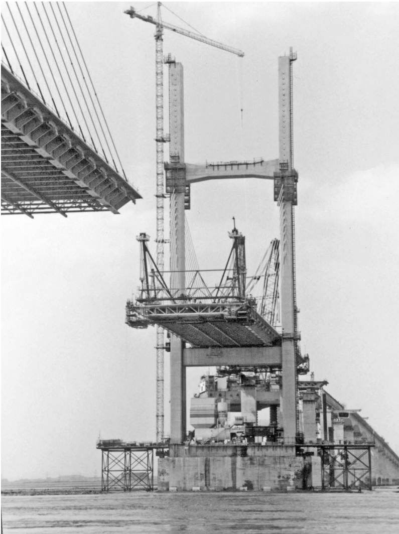
Figure 10.9 Cantilever construction of the Second Severn Bridge (© T Hambley)
