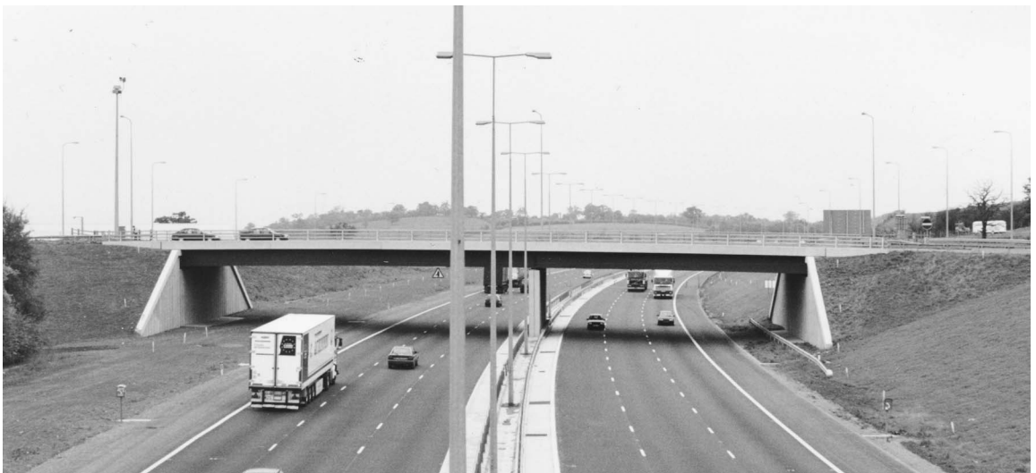
Figure 4.1 Continuous steel–concrete bridge spanning the M5 motorway (Collings, 1994)
