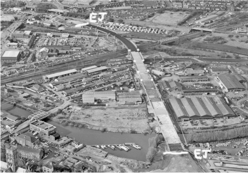
Figure 5.4 Aerial view of the Doncaster viaduct showing fixed bearings and joint locations. (Image courtesy of Morgan Sindall © unknown)
