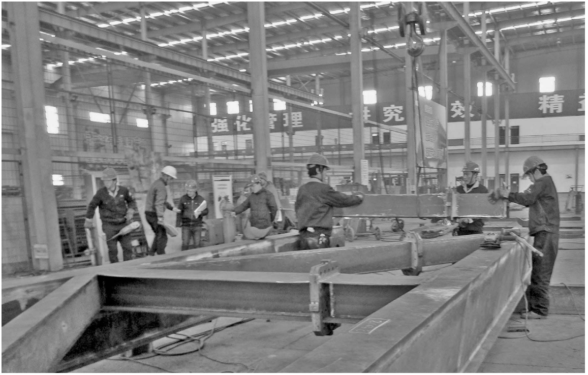
Figure 1.9 A fabrication factory in China working on a major truss structure (see Chapter 8)
