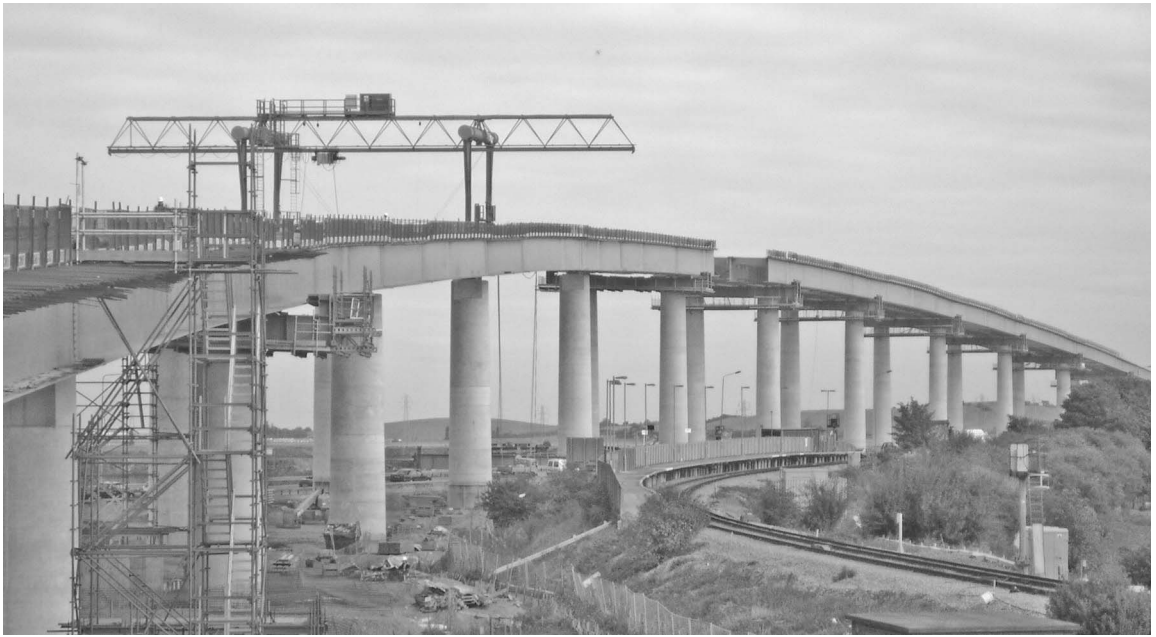
Figure 5.7 Sheppey bridge during launched construction
