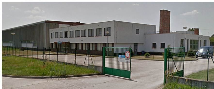
Fig. 12 WTP Kúty (view from the street)
