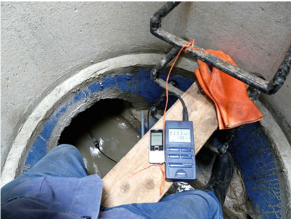
Fig. 13 Measuring device in a manhole
