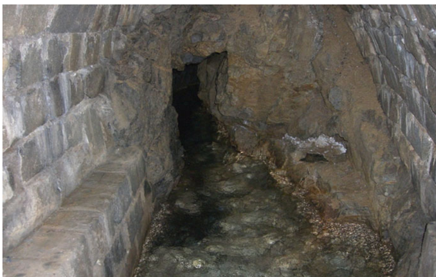
Fig. 15 The view into the side chamber with the groundwater flow from the rock massif (Photo: M. Fendeková)
