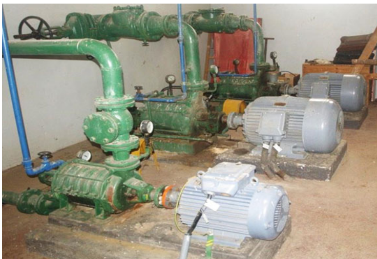
Fig. 3 Small irrigation pumping station for 300 ha (Photo: Jurík, 2016)
