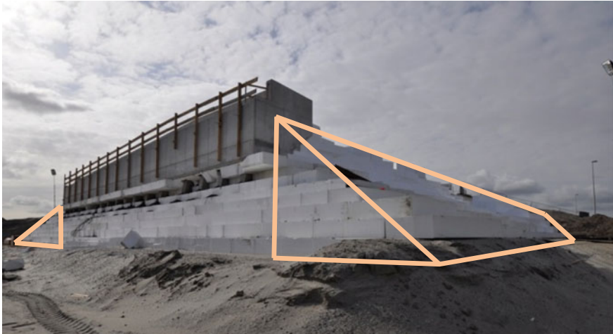
Fig. 6 Constructively unnecessary embankments made from EPS blocks: sections between the lines (reference: highway N207)
