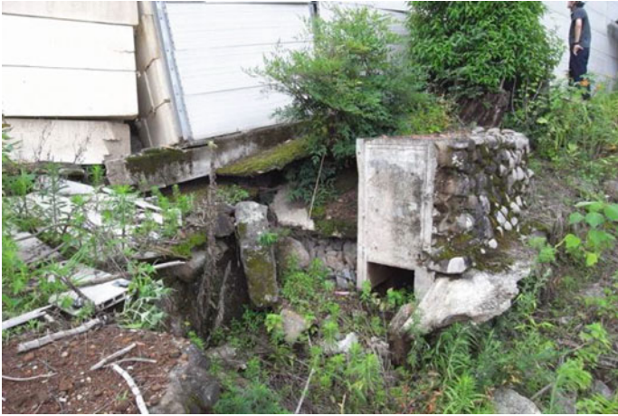
Fig. 8 EPS concrete foundation
