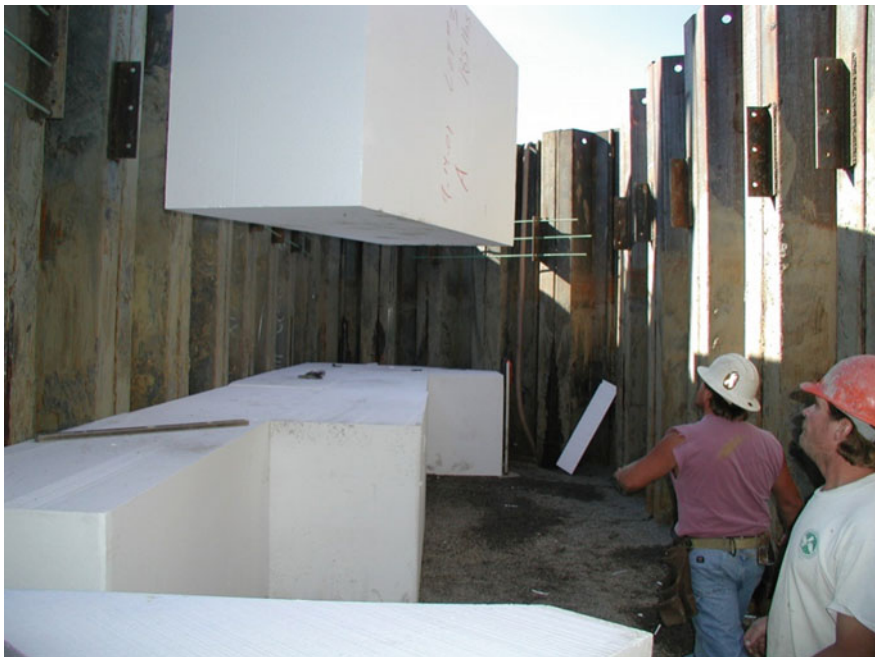
Fig. 20 Geofoam placement within the sheet pile cell (30)
