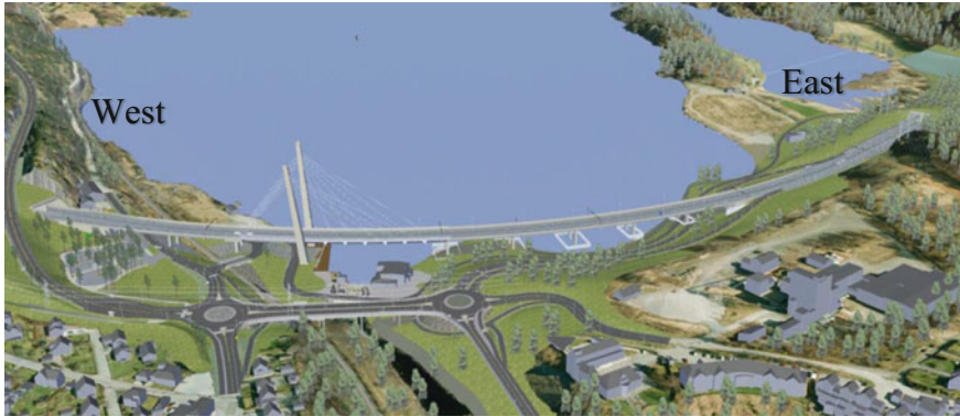
Fig. 1 Overview of Farris bridge
