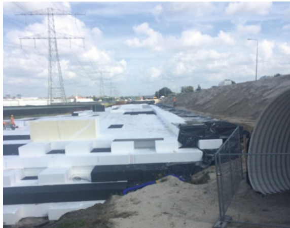
Fig. 5 Lightweight EPS-geofoam embankment (eastward) of the roundabout of the N222
