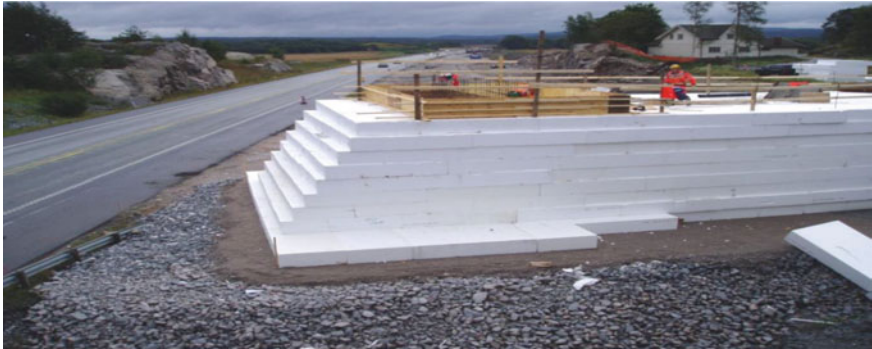
Fig. 6 Gimsøyveien bridge during construction
