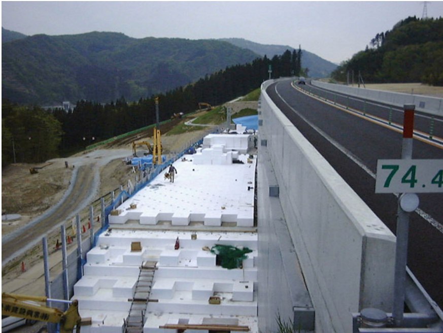
Fig. 4 Yamagata Expressway, Japan with vertical side walls (EDO)
