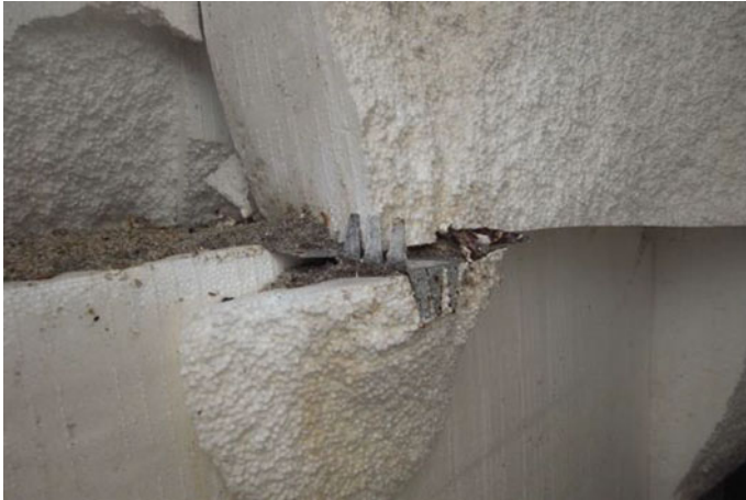
Fig. 6 JMB remained in position
