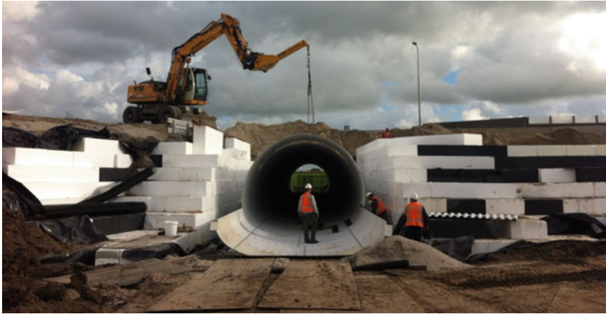
Fig. 6 Construction of the corrugated steel sheets tunnel under the N222
