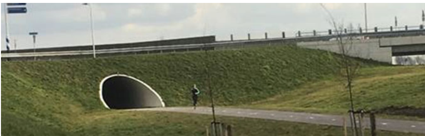
Fig. 28 Finished structure (InfraDelft)
