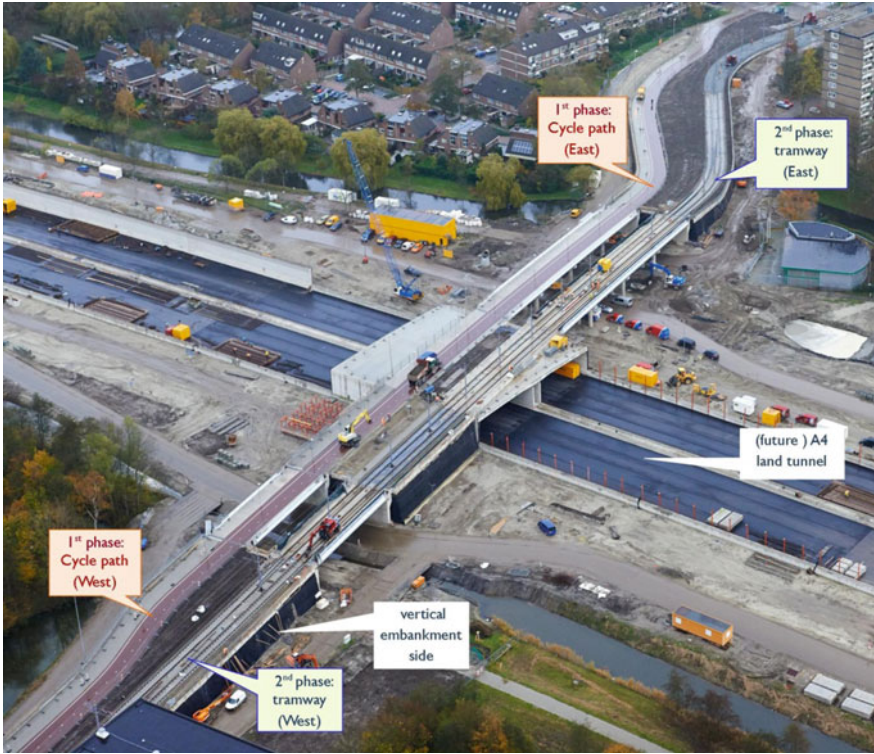
Fig. 5 The two-stage realization for the cycle path/calamity road on one side and the tramway over the A4 on the other
