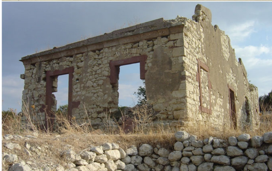
Fig. 13 Casa Prunas: localization of “casa Prunas” in the historical cadastral map (courtesy of Archivio di Stato di Nuoro) and view of the house in the summer of 2007
