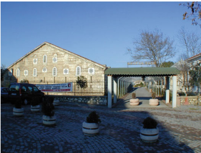
Fig. 3 The Sultan Süleyman Han caravanserai and the new access to the area (© Orlandi)
