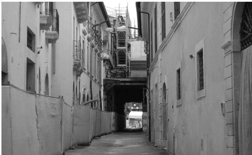
Fig. 2 The restoration of the city: construction sites along the streets of the historic centre
