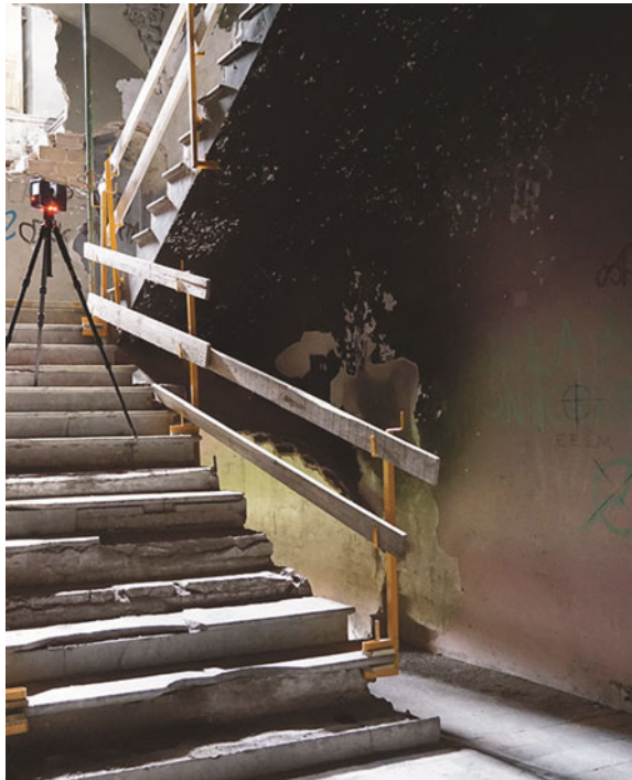
Fig. 10 Imperial staircase. Ground floor
