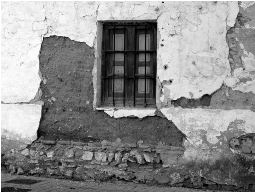
Fig. 13 A wall in Bargas
