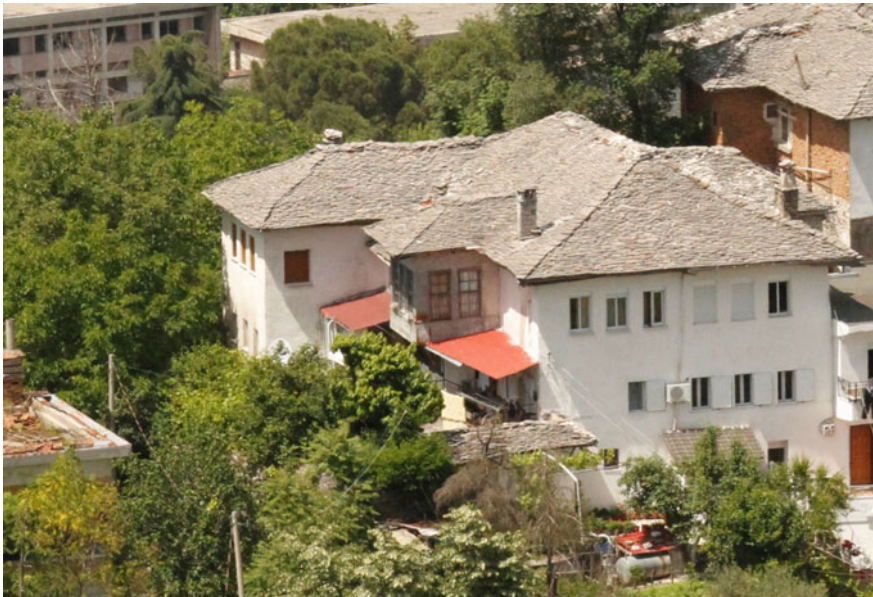
Fig. 5 Traditional House in Hazmurat neighborhood that is now delisted. As can be seen the house, features, traditional roof, kiosk, windows and stone walls and has only some minor interventions like the metallic eaves in ground floor that can easily be removed. Photo by Arch. Kreshnik Merxhani—June 2014
