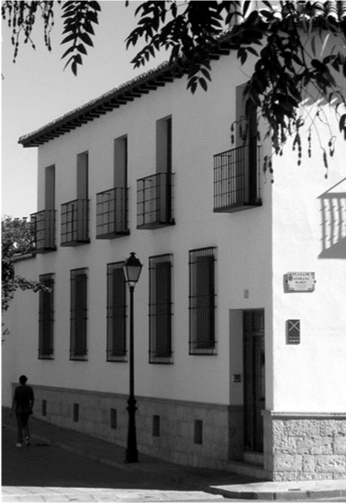
Fig. 19 Recently built house in Esquivias successfully drawing on local tradition
