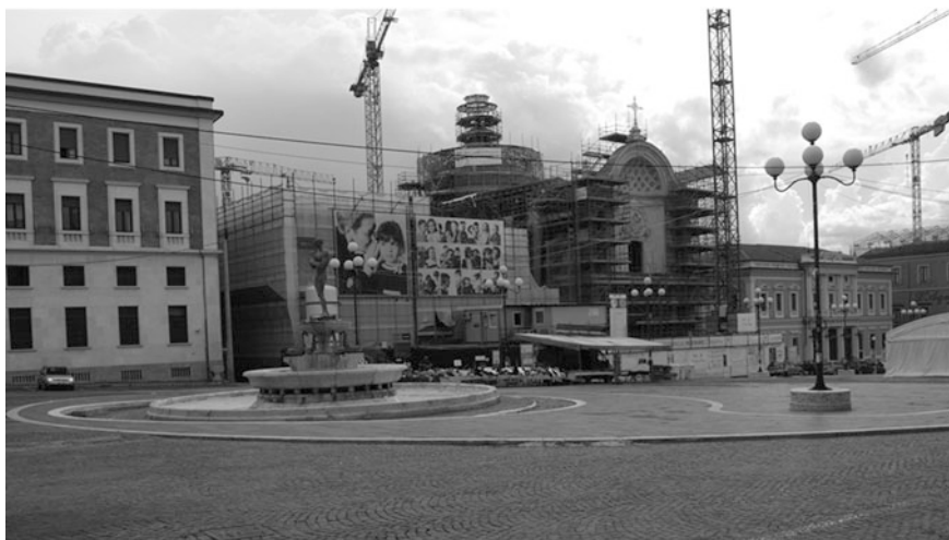
Fig. 1 Piazza Duomo in L’Aquila: the ongoing reconstruction process
