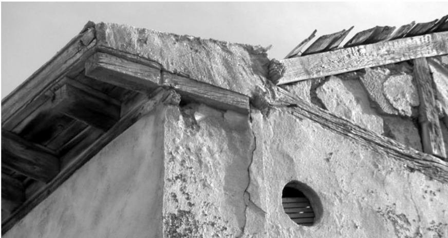
Fig. 10 Paired-corbels eave detail
