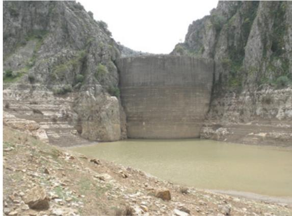
**Figure. 15** Lar Dam, Iran. One of the collapses induced by reservoir operation
