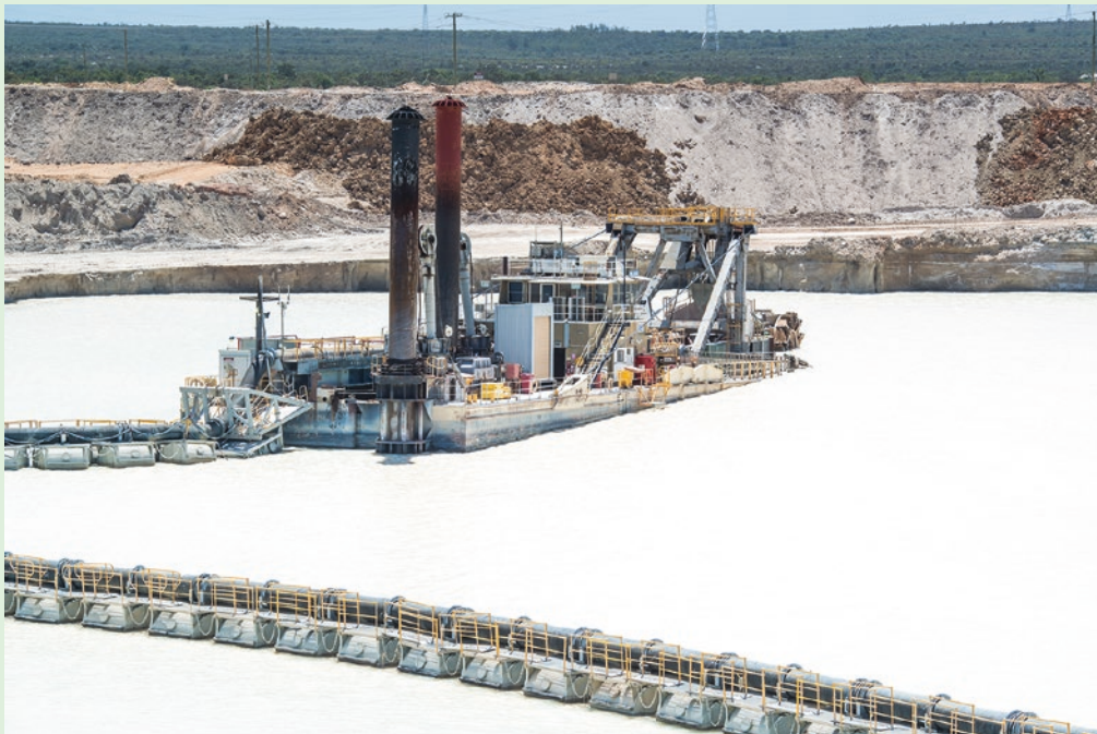
■ Fig. 5.38 Dredging operation (Image courtesy of Tronox)
