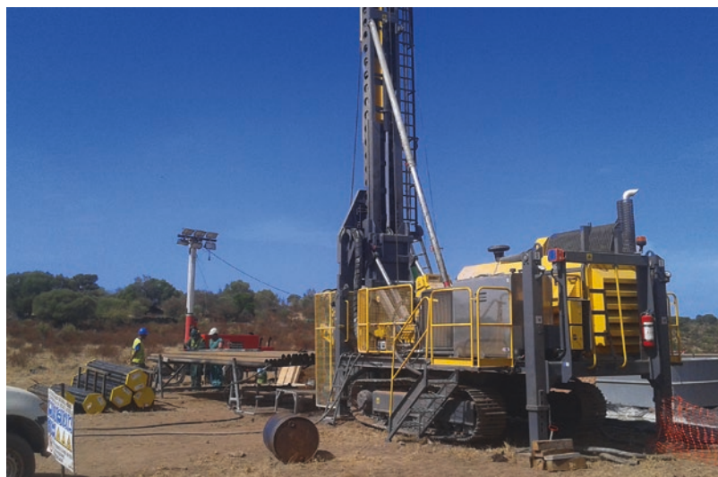
■ Fig. 3.55 Diamond core drilling operation (Image courtesy of Atlas Copco)
