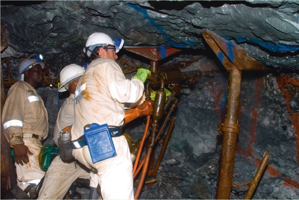
■ Fig. 5.69 Installing Split Sets (Image courtesy of AngloGold Ashanti)
