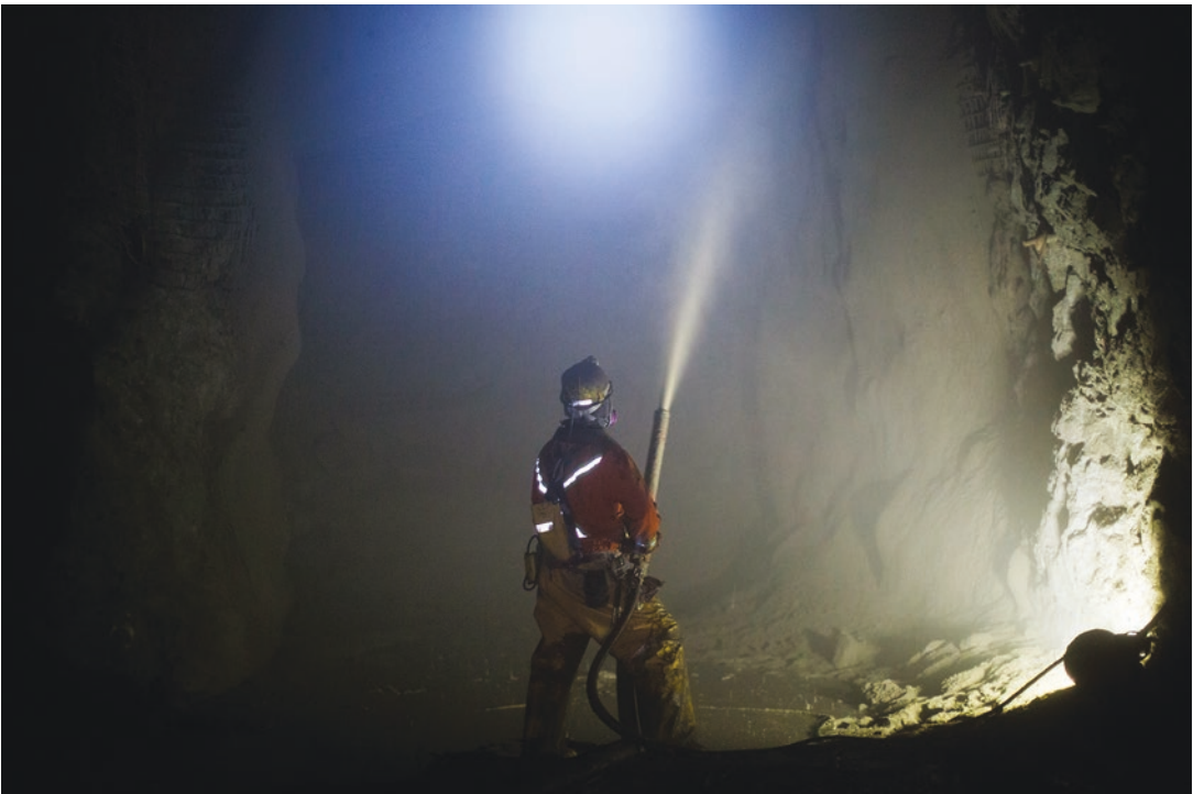
■ Fig. 5.56 Spraying shotcrete onto the walls of a drift underground at Snap Lake Mine (Canada) (Image courtesy of De Beers)
