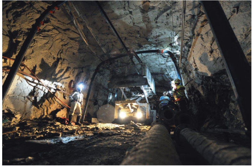
Fig. 1.14 Underground mining at Mponeng (South Africa) (Image courtesy of AngloGold Ashanti)
