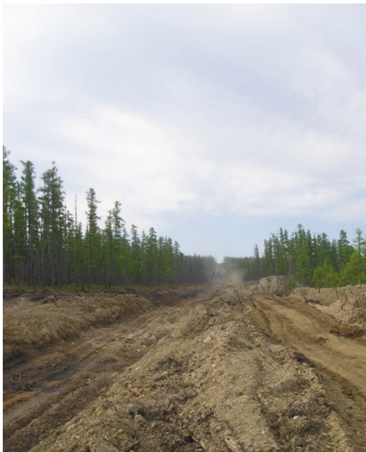
■ Fig. 4.11 Trenching in progress (Image courtesy of Petropavlovsk)
