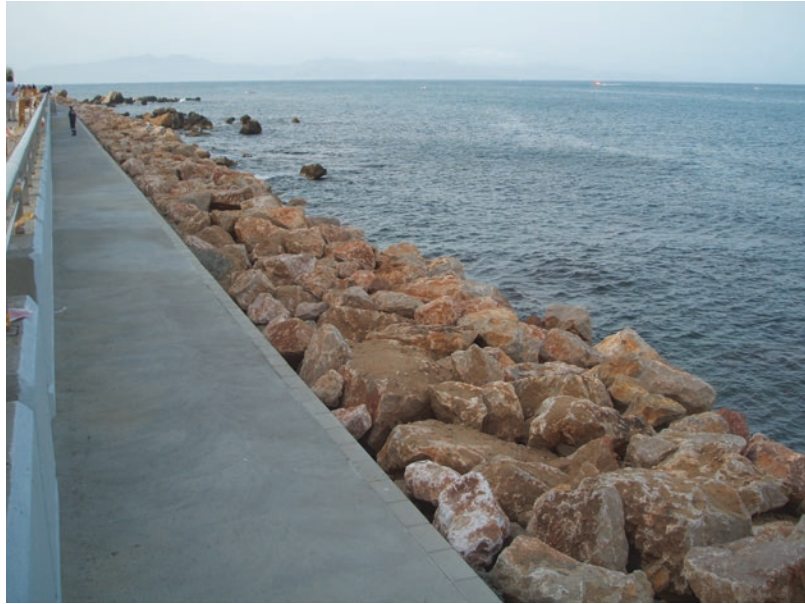
■ Fig. 2.28 Aggregates forming a breakwater or armour stone
