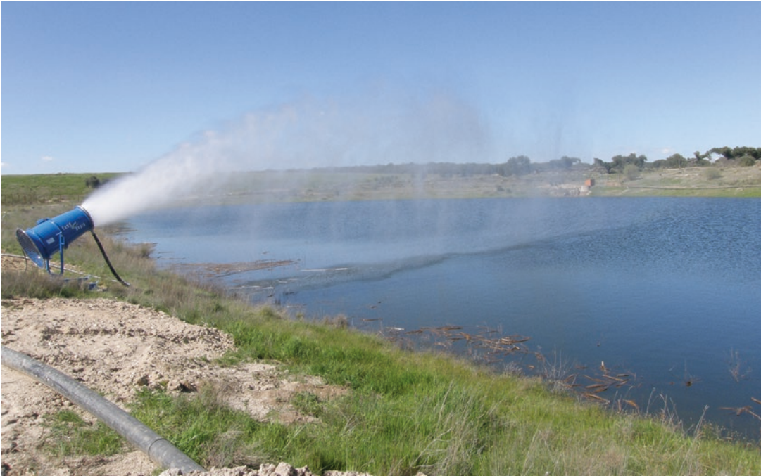
■ Fig. 7.51 Evaporation units (Image courtesy of ENUSA INDUSTRIAS AVANZADAS S.A.)
