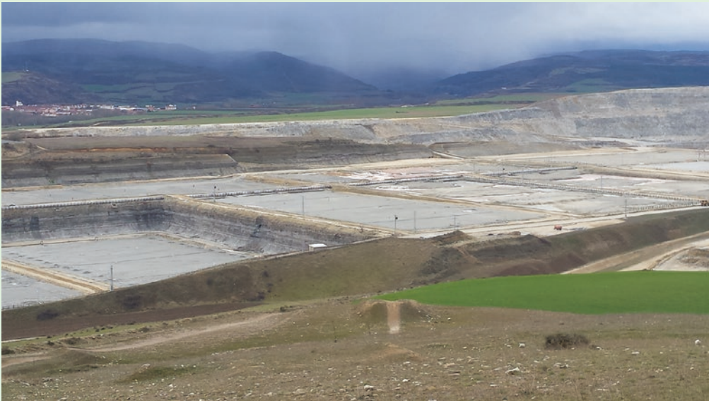
■ Fig. 5.40 General view of open-pit mine (Image courtesy of SAMCA)
