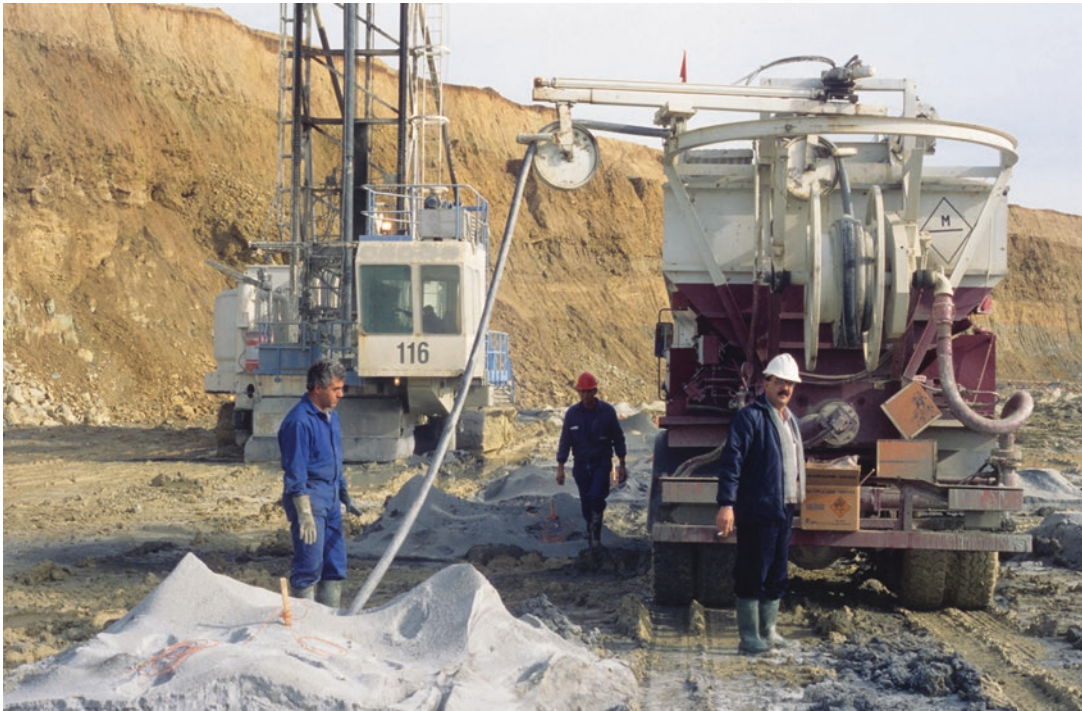
■ Fig. 5.75 Loading the borehole with explosive
