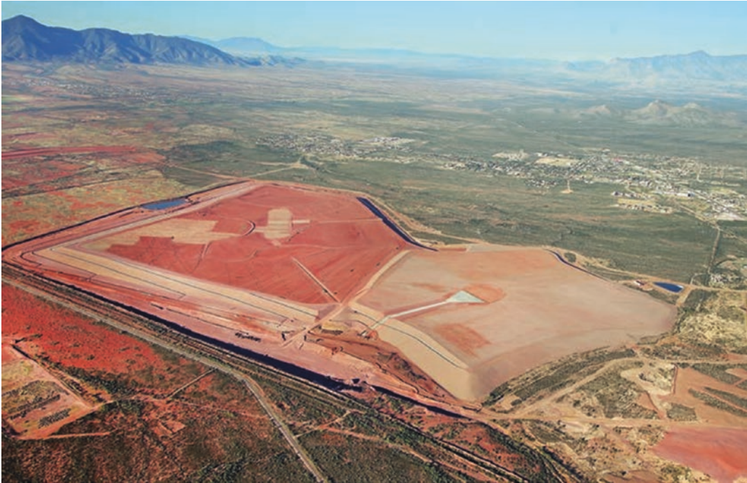
■ Fig. 7.48 Reclamation of North ( right ) and South ( left ) tailings impoundments as of 2013 (Image courtesy of FreePort-MacMoRan)
