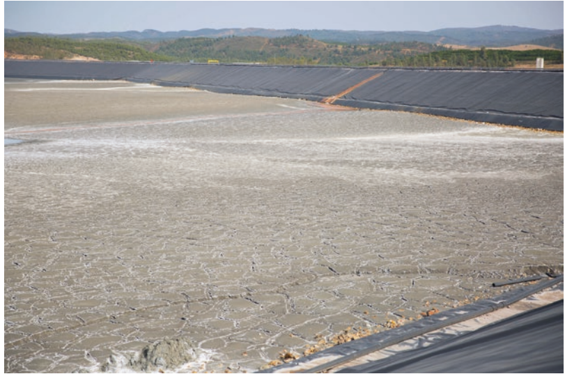
■ Fig. 6.96 Densified (dry stacking) tailings dam (Spain) (Image courtesy of Matsa, a Mubadala &Trafigura Company)
