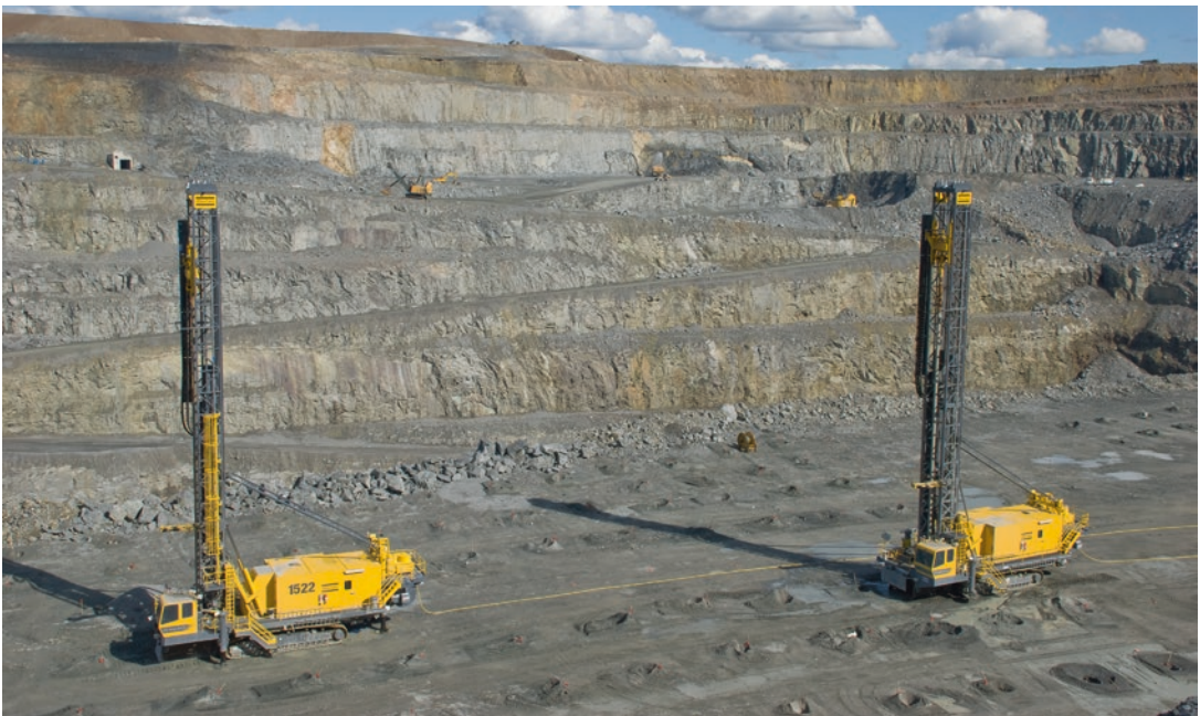
■ Fig. 5.76 High diameter rotary drills at Aitik mine (Sweden) (Image courtesy of Atlas Copco)
