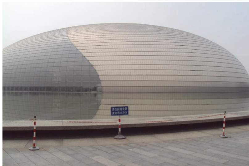
■ Fig. 1.25 Glass building (The National Grand Theater of China, Beijing)
