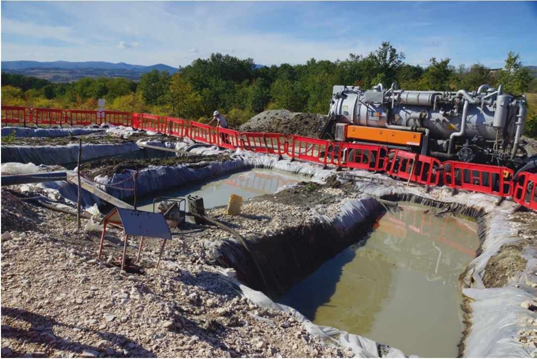
■ Fig. 3.56 Chemical products used with water in diamond core drilling (Image courtesy of AMC)
