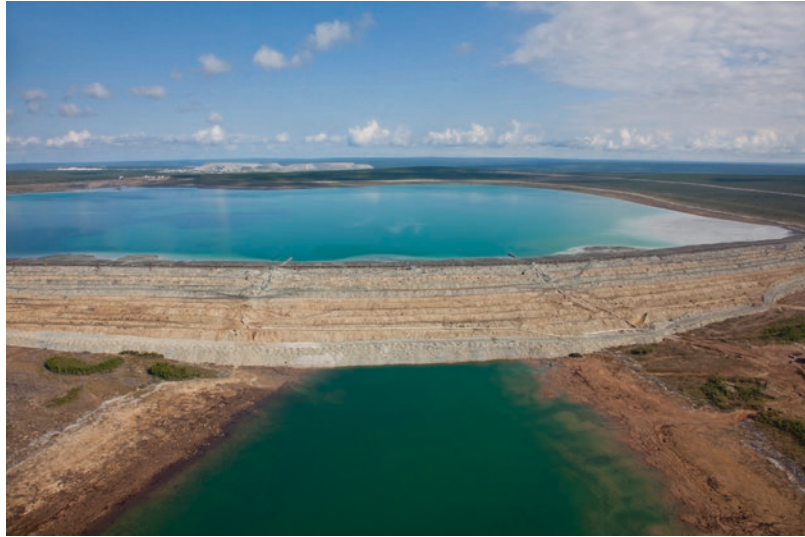
■ Fig. 6.93 Upstream tailings dam (Image courtesy of Alrosa)
