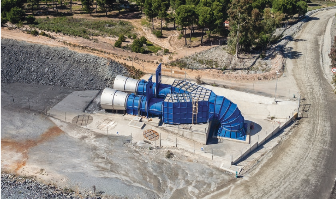
■ Fig. 5.49 Aerial view of ventilation equipment at Aguas Teñidas Mine (Spain) (Image courtesy of Matsa, a Mubadala and Trafigura Company)
