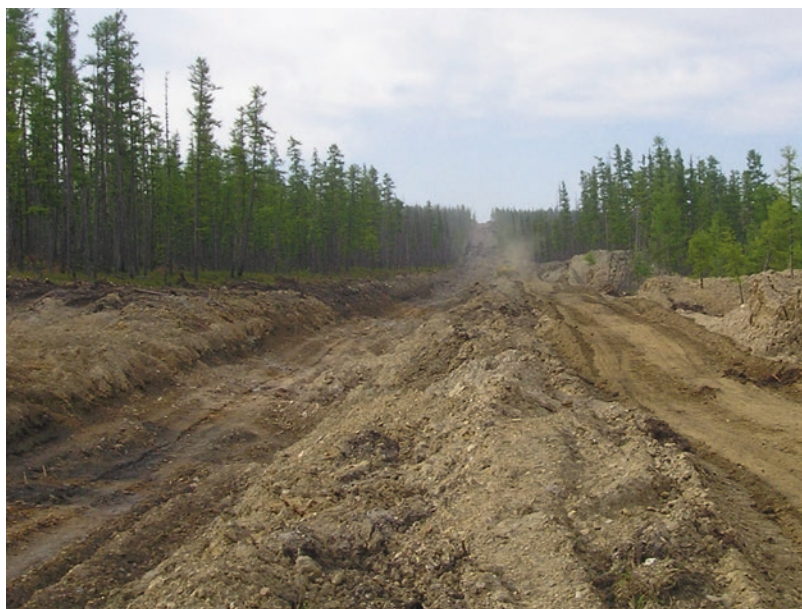
■ Fig. 3.5 Trenching in progress (Image courtesy of Petropavlovsk)
