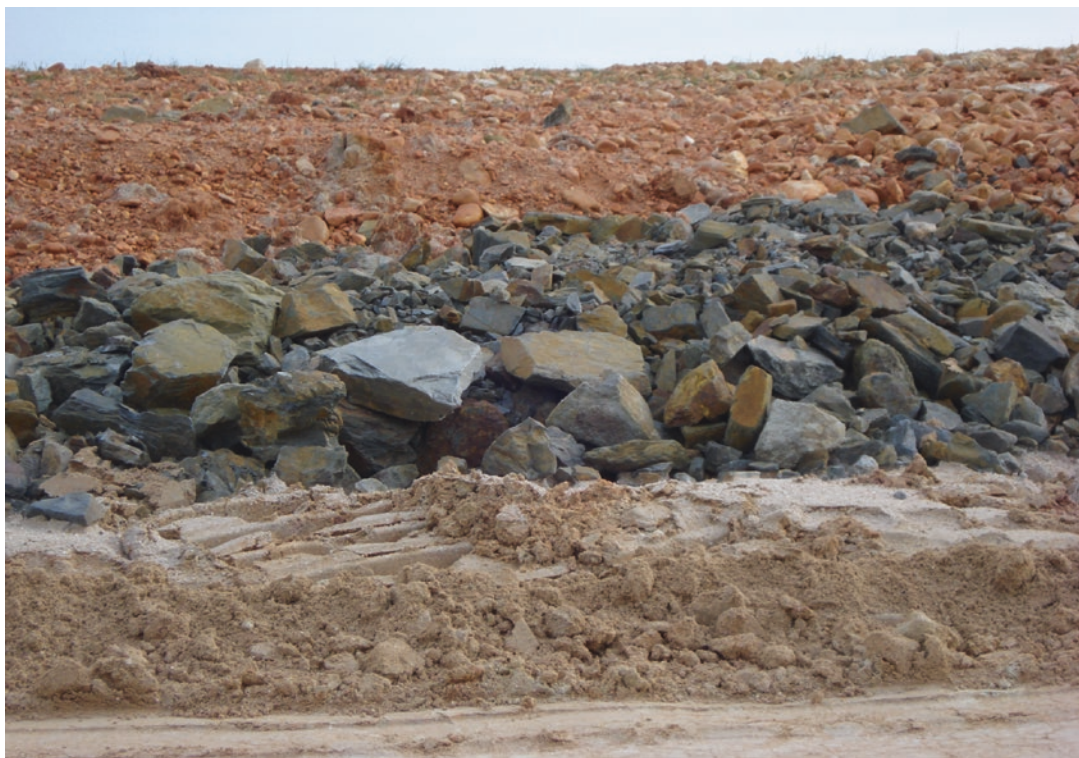
■ Fig. 7.49 Multilayer cover (Image courtesy of ENUSA INDUSTRIAS AVANZADAS S.A.)
