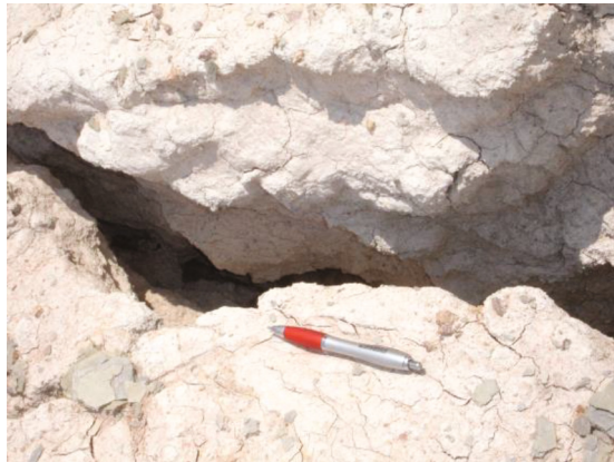
Fig. 9. Traction cracks on berm slope of cut 25.
