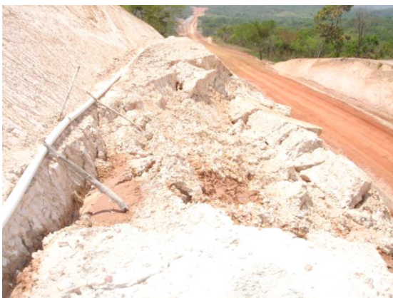
Fig. 12. Failure stretch in cut 25 slope.
