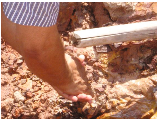
Fig. 11. Upwelling water in cut 25 slope.
