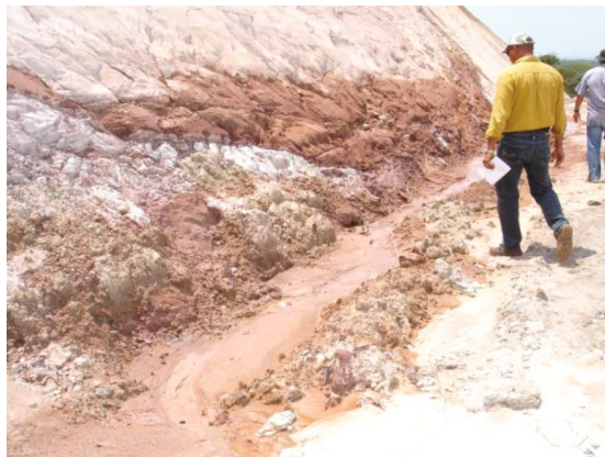
Fig. 10. Saturation from the slope basis in cut 25.
