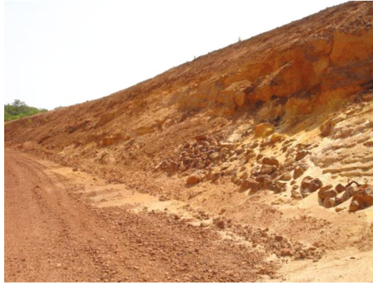
Fig. 2. General view of part of cut 16 with superficial erosion.
