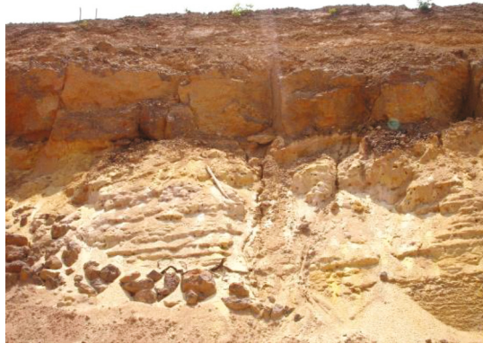
Fig. 3. General view of part of the cut 16 with superficial erosion.
