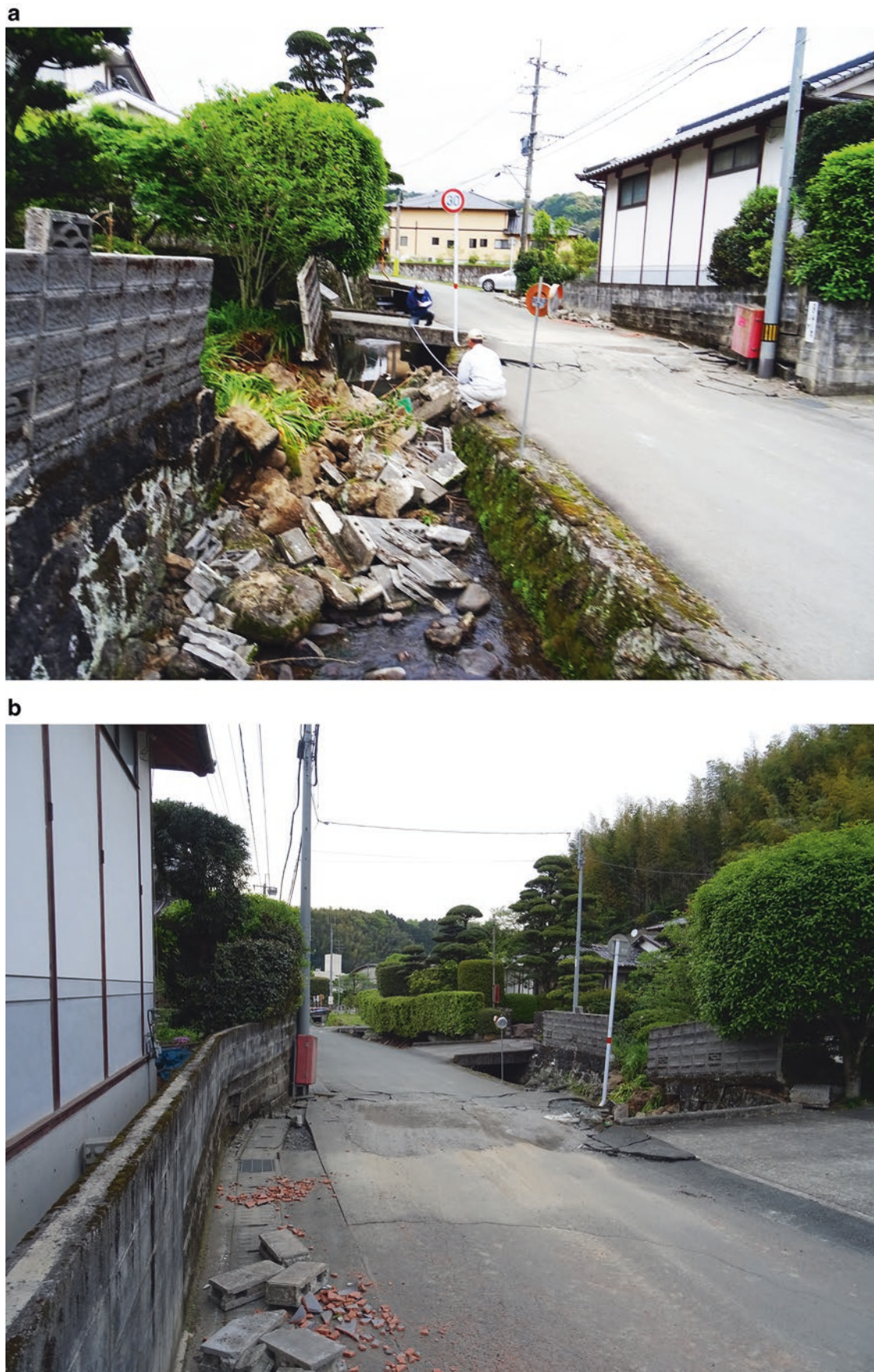
Fig. 10 Right-lateral offsets of a road, ditch, and fence wall. (a–c) Dextral offset ~1.3 m of the ditch (a), road (b), and wall fence (c–d)
