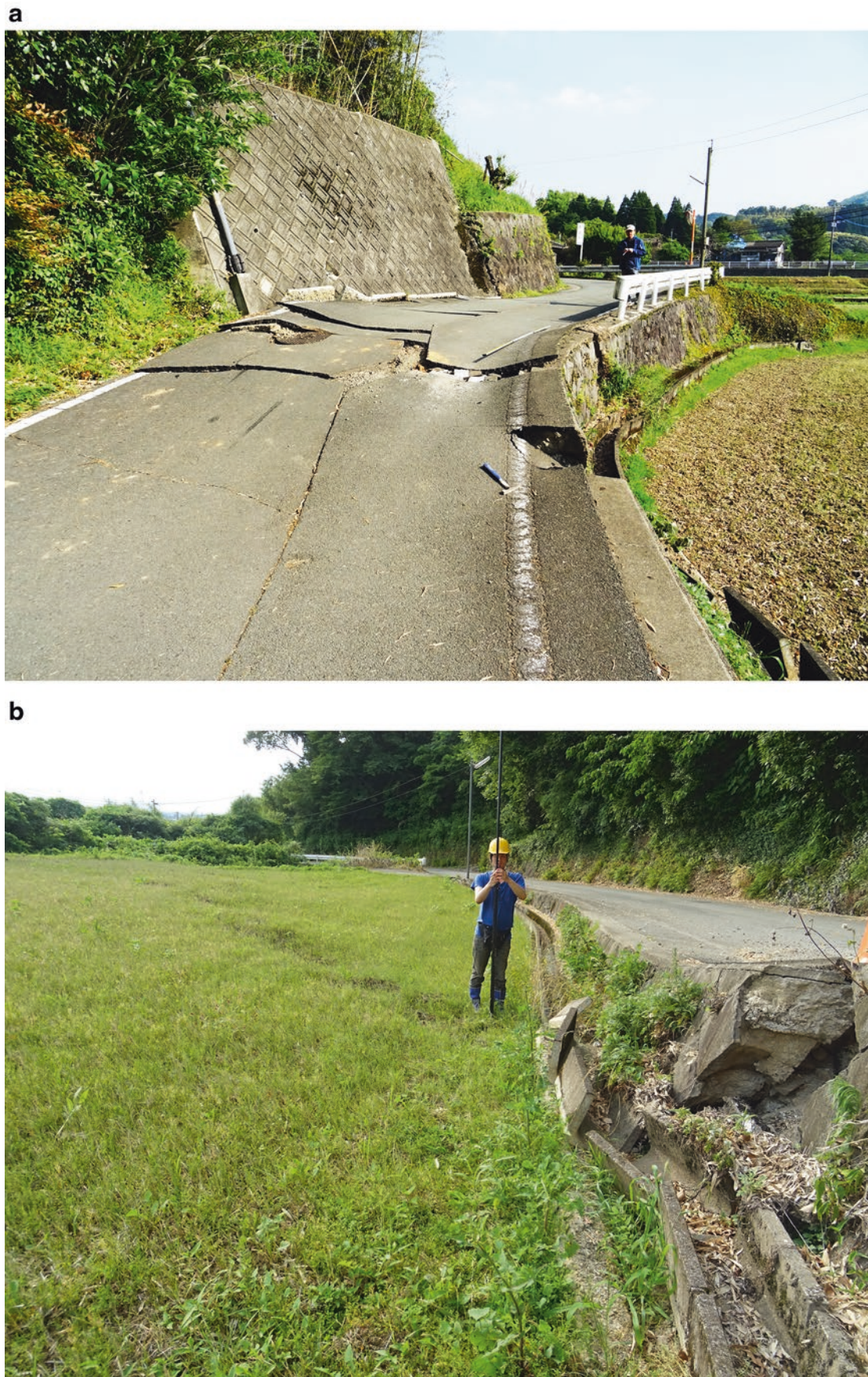
Fig. 23 Strike-slip offset of a road and field paths. (a, b) Left-lateral offset of a road and field. (c) Left-lateral offset of a field path (offset \sim 0.3 m). (d) Right-lateral offset of a field path (offset \sim 0.4 m)
