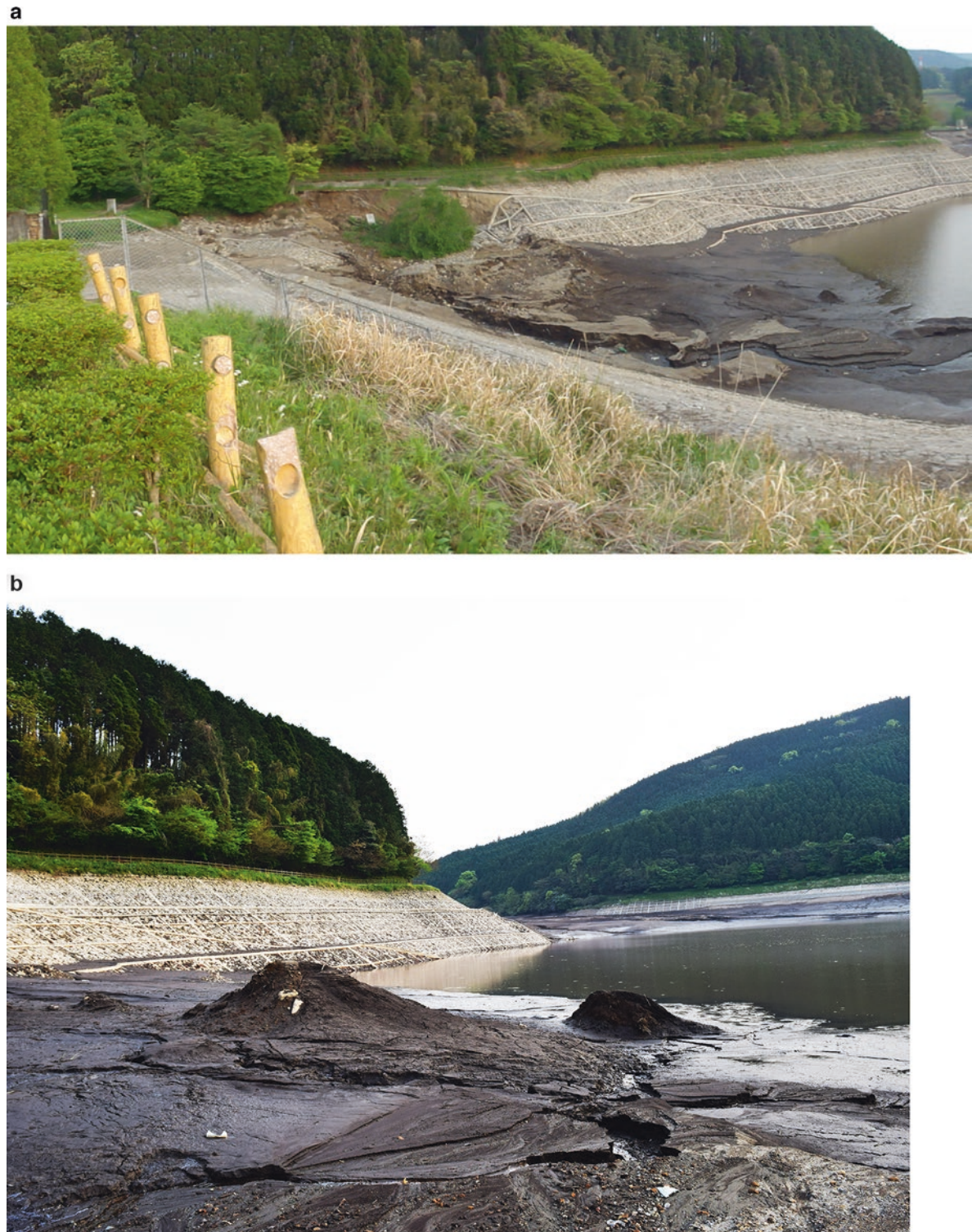
Fig. 29 Earthquake-induced liquefaction that occurred inside a dam. (a) Overview of the Okirihata dam that was damaged by the coseismic surface rupture zone. (b, c) Sand boils occurred inside the dam
