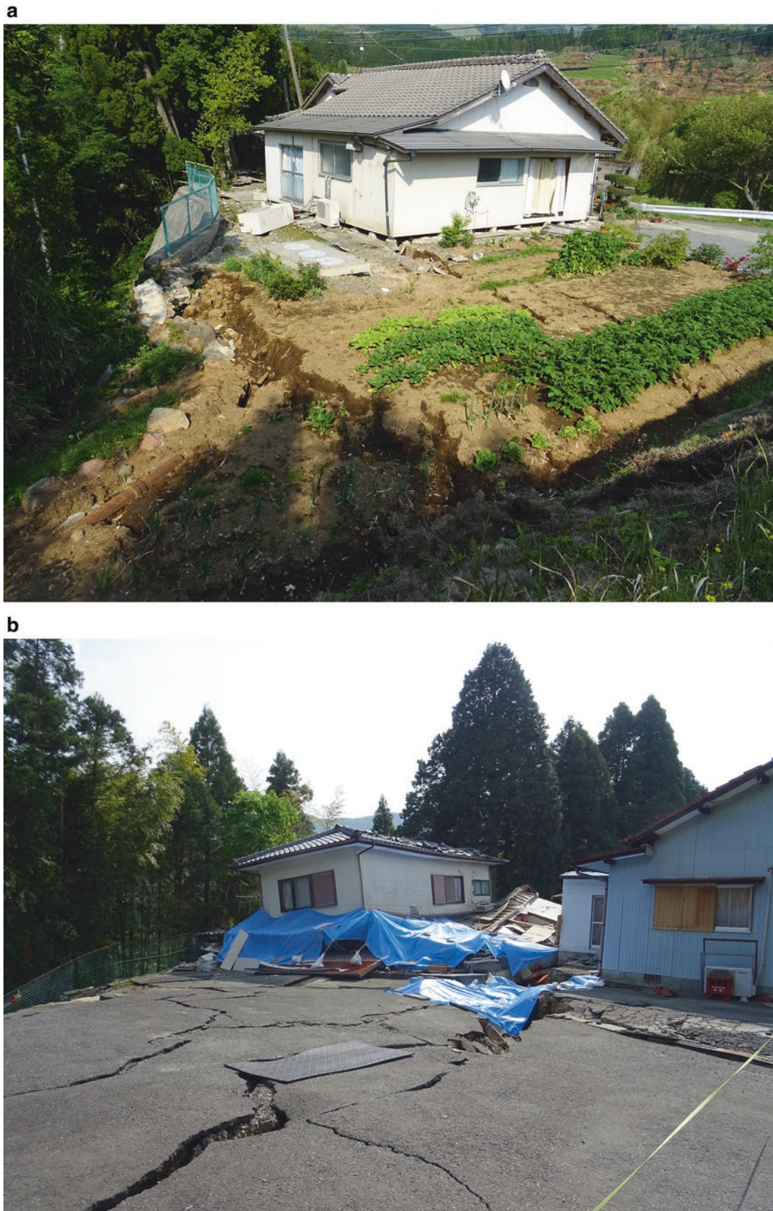
Fig. 72 Houses damaged on the coseismic surface ruptures. (a–c) Houses damaged on the coseismic surface ruptures. (d) Judgment card of dangerous house that cannot be inhabited again
