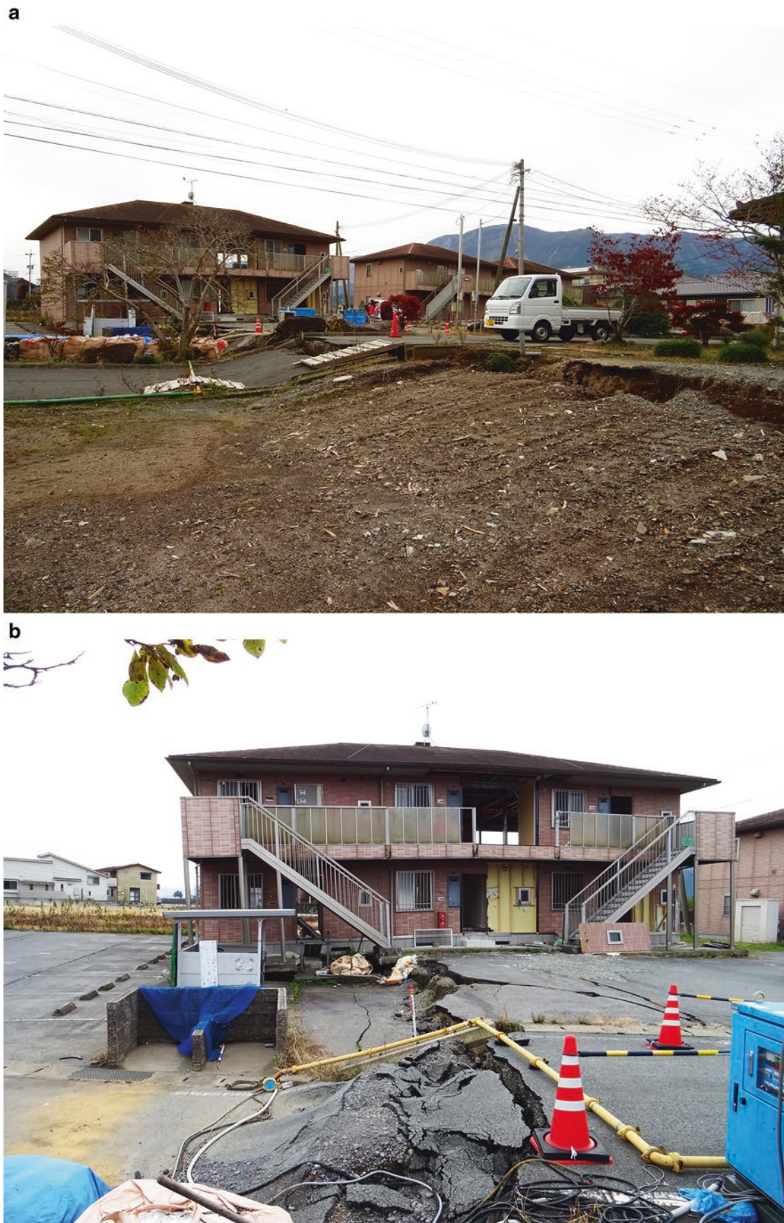
Fig. 76 Damaged houses on a coseismic normal fault scarp. (a) A damaged house located on a coseismic normal fault scarp. (b) Close-up view of (a). (c) A house inclined to a coseismic normal fault scarp,
