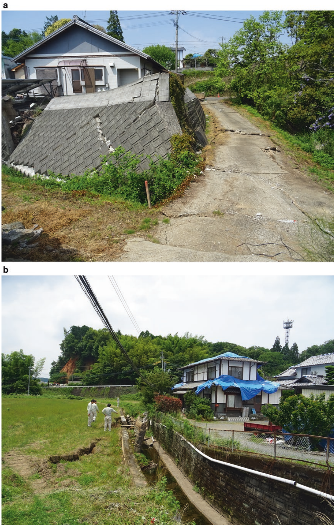
Fig. 71 Houses damaged and collapsed along the coseismic surface ruptures. (a, b) House damaged on the coseismic surface ruptures. (c)
