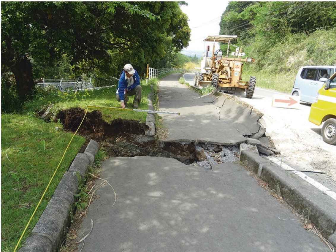
Fig. 13 Right-lateral offset of roads. (a) Coseismic surface ruptures cut a road at Okirihata dam site. Dextral offset ~1.3 m (b), ~0.8 m (c) and 0.5 m (d)
