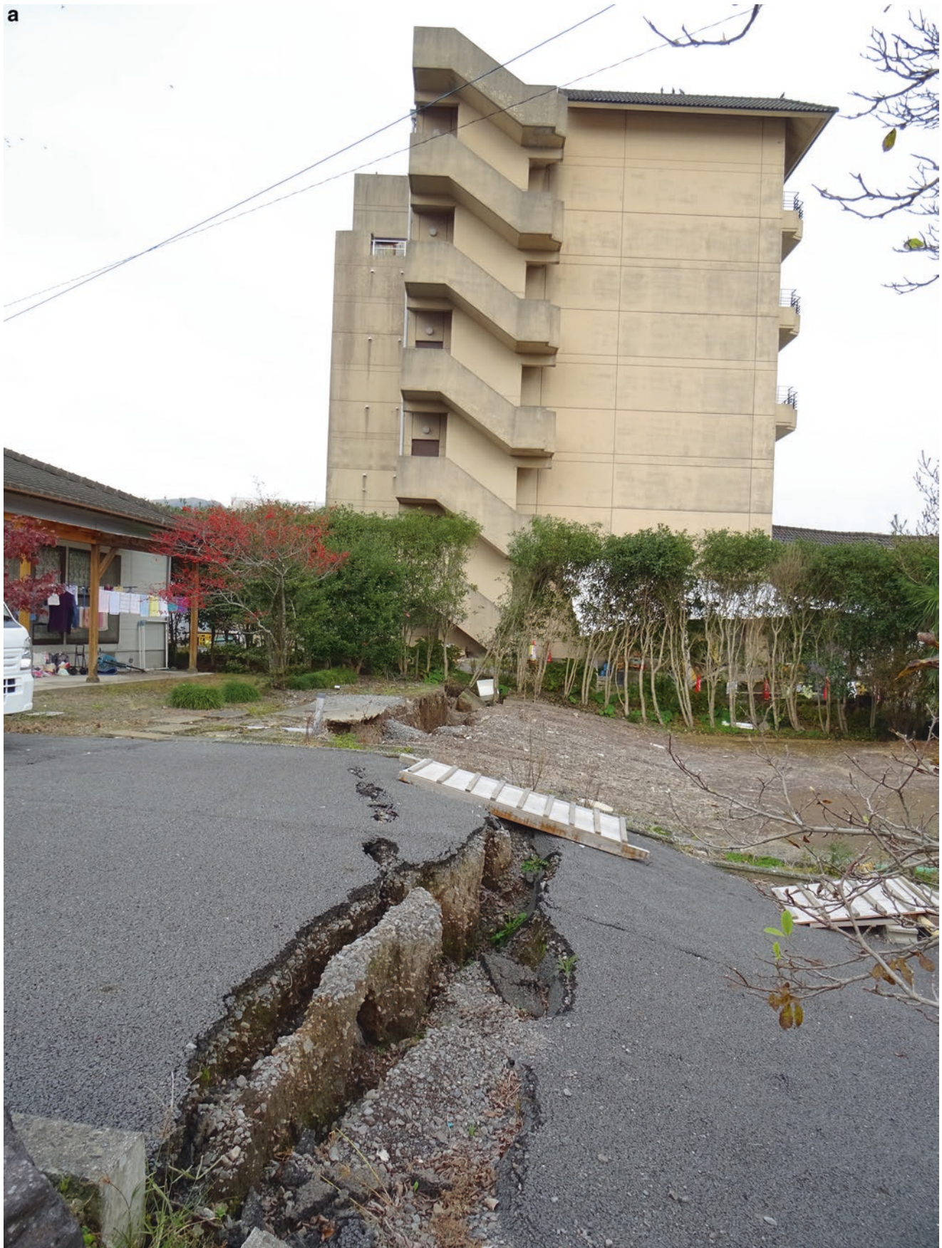
Fig. 77 Damaged building on a coseismic normal fault scarp. (a) A building on a coseismic normal fault scarp. (b) The building shown in (a) was uplifted \sim 0.5 \sim 0.7 m on a coseismic normal fault scarp (right side uplift). (c) Coseismic cracks occurred on a wall of building shown in (a, b)
