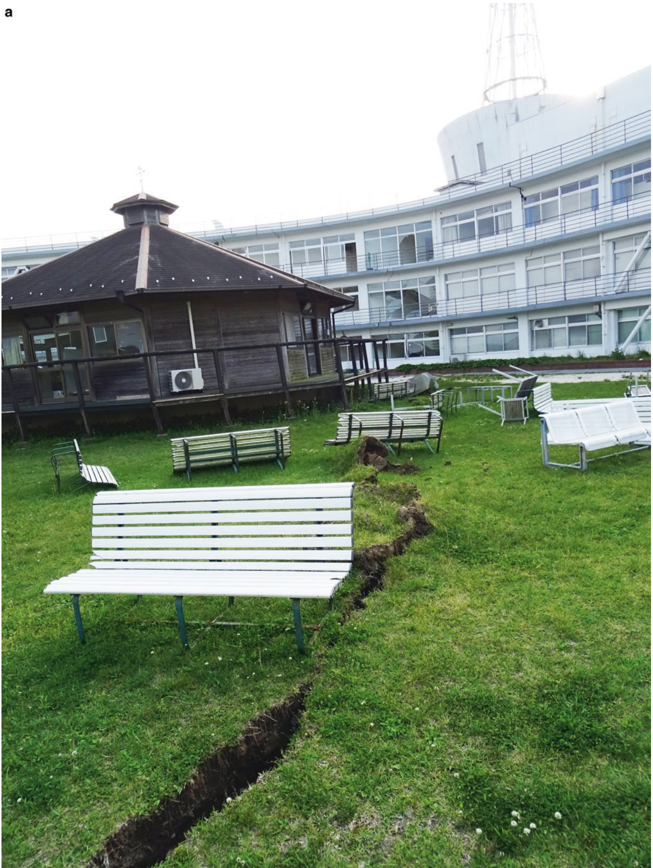
Fig. 73 Coseismic surface ruptures and damaged building of Tokai University at the Kumamoto Aso campus. (a) Coseismic surface ruptures occurred in a schoolyard throughout the base of the building. (b)
