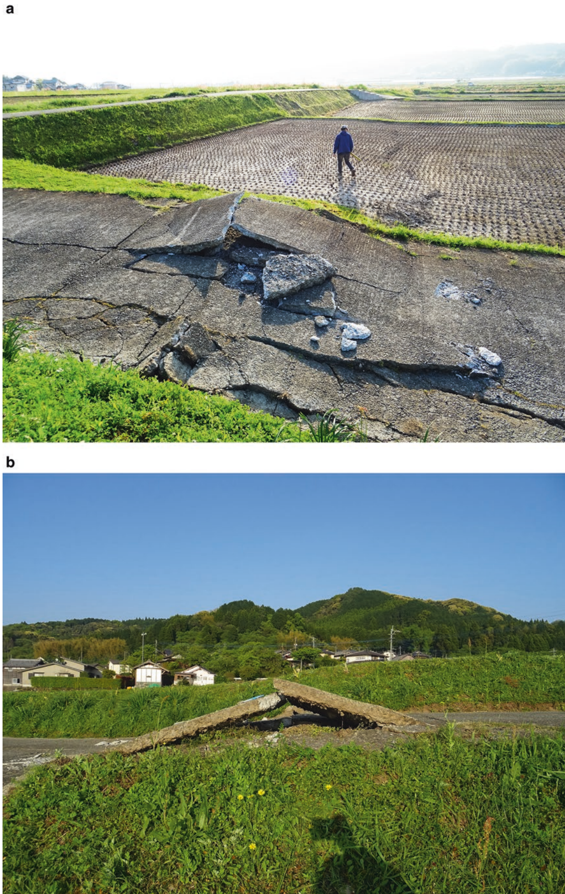
Fig. 27 Mole track structures occurred at roads. (a, b) Mole track along the WNW–ESE-striking coseismic surface rupture zone. (c, d) Mole track occurred on a road along the ENE–WSW-striking coseismic surface rupture zone
