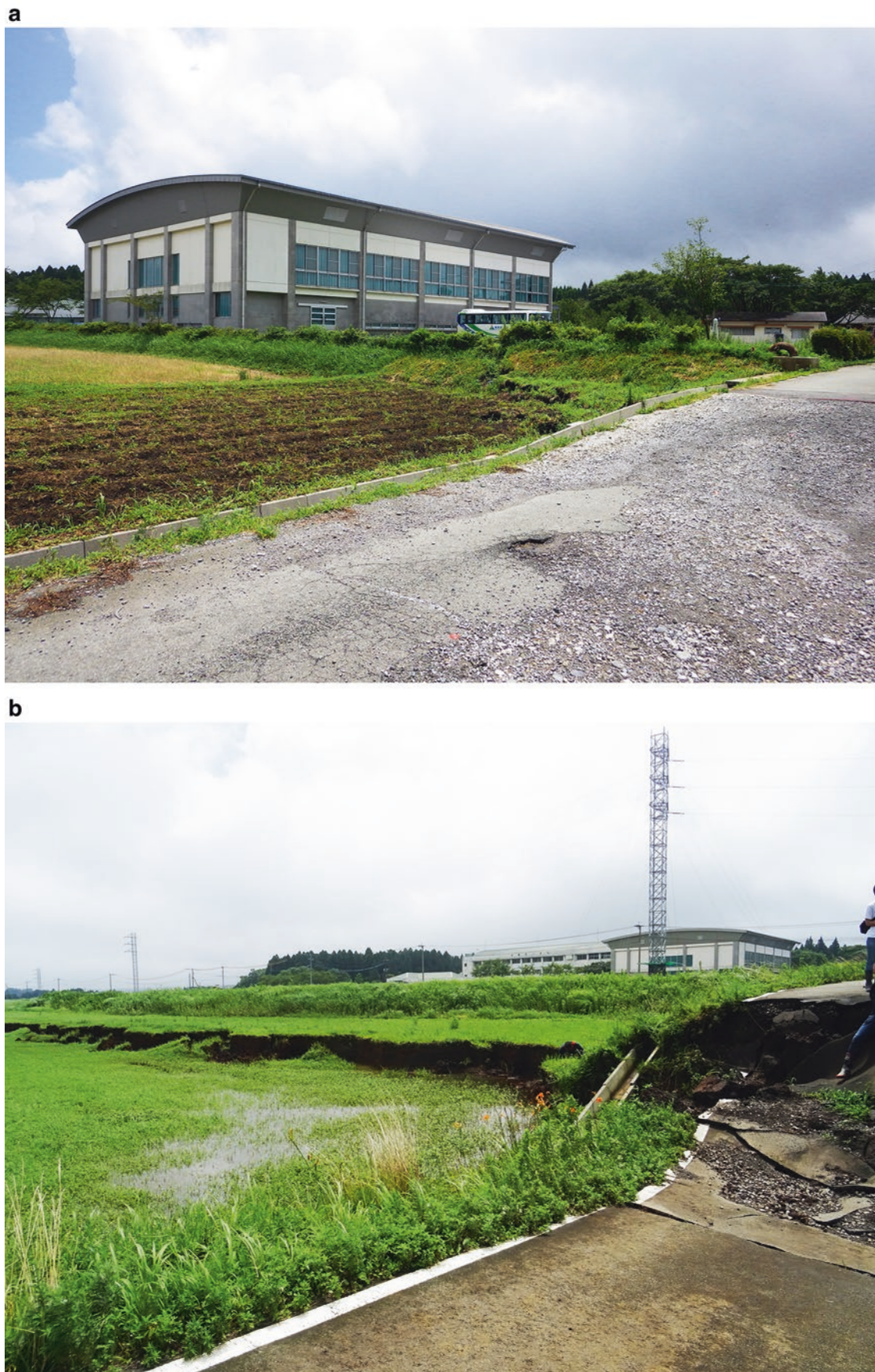
Fig. 74 Coseismic surface ruptures and damaged school house in a site near the Aso Nishi primary school. (a) Coseismic surface ruptures crosscut a road and fields (right side uplift ~50 cm). (b) A continuous
