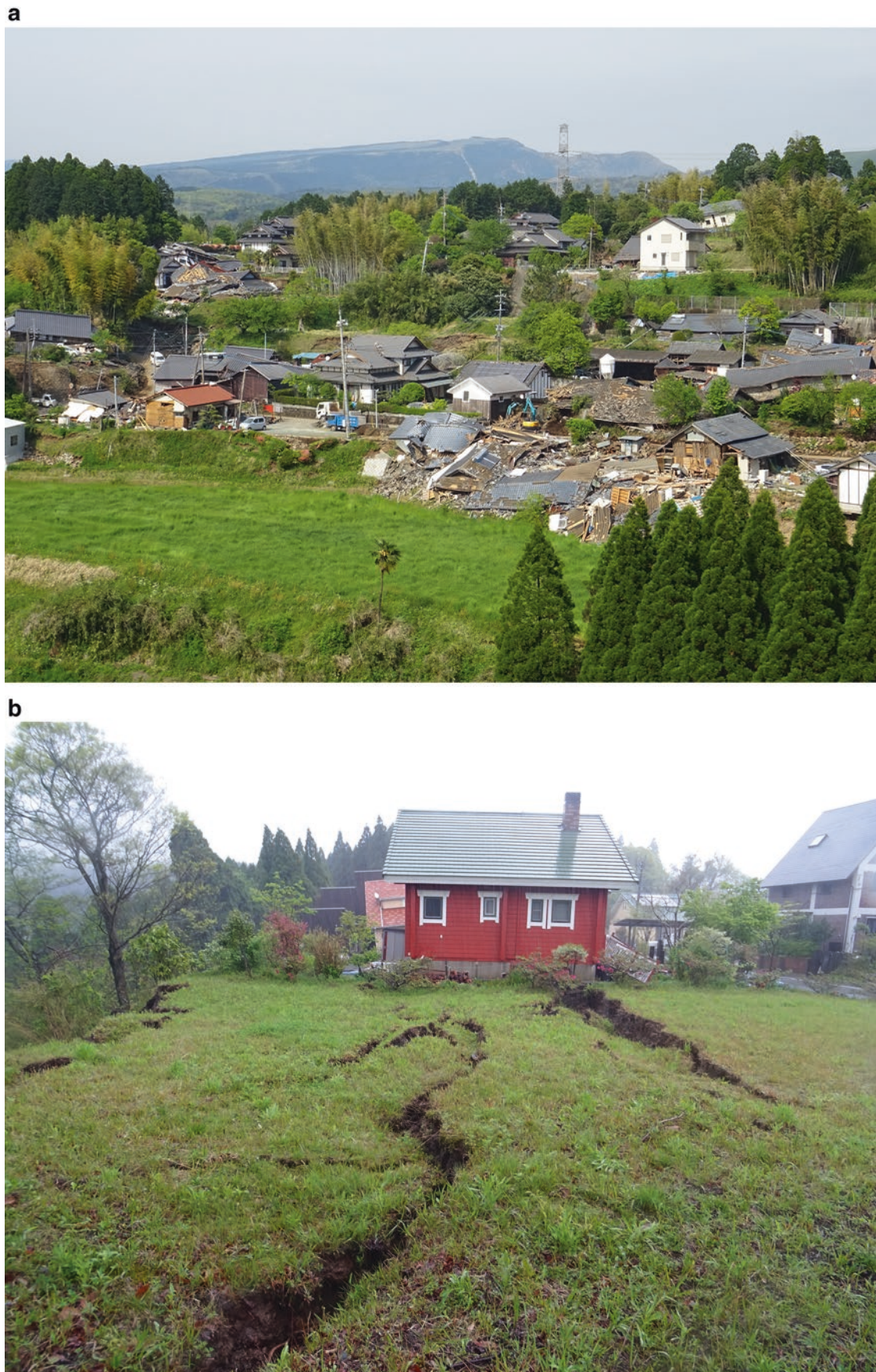
Fig. 70 Houses collapsed along a coseismic surface rupture zone. (a) Houses collapsed along the coseismic surface ruptures along a preexisting fault scarp of the Futagawa fault. (b–d) Houses collapsed and slanted along the coseismic surface ruptures
