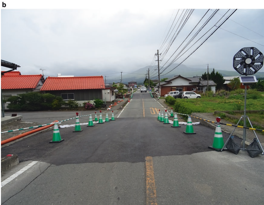
Fig. 75 Houses damaged along a coseismic graben. (a) Google image (acquired on 16 April 2016) showing a coseismic graben structure in which the houses and roads were damaged. (b, c) Ground subsidence inside a graben structure (the road was repaired immediately after the
