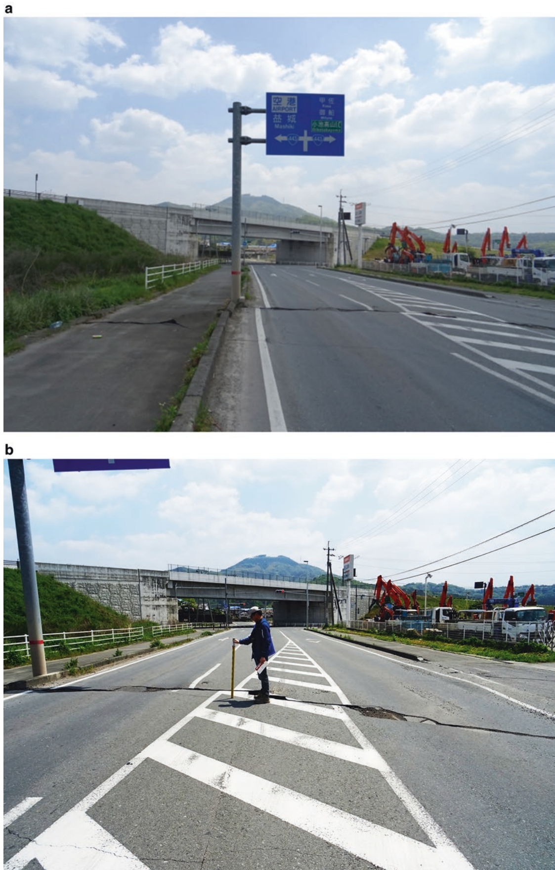
Fig. 7 Right-lateral offset of a road. (b, c) Close-up view of (a) (offset ~0.3 m)
