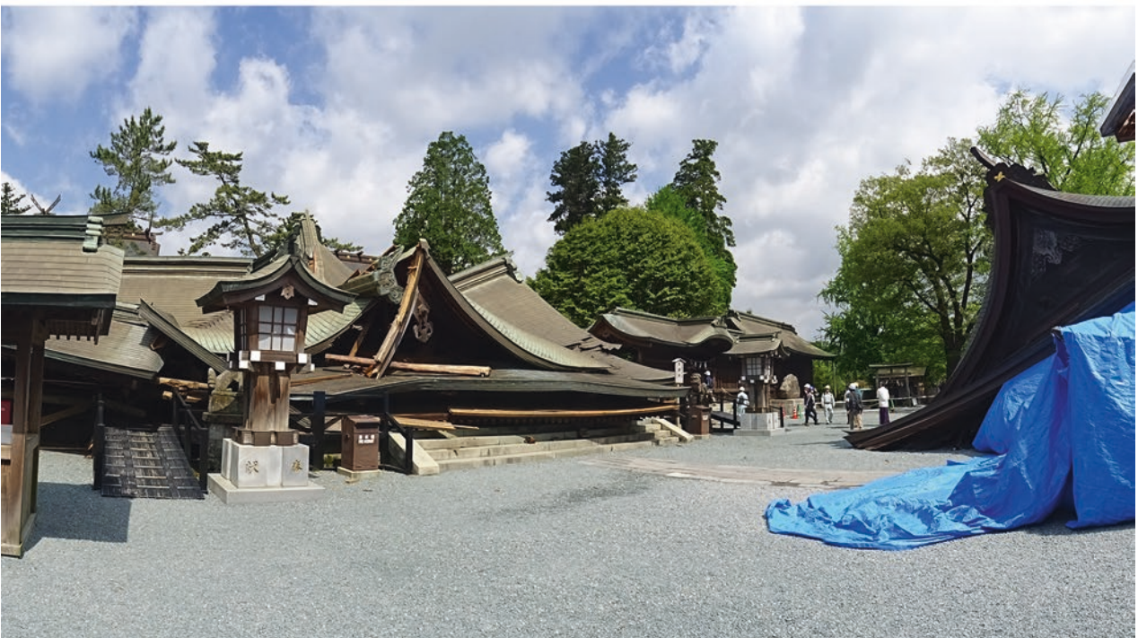
Fig. 78 Damaged shrines and landslides. (a) Collapsed stone lanterns in the Hebi-ishi ( means slake stone) shrine. (b) Collapsed Aso Shrine located in the northeastern end area of the coseismic surface rupture
