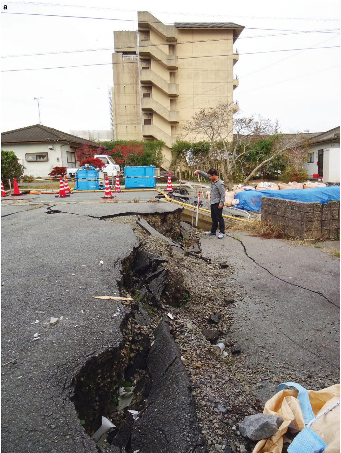
Figure Plate 4 Damaged building (a) and house (b) on the same coseismic fault scarp (vertical offset \sim 0.7 m)
