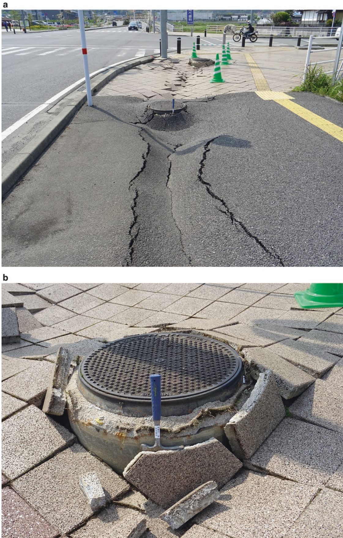
Fig. 31 Ground subsidence caused by earthquake-induced liquefaction. (a) Manhole uplift along the extensional crack. (b) Close-up view of (a)
