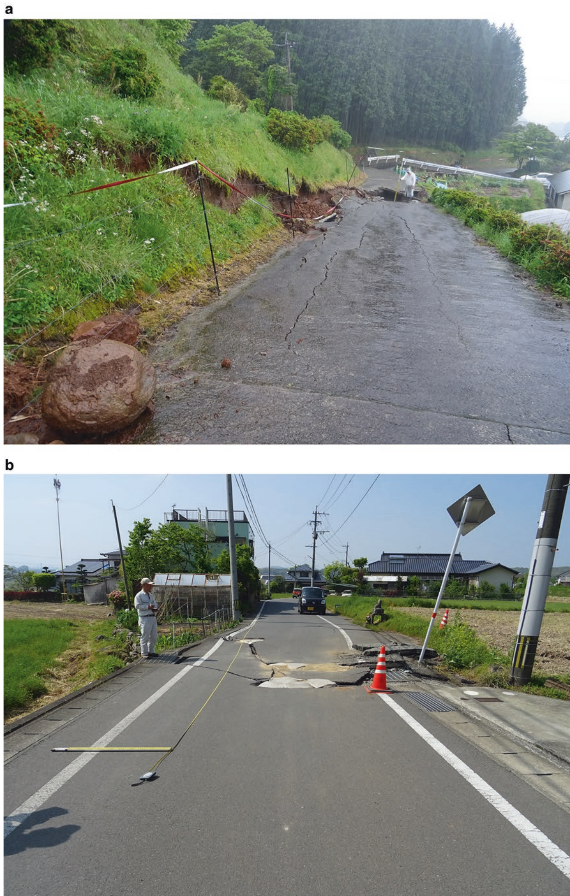
Fig. 14 Right-lateral offset of roads and slope. (a) Offset ~0.5 m, (b) 0.8.m, (c, d) 0.7.m
