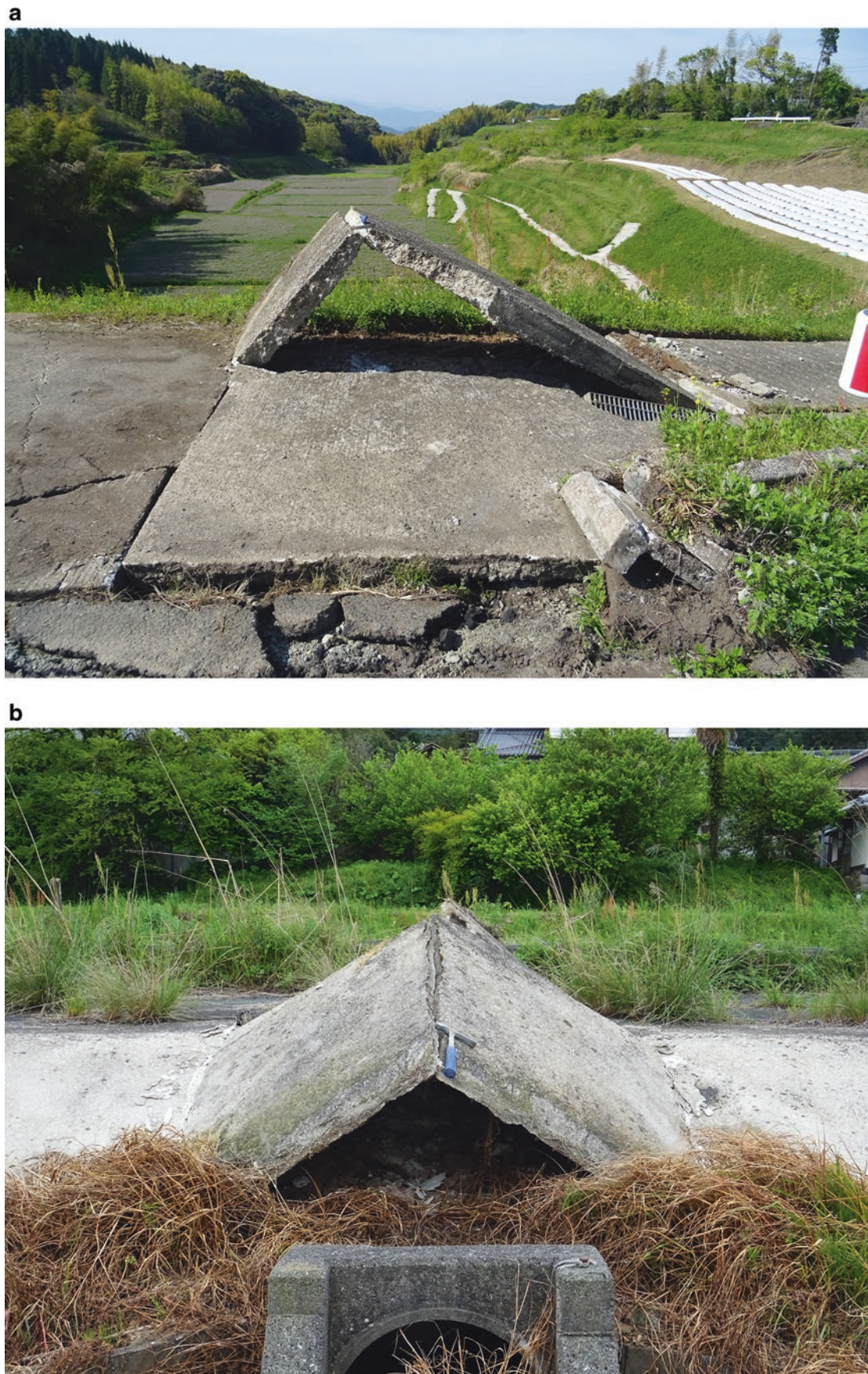
Fig. 28 Mole track structures occurred at a road and field path. (a–c) Mole track structure occurred at a road. (d) Mole track structure occurred at a field path along the ENE–WSW-striking coseismic surface rupture zone
