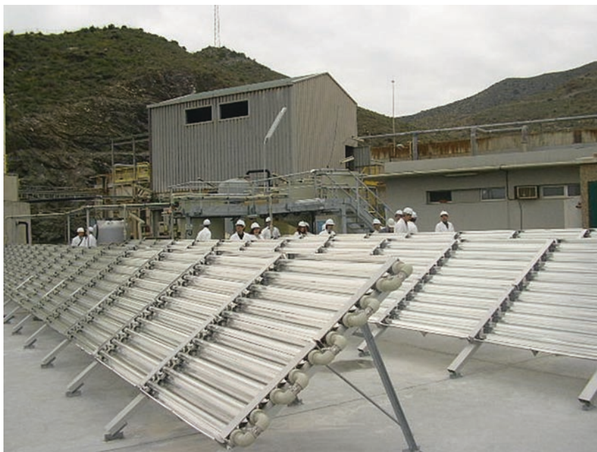
Fig. 21.3 Views of the solar collector field of the hybrid solar photocatalytic-biological plant developed in CADOX Project ( http://www.psa.es/webeng/projects/cadox )
