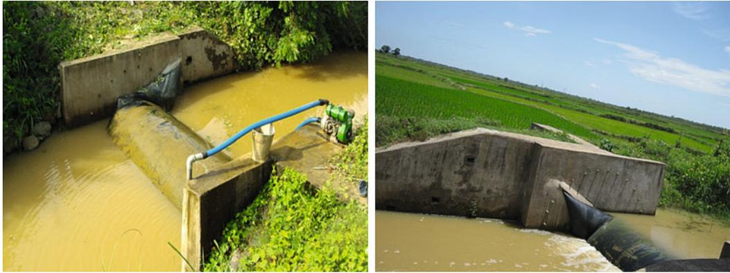
**Plate 1** Rubber dams installed in watersheds of Odisha by DWM, Bhubaneswar
