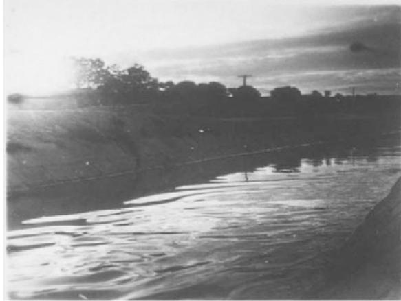
**Fig. 6.55** A hyperconcentrated flood in the North Luohe River is diverted into an irrigation canal and transported for over 50 km without serious sediment deposition
