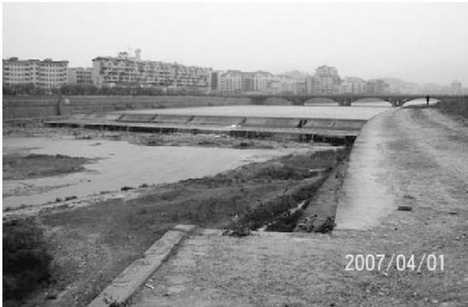
**Fig. 10.33** Riparian forest has been replaced by buildings and the banks are hardened with concrete in Guangyuan, Sichuan
