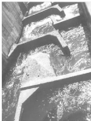
**Fig. 10.59** Fish ladder on the Bonneville Dam on the Columbia River. More than 1 million salmon swim through the fish ladder to pass the dam to upstream spawning grounds every year.
