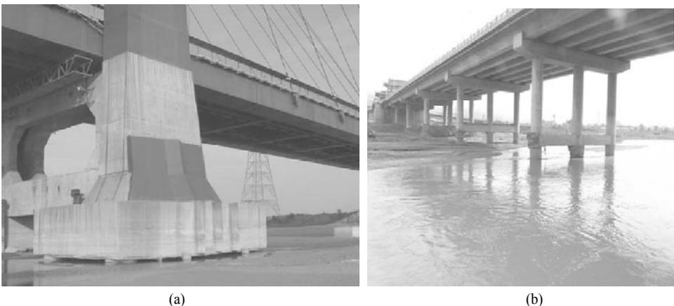
**Fig. 3.45** (a) Exposed bridge piles on the lower Yellow River due to release of clear water from the Xiaolangdi Reservoir eroding the channel bed; (b) A buried part of the bridge piers is exposed due to incision on the Weihe River at Baoji
