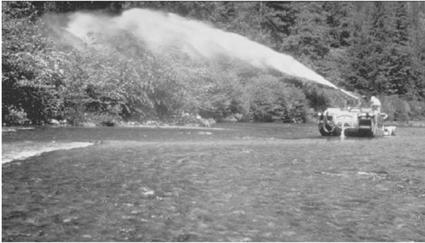
**Fig. 10.58** Hydroseeding of a streambank for restoration of understory riparian vegetation. Special tank trucks carrying seed, water, and fertilizer are used in the revegetation efforts (after FISRWG, 1997)
