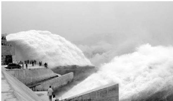
Fig. 6.17 Artificial flood created by releasing water from the Xiaolangdi Reservoir on July 04, 2002. Water was released from different elevations to control the sediment concentration. The released concentration from the bottom outlet is high dyeing the water yellow and red, and the water from the top outlet is clean and white
