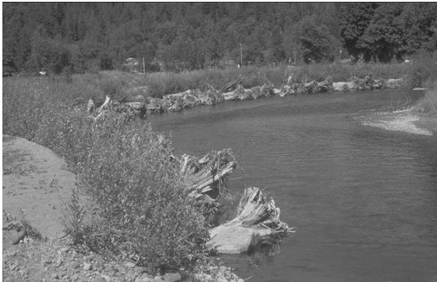
**Fig. 10.54** The protruding rootwads effectively reduce flow velocities at the toe (after FISRWG, 1997)
