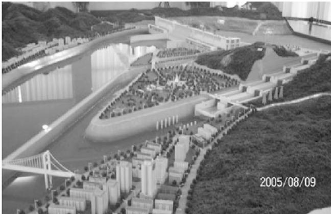
**Fig. 7.34** A model of the Three Gorges project on the Yangtze River- from right to left: five step ship locks including the upper and lower approach channels, the ship lift and its channel, the left power house, the spillway, and the right power house (See color figure at the end of this book)
