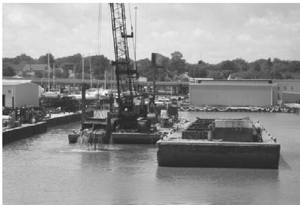
**Fig. 9.24** Environmental clamshell dredge removing PCB contaminated sediment from the Kinnickinnic River Great Lakes Legacy Act Cleanup in Milwaukee, U.S. and preparing to place it in a collection barge (photo provided by Dr. Xiaochun Zhang, Wisconsin Department of Natural Resources) (See color figure at the end of this book)
