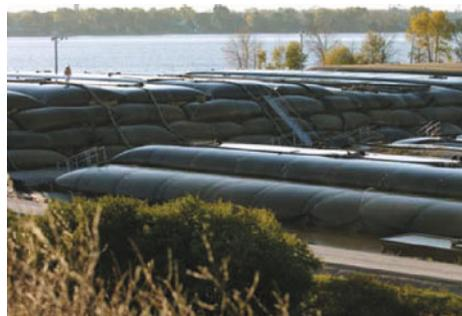
**Fig. 9.25** Geotextile tubes being filled by dredged sediment and water (left) and stack of geotextile tubes dewatering (right) at the Little Lake Butte des Morts project of the Fox River, Wisconsin, U.S. (photos provided by Steven Laszewski)
