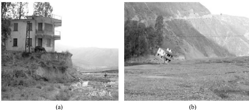
**Fig. 4.54** (a) Aggradation of the debris flow channel endangered the original observation tower on the Jiangjia Ravine in 2006; and (b) The tower fell into the ravine due to direct assault of flow at the tower base in 2009
