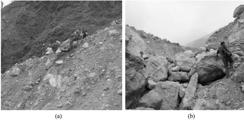
**Fig. 11.63** An artificial step-pool system was constructed in June 2009 for stabilization of the new drainage system on the Wenjiagou Landslide: (a) Large stones with diameters larger than 1 m were removed from the banks of the new gully for construction of steps; (b) Large stones were placed together to form the artificial steps. (See color figure at the end of this book)
