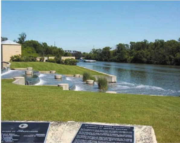
**Fig. 9.16** Sidestream Elevated Pool Aeration station number 5 discharging aerated water back to the Calumet-Sag Channel
