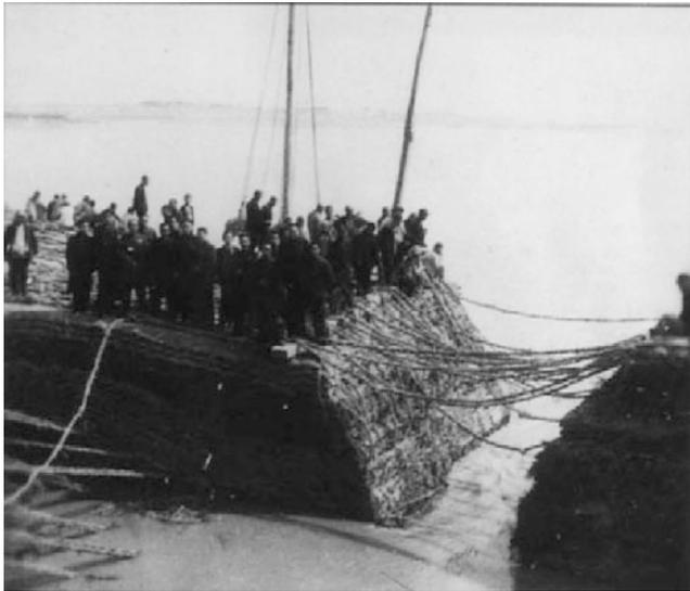
**Fig. 6.7** The breached south levee of the Yellow River was finally closed in 1946, which ended the 8 years of flooding of Yellow River water over the central China plain. (after YRCC, 2001)
