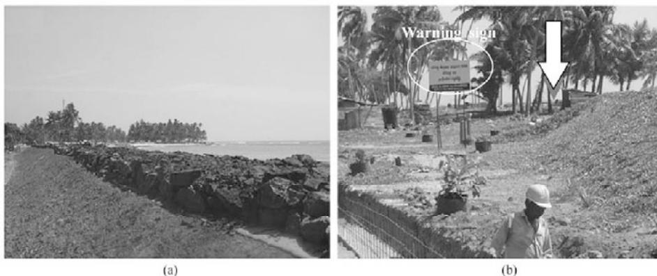
**Fig. 8.74** (a) Post-tsunami reconstruction of beach defenses in Sri Lanka; (b) at the edge of a beach defense is an open area (arrow) that creates conditions for a low resistance path for water in case of a surge. (from Fernando, et al. 2008)
