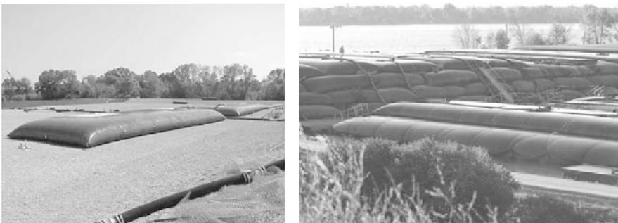
**Fig. 9.25** Geotextile tubes being filled by dredged sediment and water (left) and stack of geotextile tubes dewatering (right) at the Little Lake Butte des Morts project of the Fox River, Wisconsin, U.S. (photos provided by Steven Laszewski) (See color figure at the end of this book)
