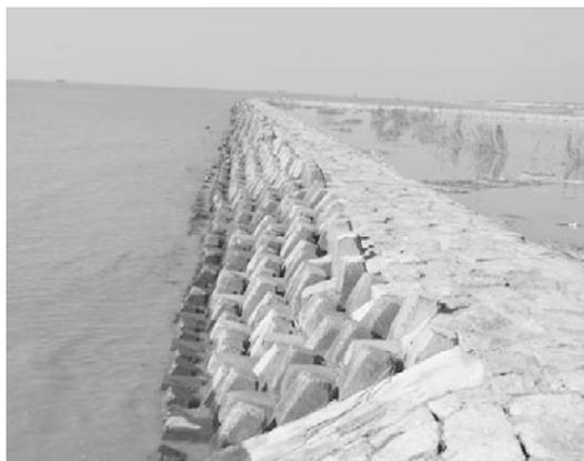
**Fig. 8.78** Spur dikes established for reclamation of wetlands in the Chongming Island, China
