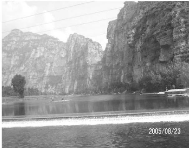
**Fig. 10.49** A weir placed on the Juma River in the suburbs of Beijing for creation and maintenance of a habitat with stable low current and high depth of water. In dry seasons the weir maintains a depth of water for fish and invertebrates to survive
