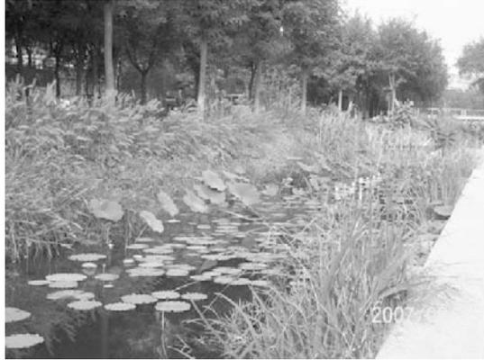
**Fig. 10.60** A layer of soil is placed on the hardened channel bed and banks on an urban stream in Beijing, and a vegetation bank and aquatic high plants have developed
