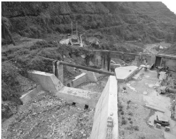
**Fig. 4.75** Three auxiliary dams downstream of a main dam on a debris flow gully in Ningnan County, Sichuan Province
