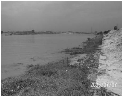
**Fig. 1.14** Channelization and hardened banks made the lower East River a straight river
