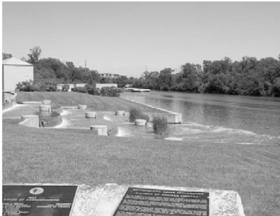
**Fig. 9.16** Sidestream Elevated Pool Aeration station number 5 discharging aerated water back to the Calumet-Sag Channel (See color figure at the end of this book)
