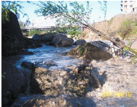
**Fig. 2.6** Channel erosion and collapse of vegetative banks and hardened banks on the Charlooze River in Iran, which was caused by floods
