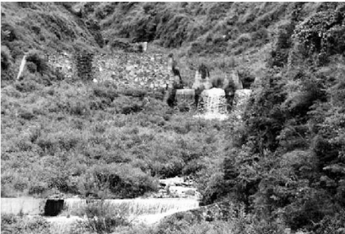
**Fig. 4.78** Debris flow control dams and reforestation of the hills used as the comprehensive debris flow control strategy in the Shengou drainage basin have changed the debris flow gully into a forest park of the Dongchuan City; Yunnan Province
