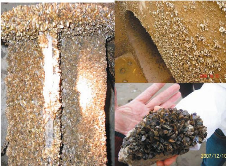
**Fig. 10.37** Colonization of golden mussel on concrete walls in a water transfer tunnel and attachment of golden mussel on a concrete fragment with high density
