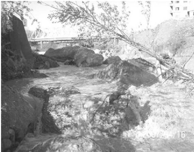
**Fig. 2.6** Channel erosion and collapse of vegetative banks and hardened banks on the Charlooze River in Iran, which was caused by floods (See color figure at the end of this book)
