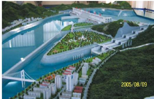
**Fig. 7.34** A model of the Three Gorges project on the Yangtze River- from right to left: five step ship locks including the upper and lower approach channels, the ship lift and its channel, the left power house, the spillway, and the right power house
