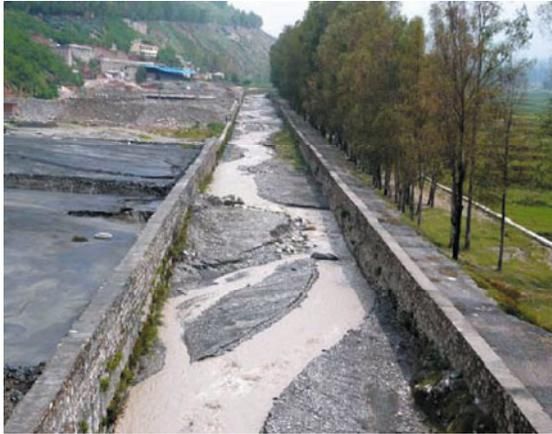
**Fig. 5.45** Regular meandering thalweg bed developed within a channelized stream in Yunnan, China
