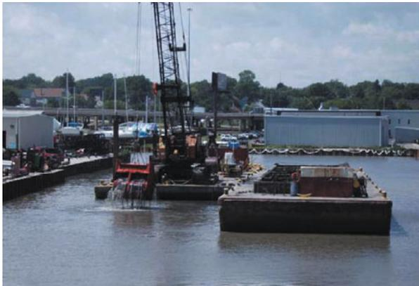
**Fig. 9.24** Environmental clamshell dredge removing PCB contaminated sediment from the Kinnickinnic River Great Lakes Legacy Act Cleanup in Milwaukee, U.S. and preparing to place it in a collection barge (photo provided by Dr. Xiaochun Zhang, Wisconsin Department of Natural Resources)
