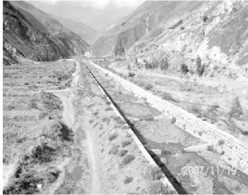
Fig. 4.72 Debris flow-guiding channels on a debris flow gully in the Xiaojiang River basin
