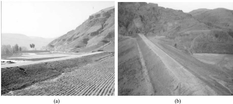
**Fig. 6.15** (a) A sediment check dam in the Sha-anxi Province has trapped sediment and created fertile farmland; (b) A new sediment check dam in Shanxi Province has been completed and begun to trap sediment (See color figure at the end of this book)
