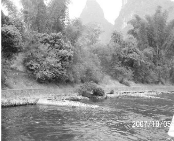
**Fig. 10.48** Spur dikes on the Lijiang River in south China used to promote the formation of low velocity habitats
