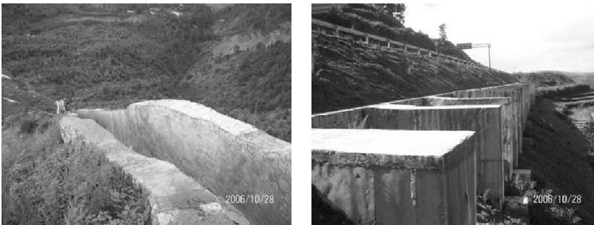
**Fig. 4.65** (a) A drainage system on a landslide body in the upper Yangtze River basin installed to lower the groundwater table; and (b) Concrete walls installed to stabilize a sliding body
