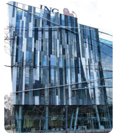
Stick glazing system: ING Headquarters, Budapest, Hungary. Architect: Erick van Egeraat
