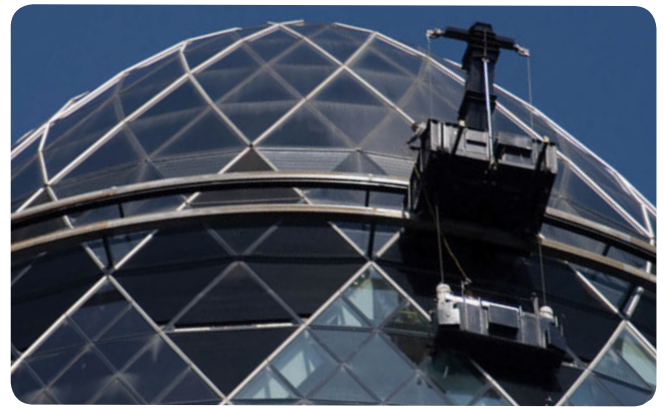
(Above). Cleaning cradle on trolley around Swiss Re building, London, U.K. Architect: Foster and Partners
