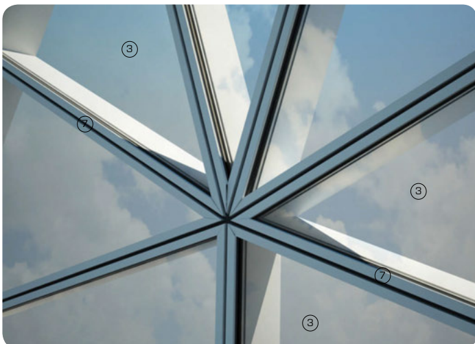
3D detail views showing triangular unitised glazing panels for twisted facade
