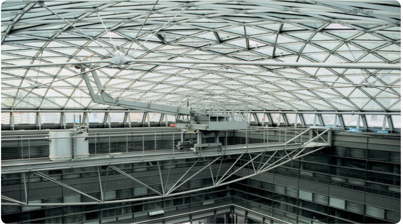
Cleaning gantry allowing underside of roof to be cleaned and maintained without cleaning platform from below. B8 offices, Daimler Chrysler Projekt, Potsdamer Platz, Berlin, Germany. Architect: Richard Rogers Partnership.
