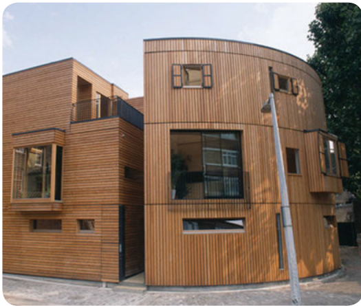
Timber cladding panels: Carmarthen Place, London, U.K. Architect: Architects in Residence
