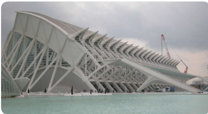
Curved concrete frame. Science Park, Valencia, Spain. Architect: Calatrava
