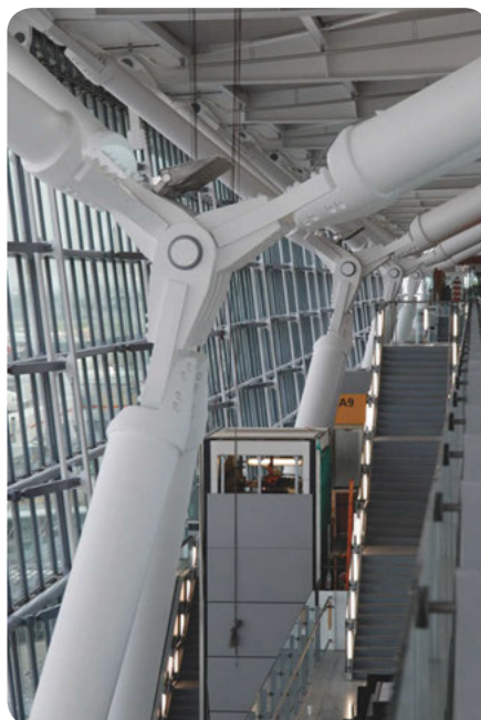
Branched steel roof structure. Heathrow Terminal 5, London, U.K. Architect: Rogers Stirk Harbour
