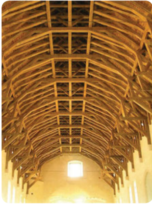
Hammerbeam Roof, Stirling Palace, Scotland, U.K.
