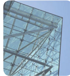
Stick glazing system: ING Headquarters, Budapest, Hungary. Architect: Erick van Egeraat
