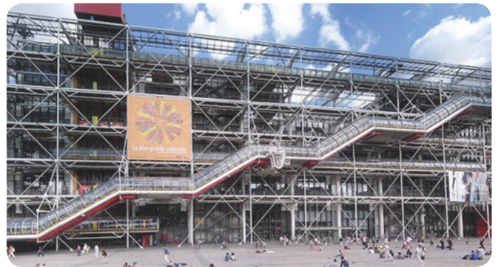
Braced steel frame. Pompidou Centre, Paris, France. Architect: Richard Rogers
