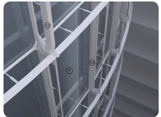
3D internal views showing cast aluminium glazing frames with double-layer rod support
