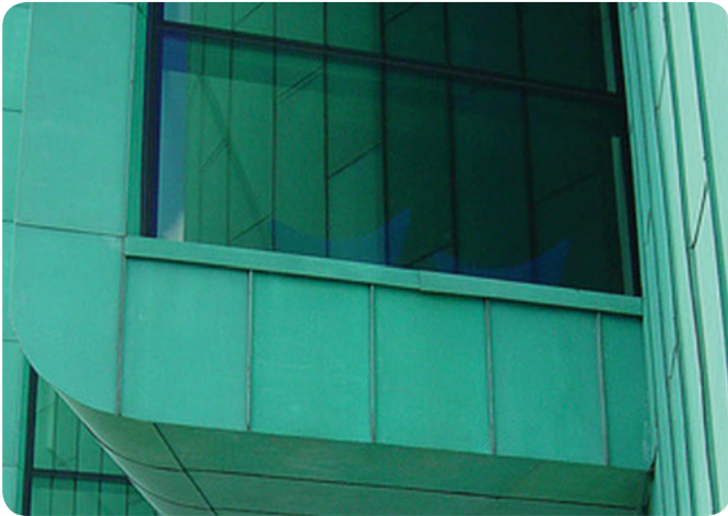
Copper cladding in use
