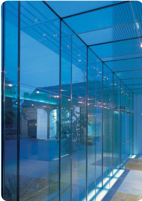
Loadbearing glass box. Broadfield Glass Museum, West Midlands, U.K. Architect: Design Antenna
