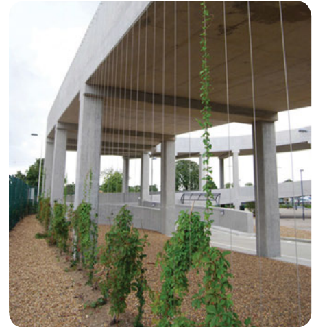
Tensioned wire green wall, Heathrow Airport, U.K.
