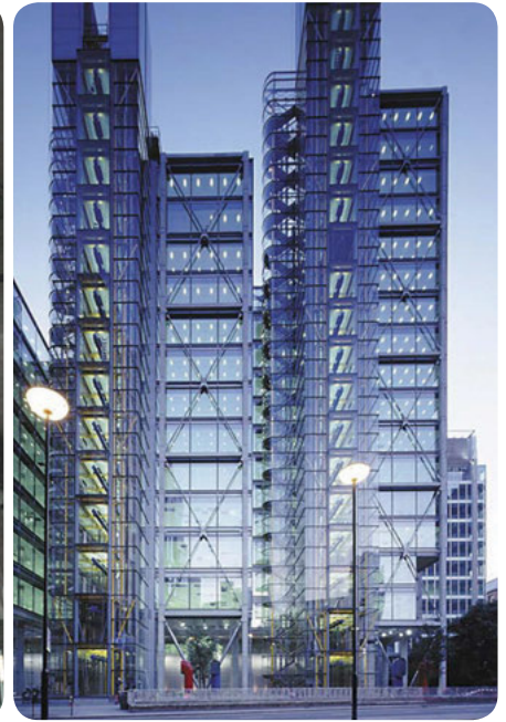
Braced steel framed construction. Wood Street, London, U.K. Architect: Richard Rogers
