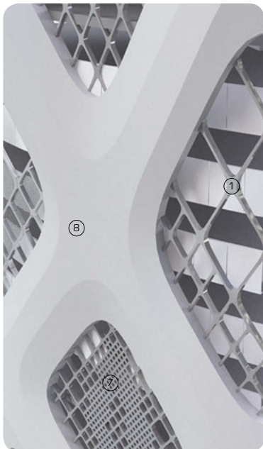
3D view showing GRC-clad steel exoskeleton with metal mesh panel infill
