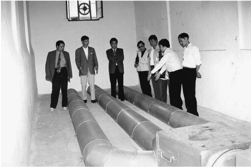
FIGURE 10.6 Warehouse with on-floor ductings for in-store drying.
