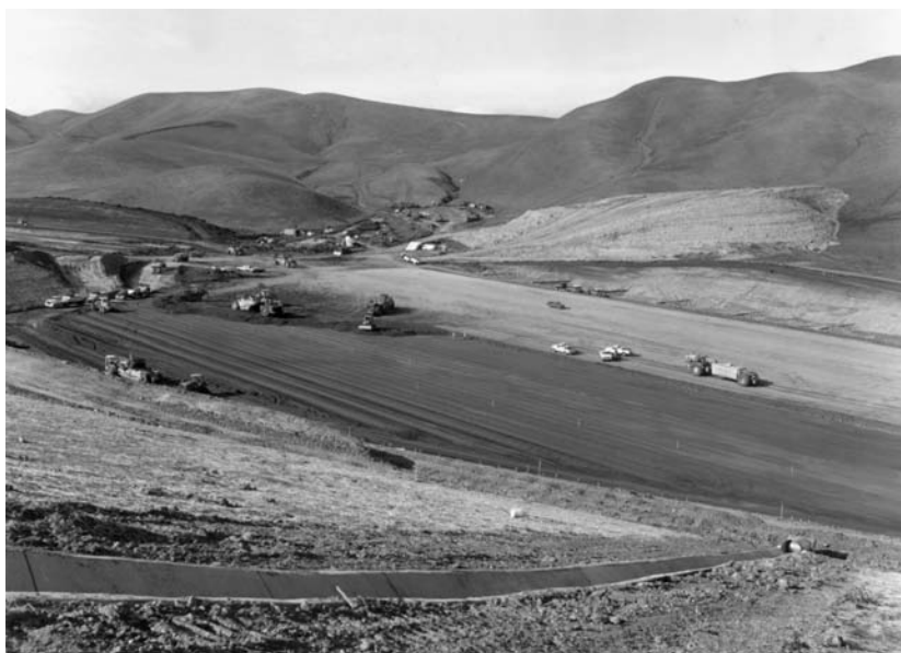
FIGURE 3.25 Development of large ravine landfill site. Equipment is compacting sub-base of landfill in preparation for placement of geomembrane liner.
