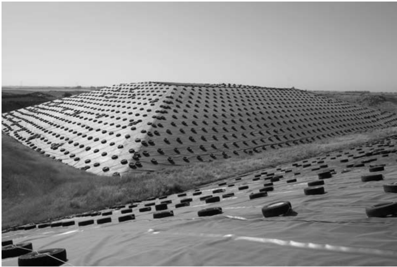
FIGURE 3.30 Bioreactor type landfill with leachate recirculation: (a) schematic diagram and (b) photograph of a highly instrumented anaerobic landfill bioreactor located at Davis, California. Photo of bioreactor was taken shortly after landfill was completed, before significant decomposition had occurred. (Source: O’Leary, P. R., and G. Tchobanoglous, “Landfilling,” in G. Tchobanoglous and F. Kreith (Eds.), Solid Waste Handbook , 2nd ed., McGraw-Hill, New York, 2002, Chapter 14.)
