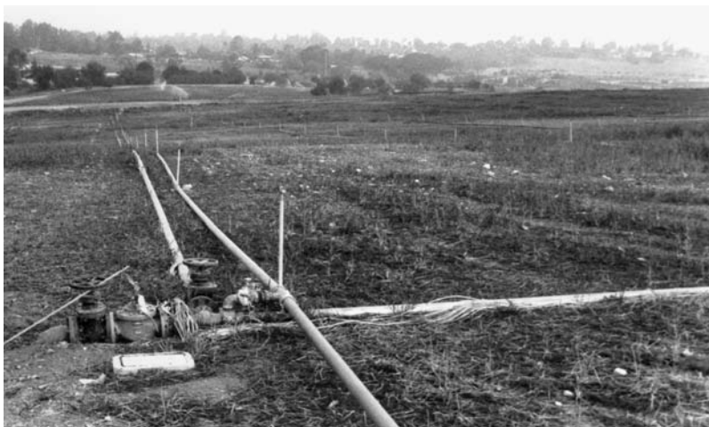
FIGURE 3.38 Completed landfill with irrigation system.
