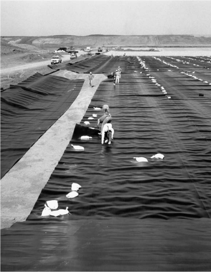
FIGURE 3.28 Placement of geomembrane liner in area-type landfill.
