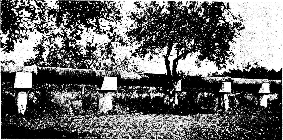
Figure 16-17 Sewer supported on piers.
