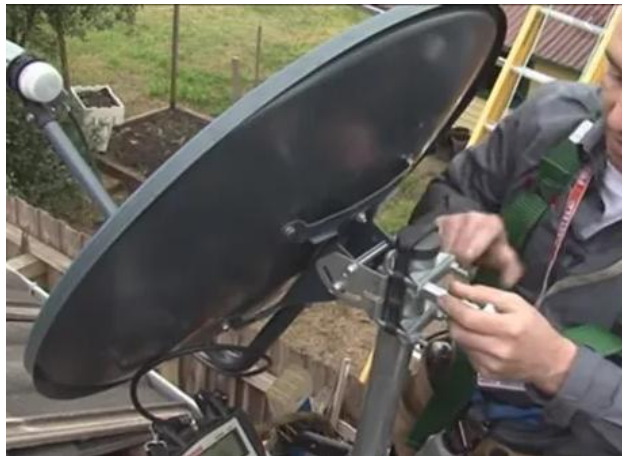
Fig. Tightening loosely connected bolts and nuts
