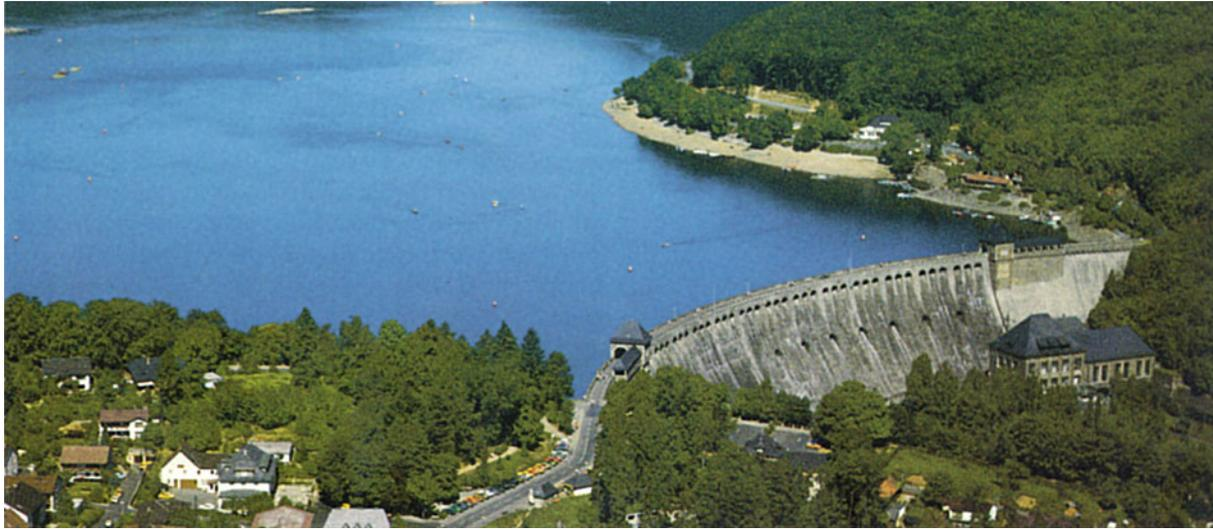
**Figure 6.26** River dam of the river Eder, Germany. The bending of the dam towards the water side conducts part of the water pressure against the mountain sides (see Sect. 6.3). With kind permission of Cramers Kunstverlag, Dortmund
