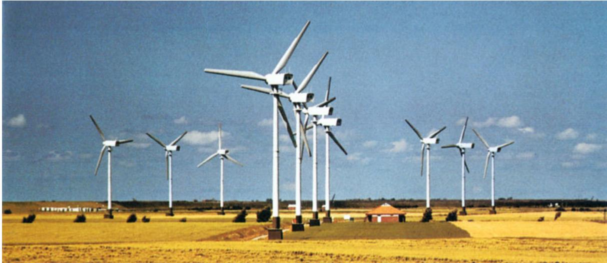
**Figure 8.49** Windfarm Krummhörn. Rotor span width is 30 m, the nominal electric power output is 300 kW per wind converter. (With kind permission of EWE corporation, Oldenbourg)
