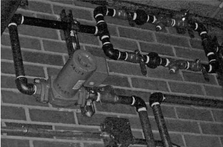
**Figure 3.5** Pipes and an in-line pump mounted on brackets
