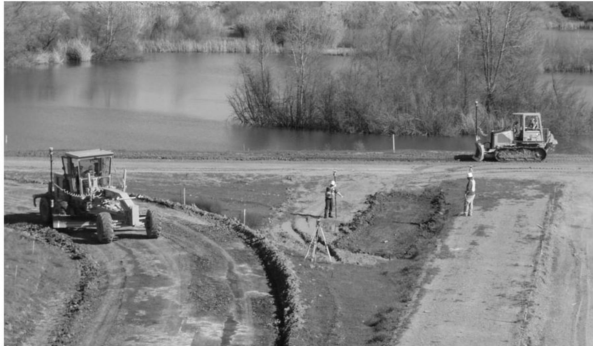
A dozer and grader using machine control to create an intersection of roads.
