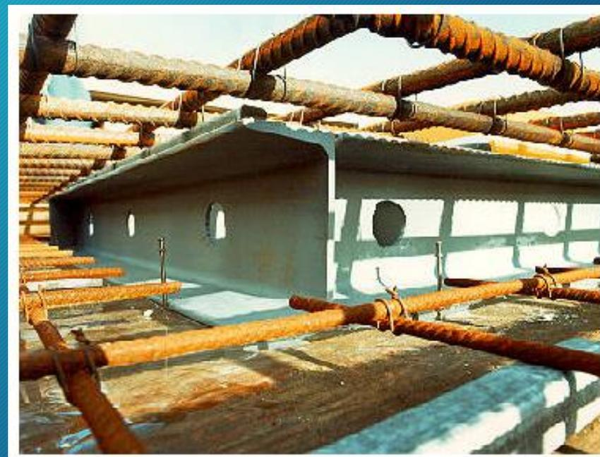
The detail is much simpler than traditional links, making it far easier to fix. The **shear resistance** of a shear head is either determined by test, or provided by the manufacturer.
