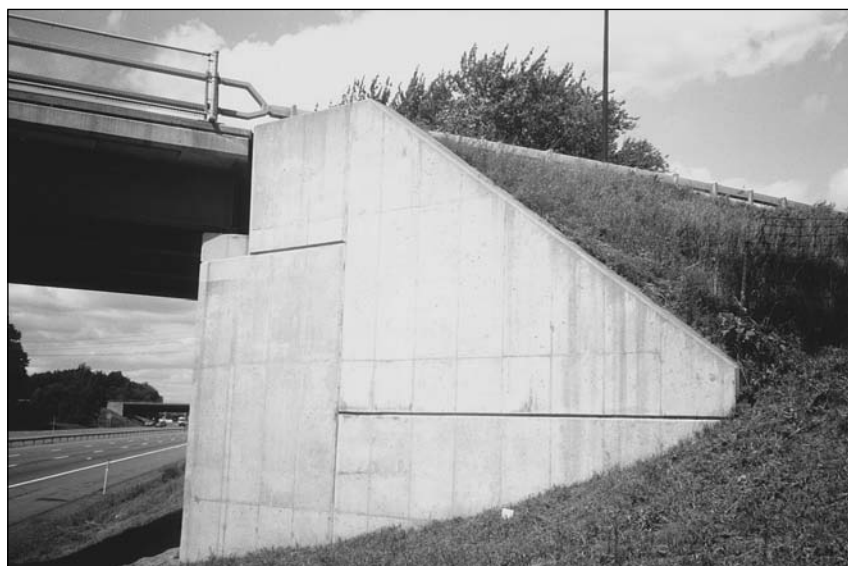
Figure 1.6 Wingwall of a two-span bridge crossing the Interstate.
