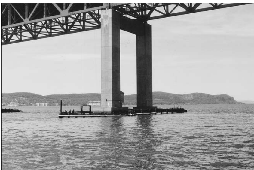
Figure 4.12 A two column bent pier helps support the Tappan Zee bridge.
