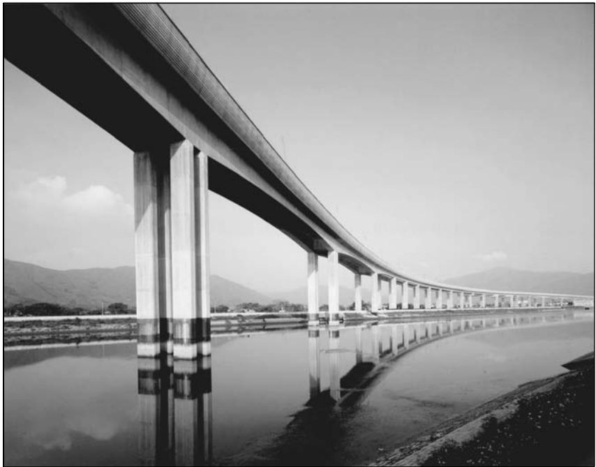
Figure 1.11 KCRC West Rail Viaducts, Hong Kong.
