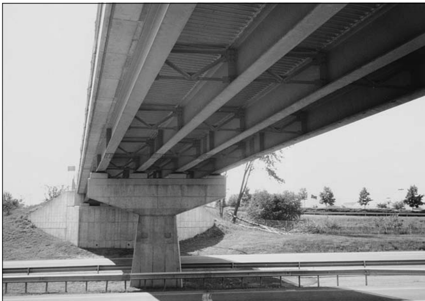
Figure 1.5 A hammerhead pier supports a slab-on-stringer superstructure.
