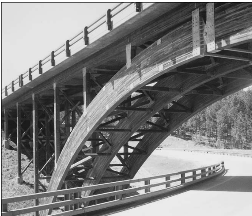
Figure 3.4 Timber was used to construct this open spandrel arch bridge in South Dakota.
