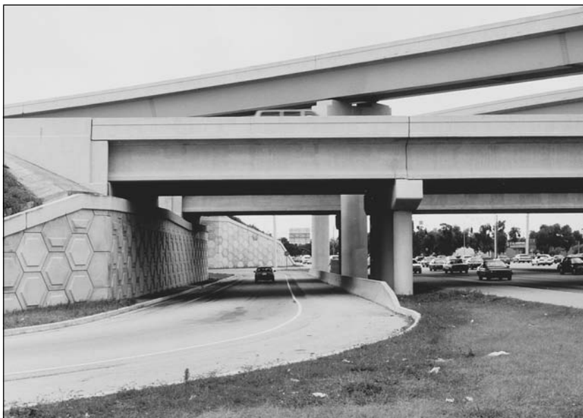
Figure 3.54 A steel plate girder structure passes over a prestressed concrete bridge in Florida. Steel and prestressed concrete often coexist in the same environment.
