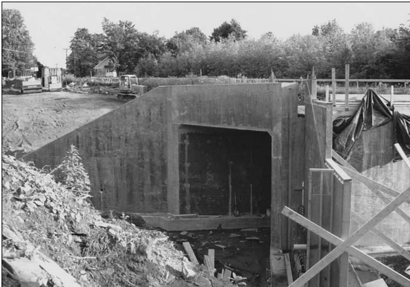
Figure 4.3 A single span bridge under construction crossing a stream.
