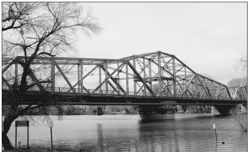
Figure 1.14 American River Bridge near Sacramento, California.
