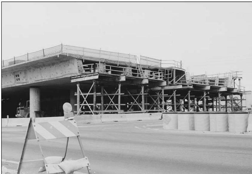
Figure 3.56 A prestressed concrete box structure under construction.
