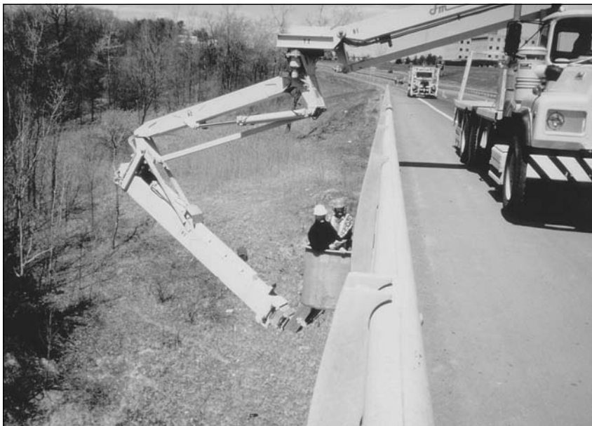
Figure 3.57 A bucket snoopers is used to inspect the underside of bridge over water.
