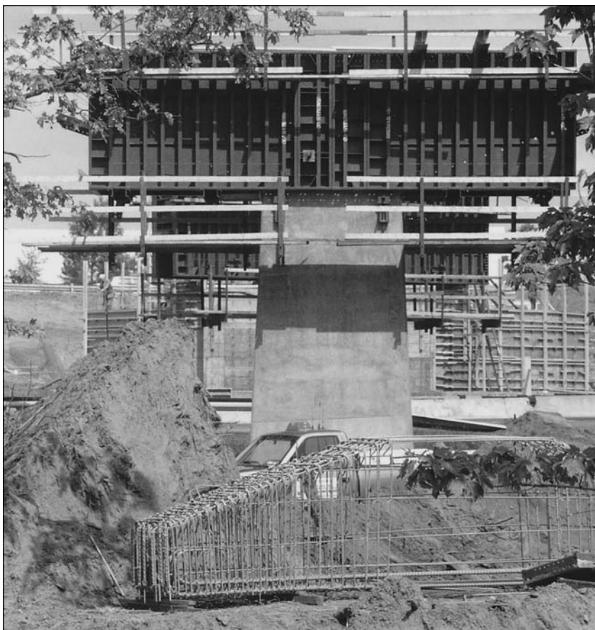
Figure 4.9 This hammerhead pier still has its cap beam formwork in place.
