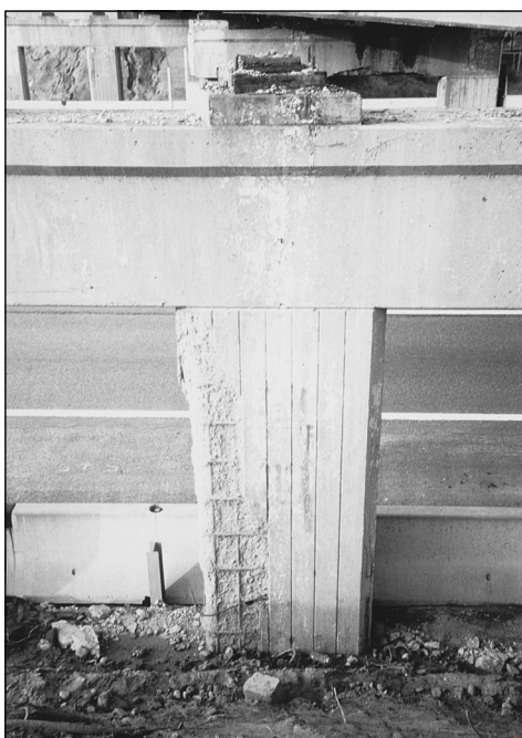
Figure 2.6 Exposed reinforcing signals repair.
