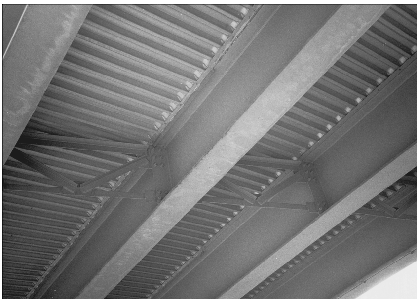
Figure 2.8 Stay-in-place forms can hide deterioration beneath them.
