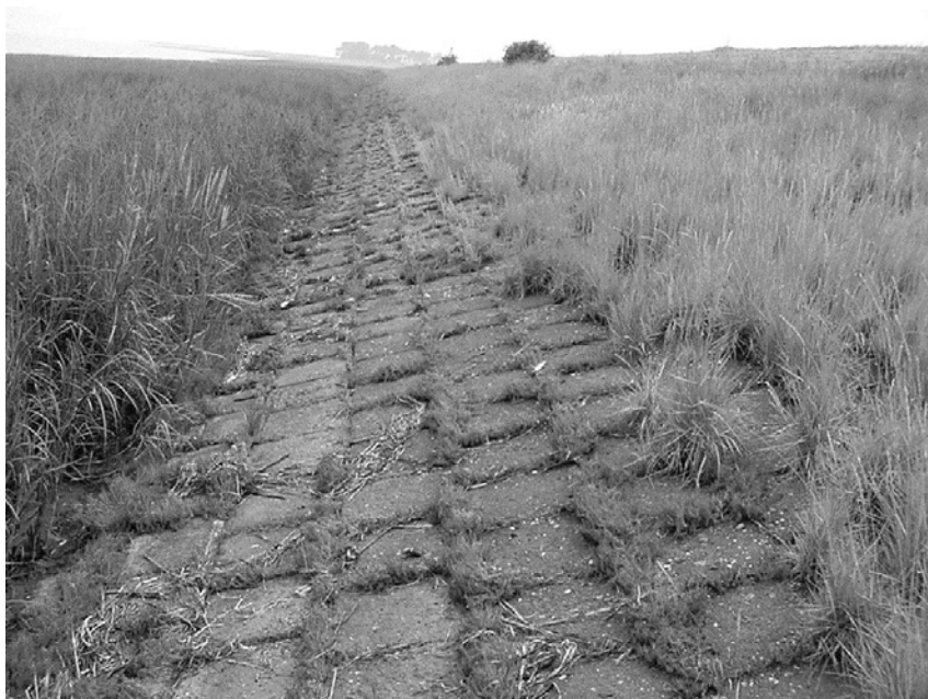
Figure 4. Reigersbergsche polder (Western Scheldt, near Rilland village): an interrupted vegetation gradient due to the used stone material.
