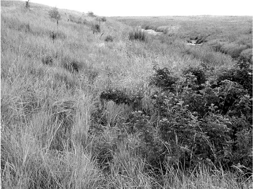
Figure 3. Hellegatpolder (Western Scheldt, near Kloosterzande village): a dike reach with a continuous vegetation gradient from the adjacent marsh to the top of the dike.
