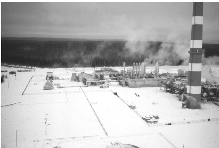
FIGURE 2.2 Natural gas processing plant. Petroleum refining and distribution facilities can impact groundwater through releases of hydrocarbons, produced water (brines), and other wastes and by-products. The petroleum industry is active in improving its environmental management through a number of organizations, such as IPIECA (International Petroleum Industry Environmental Conservation Association), the API (American Petroleum Institute), and CAPP (Canadian Association of Petroleum Producers).
