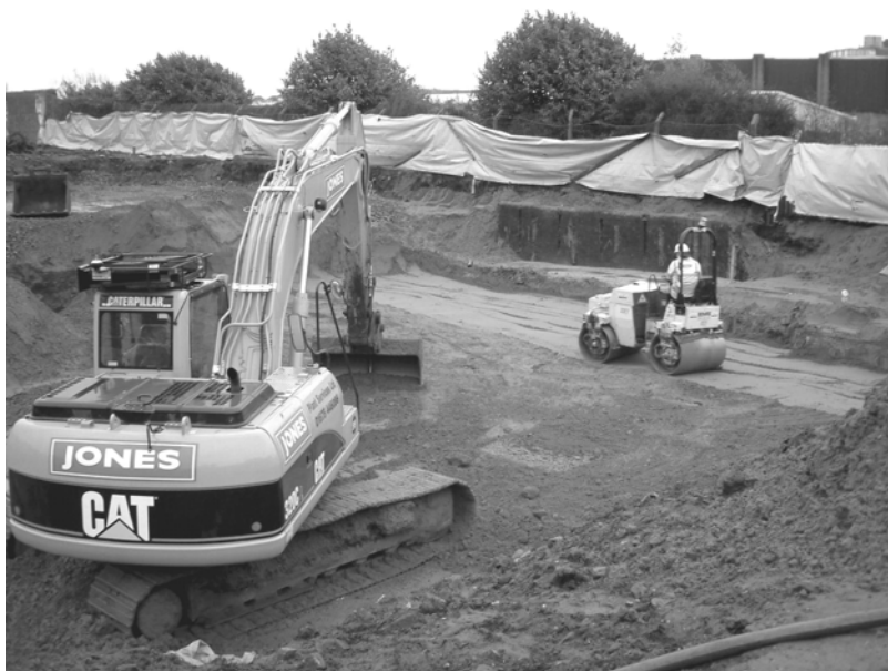
FIGURE 1.3 Excavation of contaminated soil as part of a major remediation project in the U.K.
