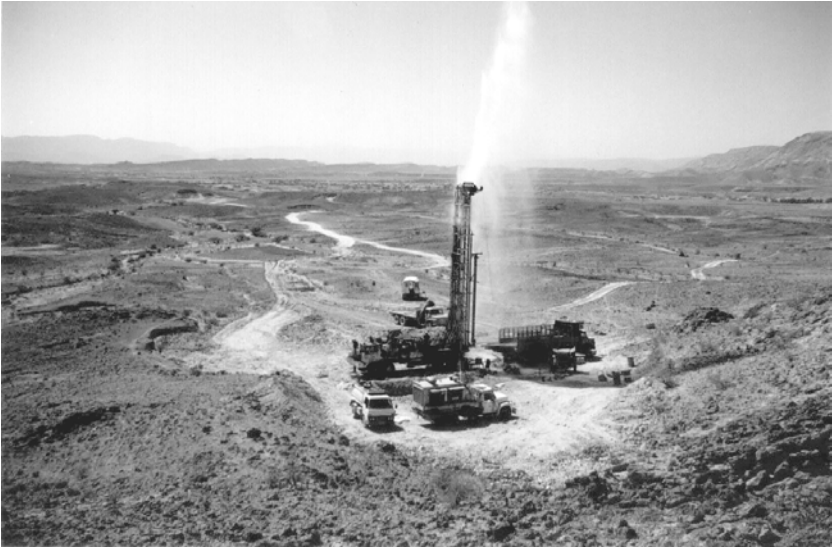
FIGURE 2.1A Drilling for deep groundwater in Yemen. (Photo courtesy of Komex.)
