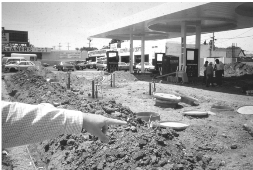
FIGURE 2.3 Petrol service station underground tank replacement.
