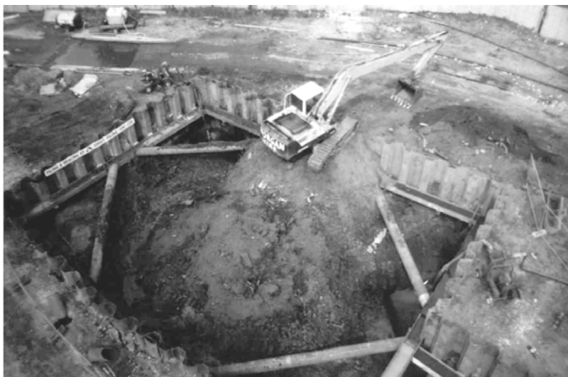
FIGURE 3.10 Removal of subsurface source of coal tar by excavation, as part of a remediation project at a manufactured gas plant in the United Kingdom. (Courtesy of Komex.)
