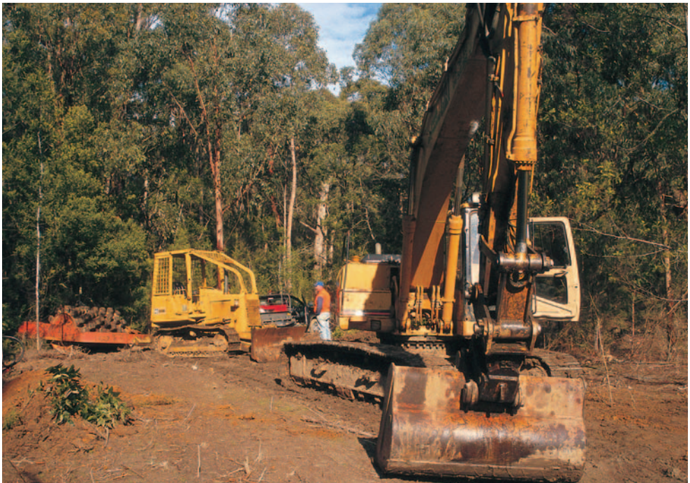
b) An excavator, and a bulldozer with a sheep's foot roller.
