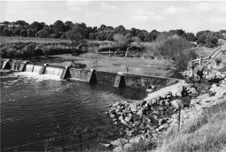
Photo 1.1 Typical in-stream barrier with rock-ramp fish way, Merri River, Victoria (Photo: T. O'Brien).
