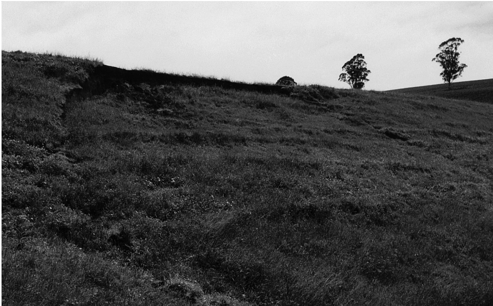
Photo 6.3 Slump on the downstream batter slope.
