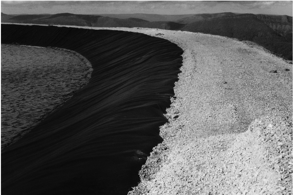
Photo 6.4 Plastic liner on the upstream side of the dam crest.
